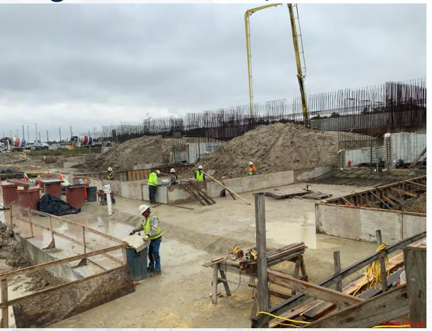
281-FILTER MODULE- Reinforcing/Forming/Pouring Walls
