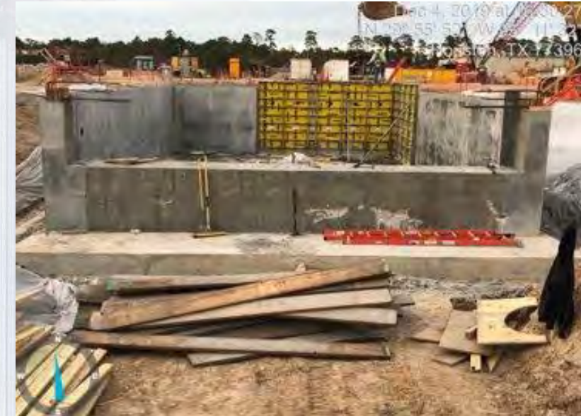
Removing formwork at the Overflow box
