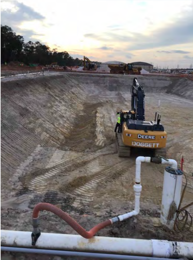
Installed dewatering wells at facility 401
