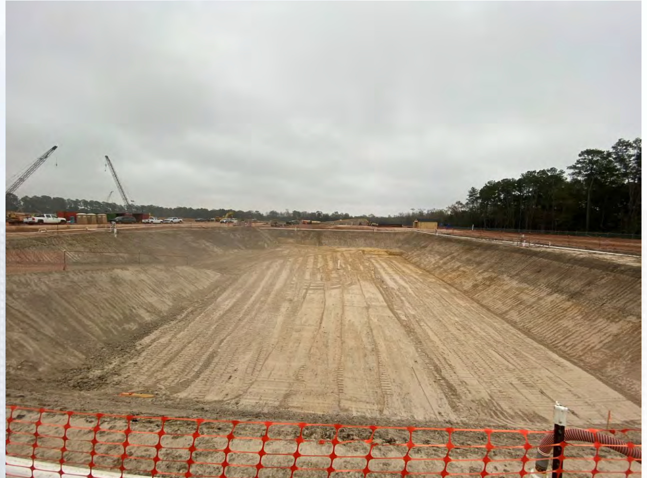
Facility 401 Mass Excavation down to groundwater elevation
