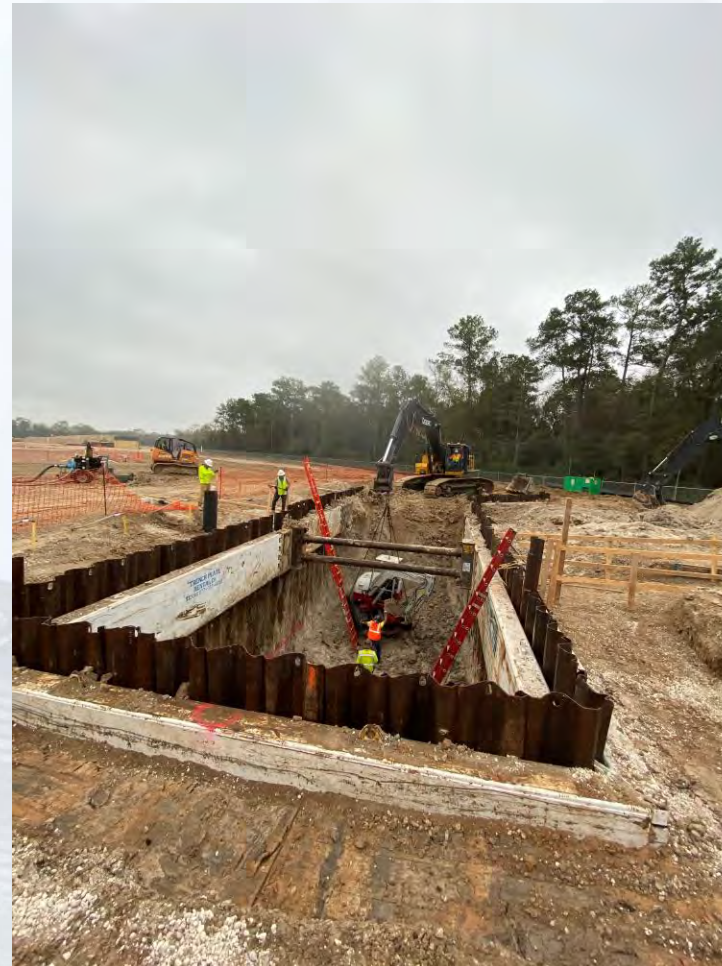
Installing Sheet piles for the 102" pipe at GST 362
