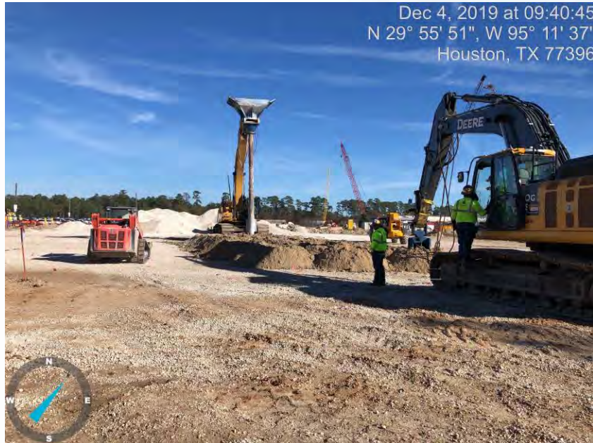
Installing Vibro Stone Columns (VSC's) at GST 361
