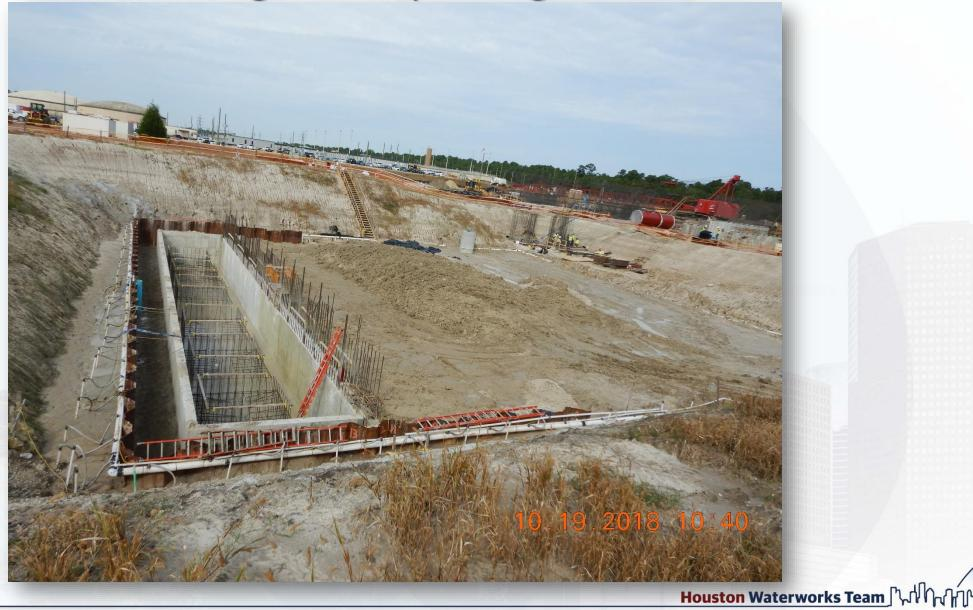
**Backfilling & Compacting Behind TPS Retaining Wall**
