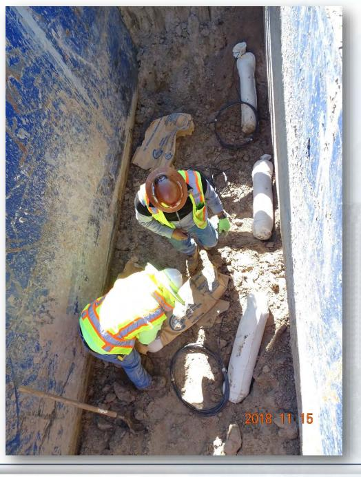
Installing anodes and Cathodic Protection on 24in FW Pipeline
