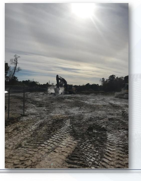
Lime Stabilizing subgrade
