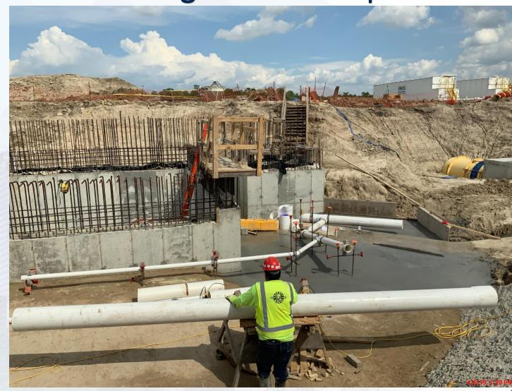
FILTER STRUCTURE- Excavation (FD Pump Can) & Backfill (b/w TPS & Filter)
