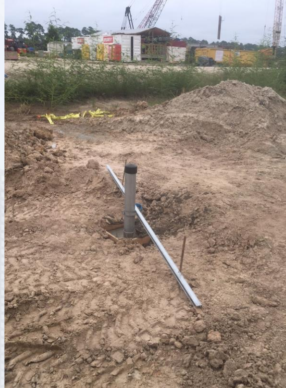
T362 Temp Power Bore
