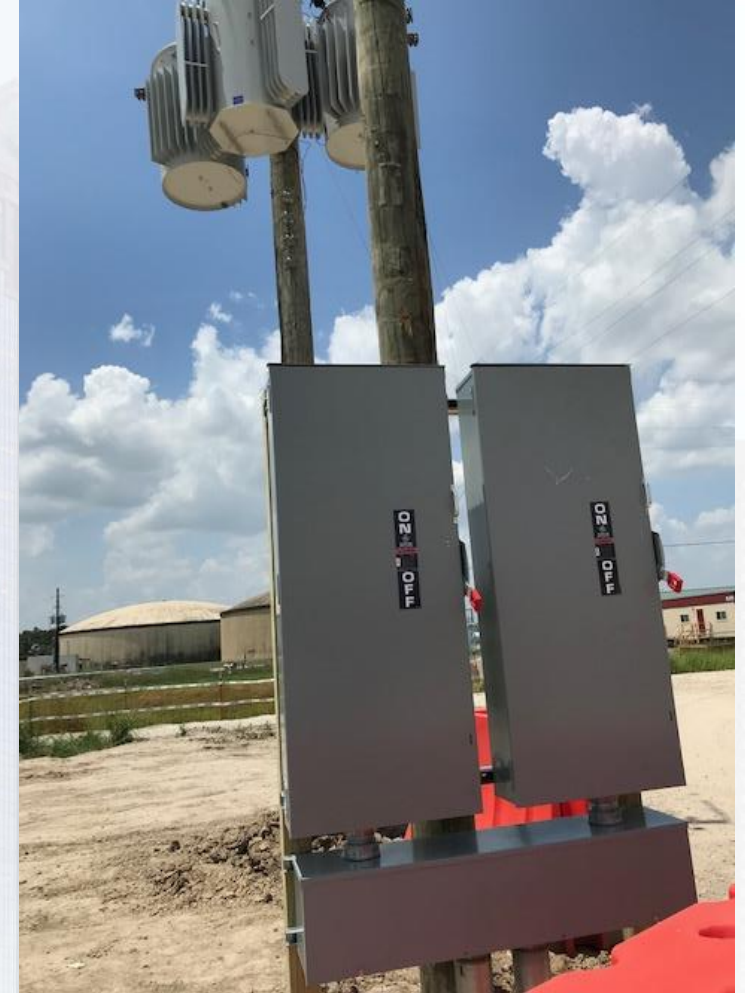
(New) H13 Power South Plant, HSPS, T-291,T-312 1,200 Amp Service
