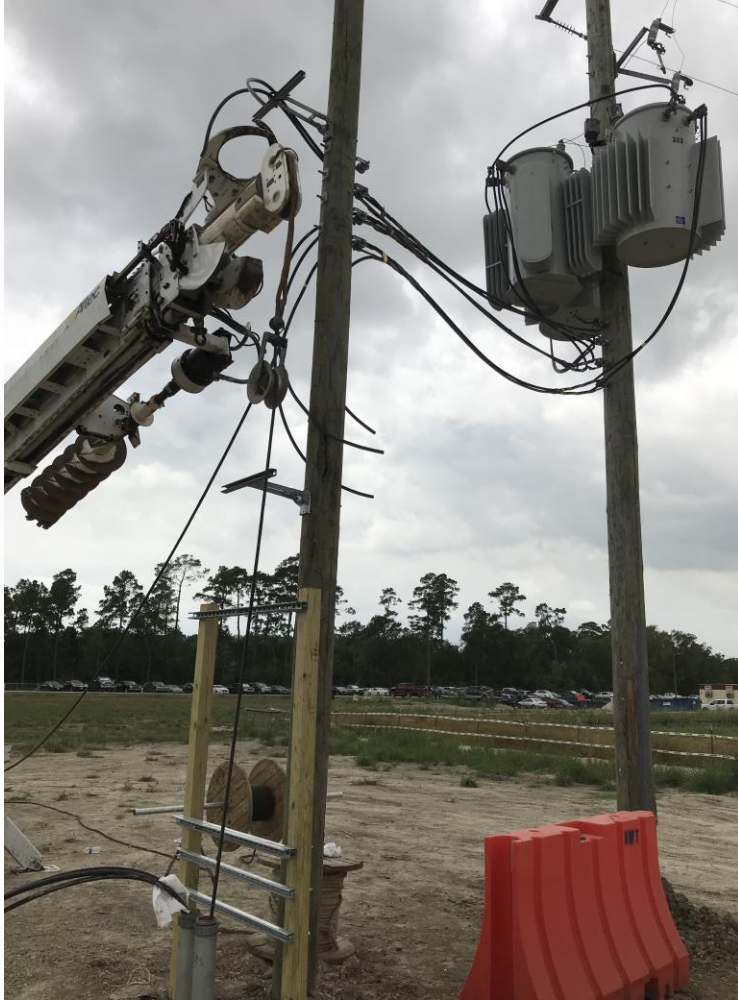
Wire Pull to South Plant Temp Power
