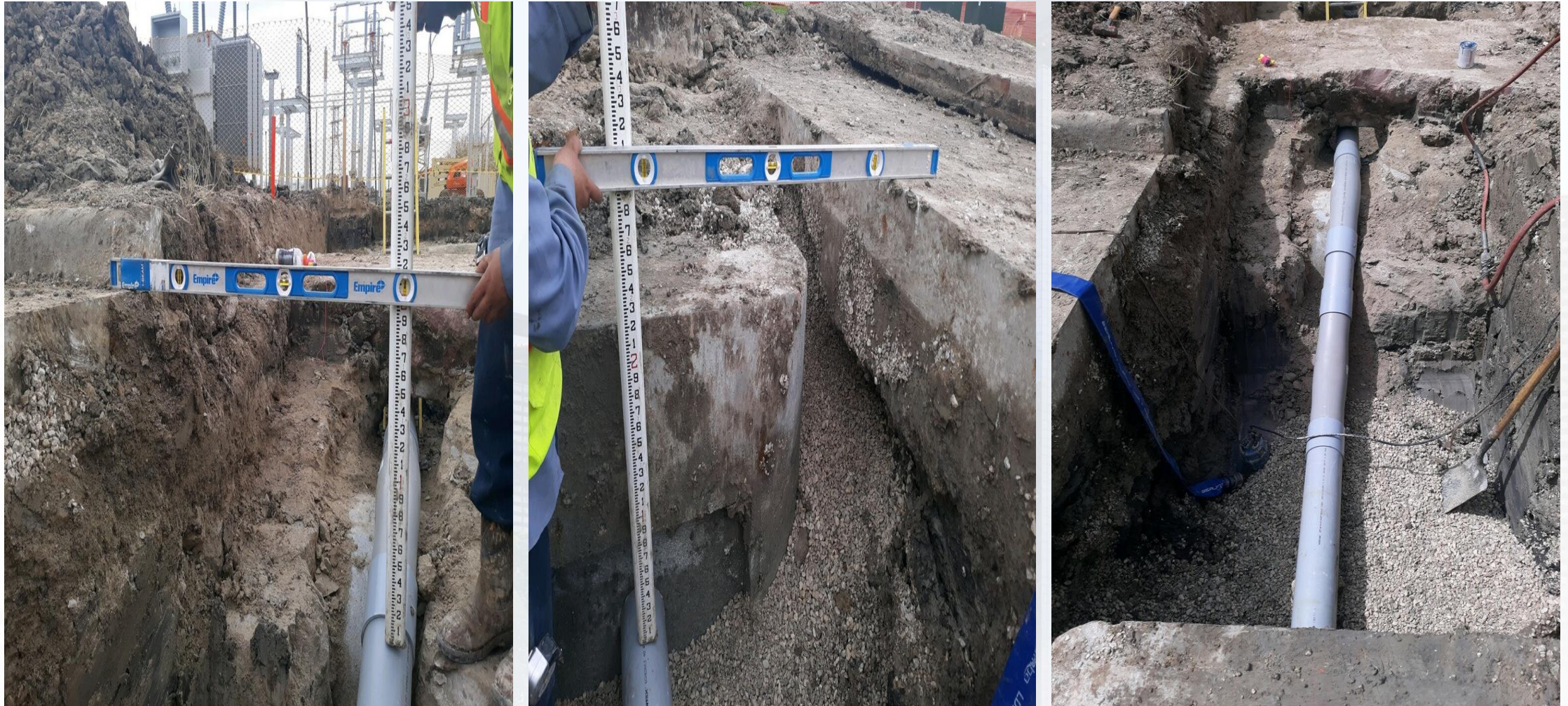
Found the depth and mocked up the run into the 102
