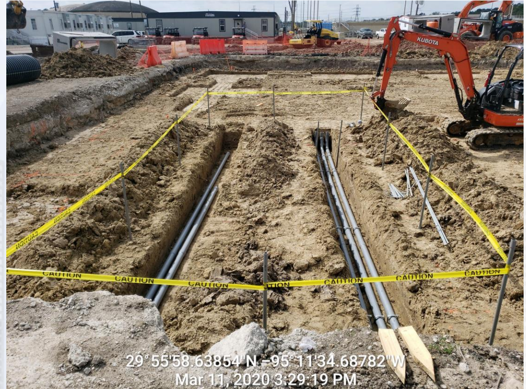
Installation of Electrical Conduit in the MB
