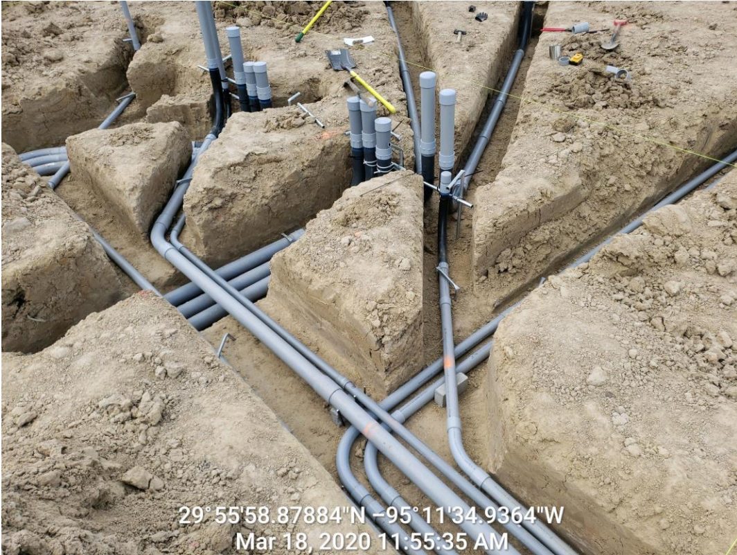
Installation of Electrical Conduit in the MB
