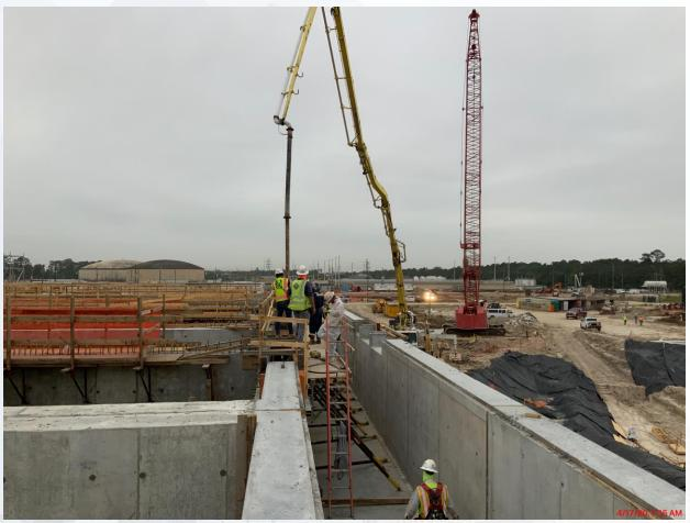
281-FILTER MODULE- Reinforcing/Pouring Filter 2 Slab
