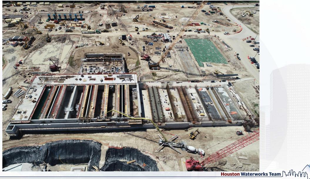
282- Reinforcing/Pouring OZW Inlet Box(West) Walls
