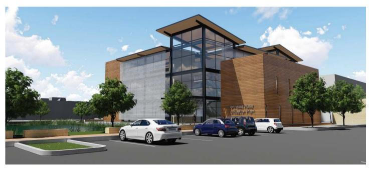
The major component of the expansion is a new treatment facility; constructed on land owned by the City of Houston next to the current plant. It is designed to supply 320 million gallons per day of treated water capacity in addition to the current 80 million gallons per day of treated water capacity.
