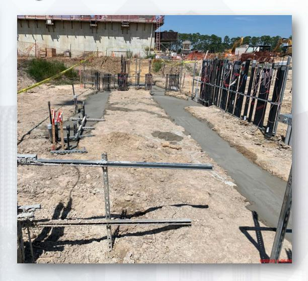
282- FILTER MODULE 2- Reinforcing/Pouring First Foundation Slab
