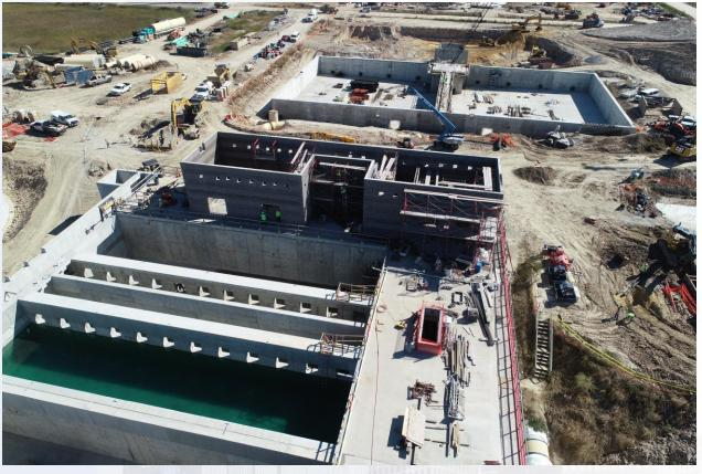
281-FILTER MODULE - Setting Scaffolding for West Side Masonry
