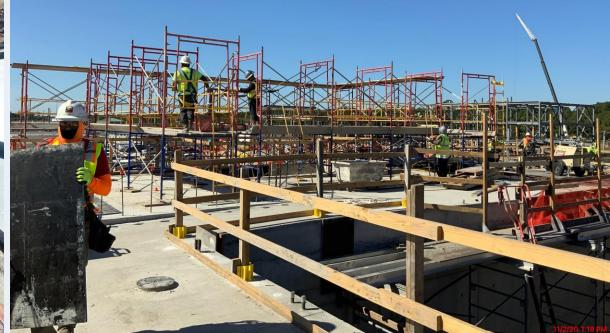
281-FILTER MODULE- Reinforcing/Pouring Walkways
