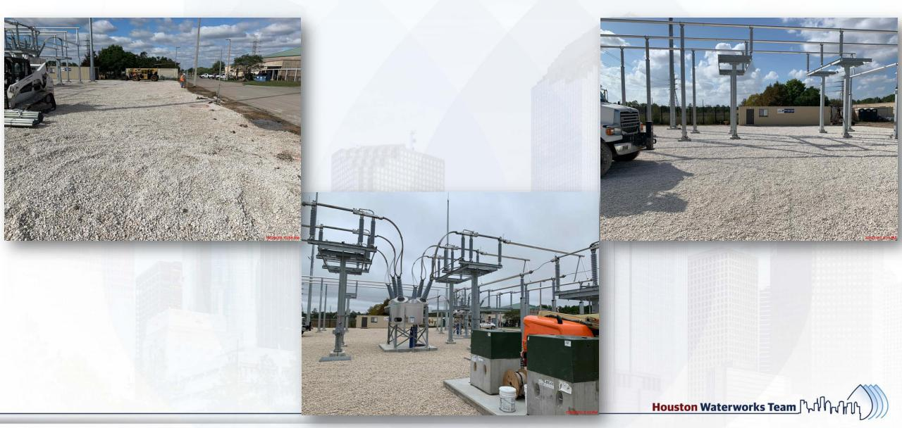
Installation of lighting fixtures, DC battery system and prelim-testing of 25kV switchgear
