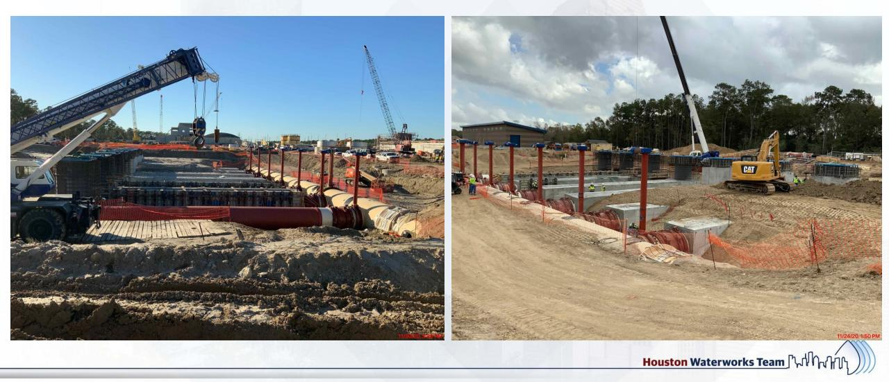
Rebar installation at locking slabs, installation of grout and leveling pump cans at HSPS 402
