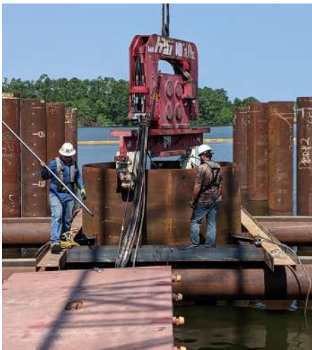
Preparing To Drive 10' Pump Can Casings at Intake Pump Station
