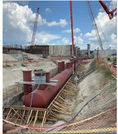
Filter Module- CFE/FTW Pipeline Encasement
