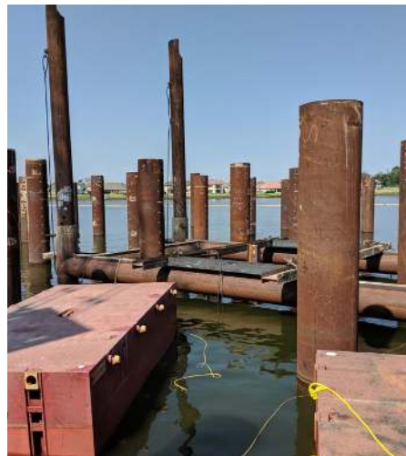
Preparing To Drive 10' Pump Can Casings at Intake Pump Station
