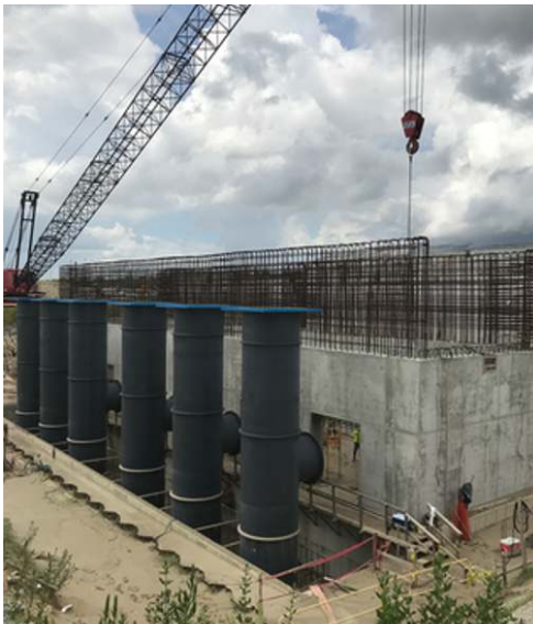
TPS – Installing Pump Cans
