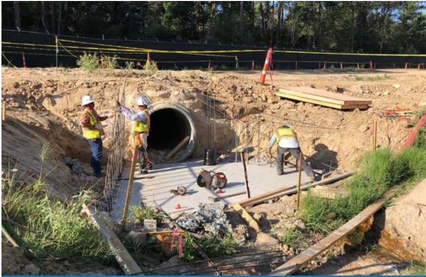
Storm Drainage Installation in West Corridor
