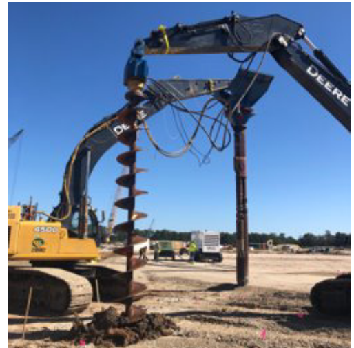
GST Vibro-stone column installation
