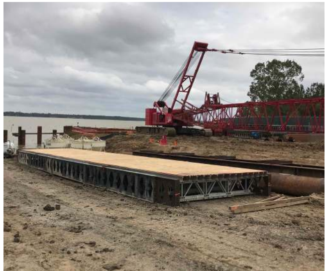
IPS platform construction
