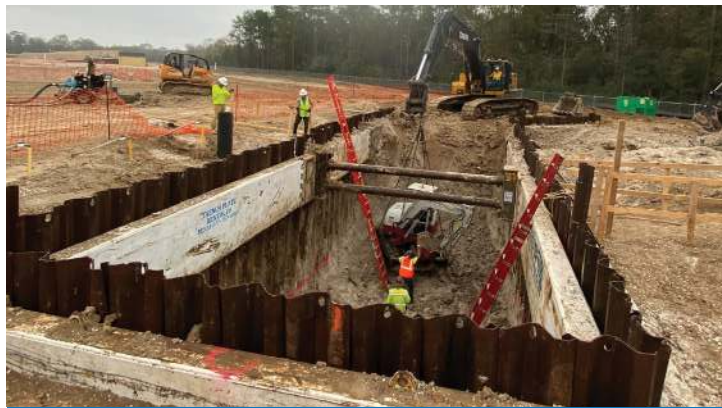
Gst 362 Trench Prep for 102" FW Pipe
