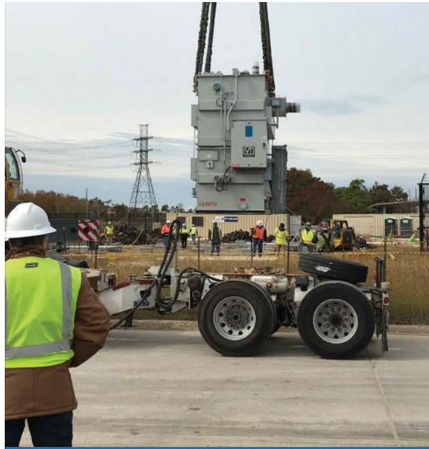
Facility 102 Transformer Installation
