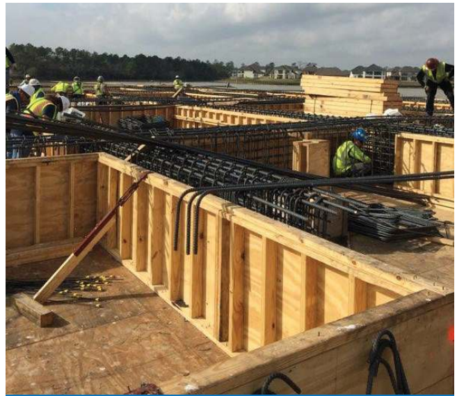
IPS Deck Formwork
