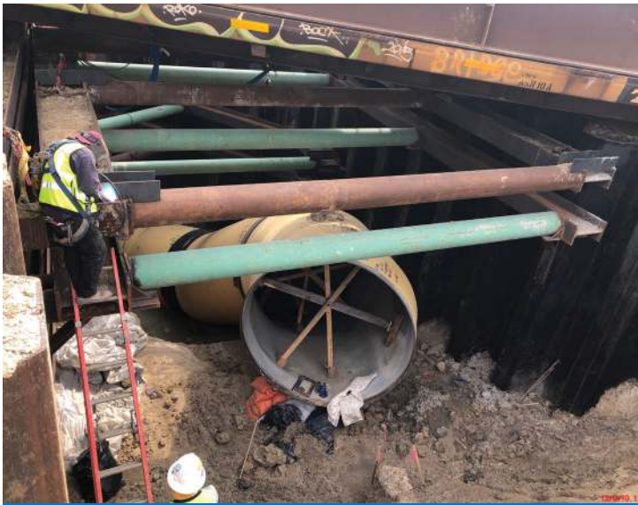
Sta 128+50 Pipe Installation
