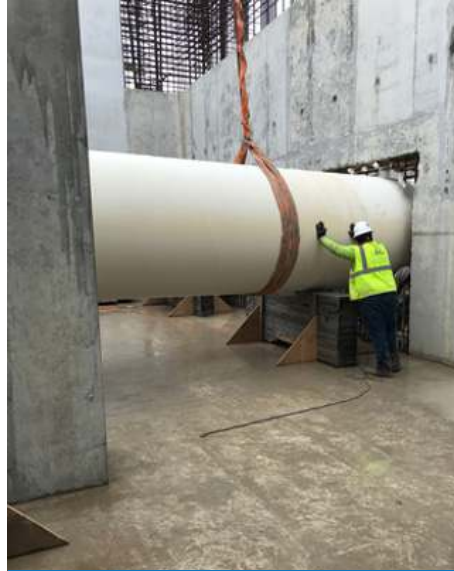
TPS – Installed 60” Suction pipes (East Half)
