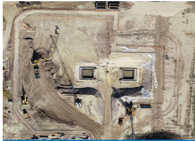
Facility 601/602 Excavation Progress
