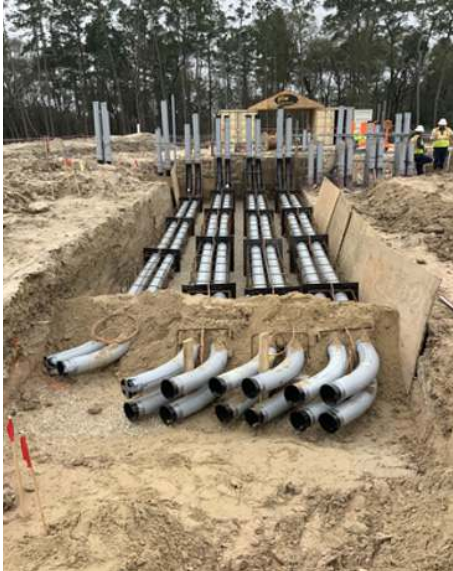
Under Slab Conduit Placement at Facility 111
