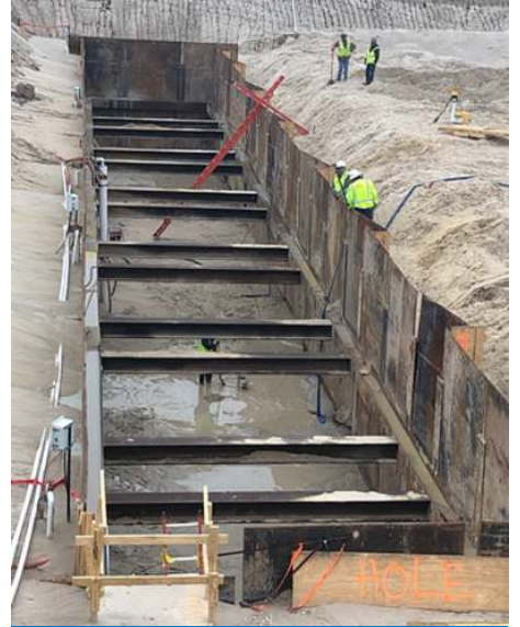
Excavation and dewatering for HSPS 401 pump cans
