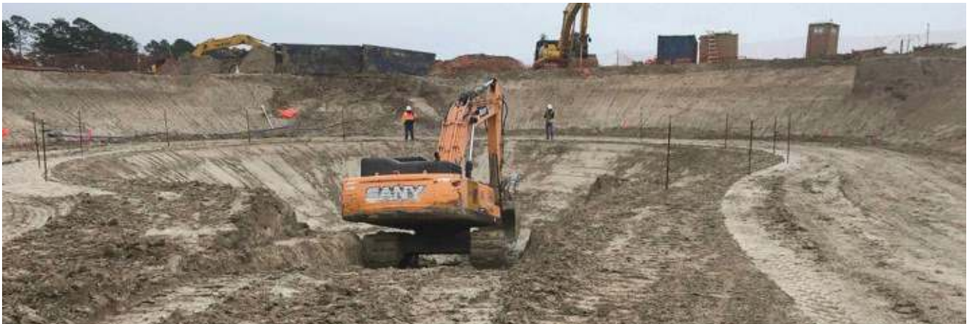
Facility 502 Mass Excavation
