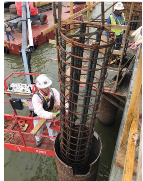
Preparing Bridge Piles for Precast Bridge at IPS
