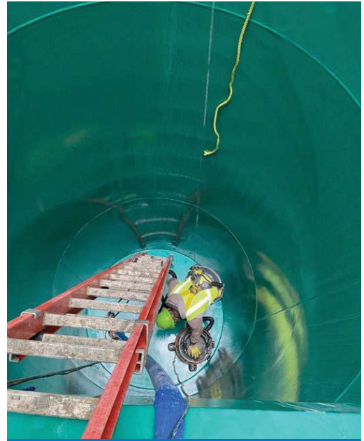
Cleaning Pump Cans at TPS
