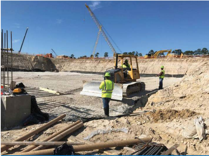
Limestone Rock Placement for 601 Underdrain
