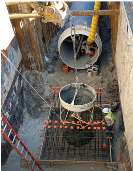
84-inch pipe installation in Corridor 4
