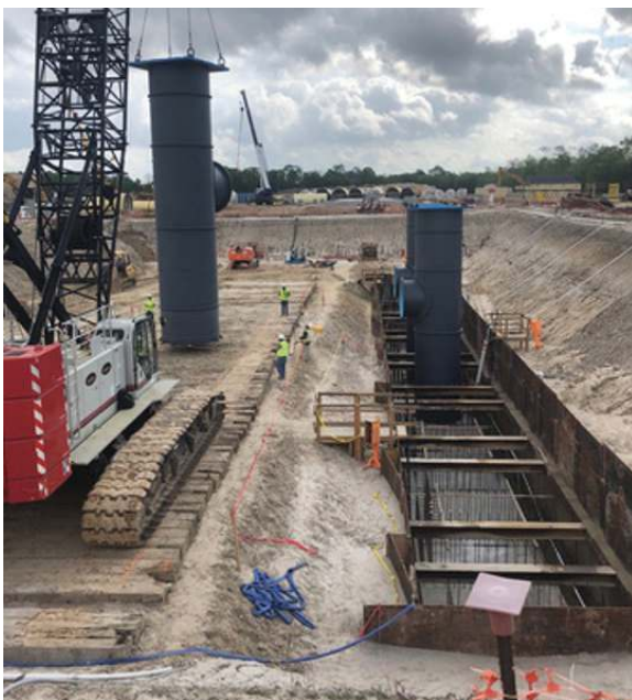
Pump can placement at HSPS 401
