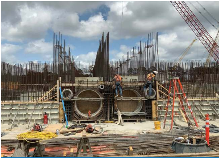
281 - Filter Module - Reinforcing/Forming/Pouring Walls
