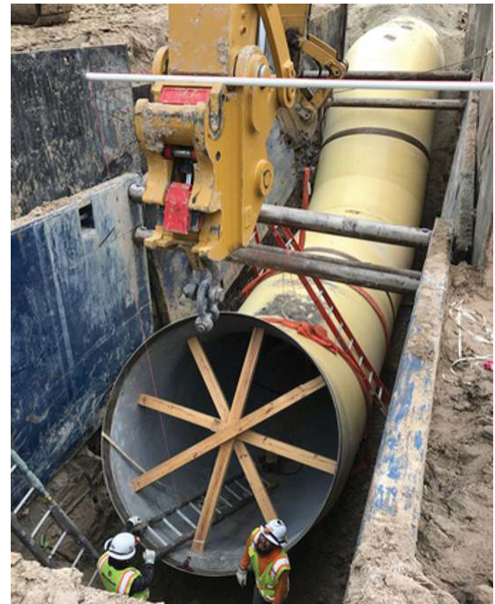
Installing 108" RW steel pipe line in Corridor 1
