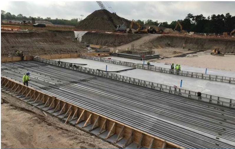
Rebar Installation North Area of 601
