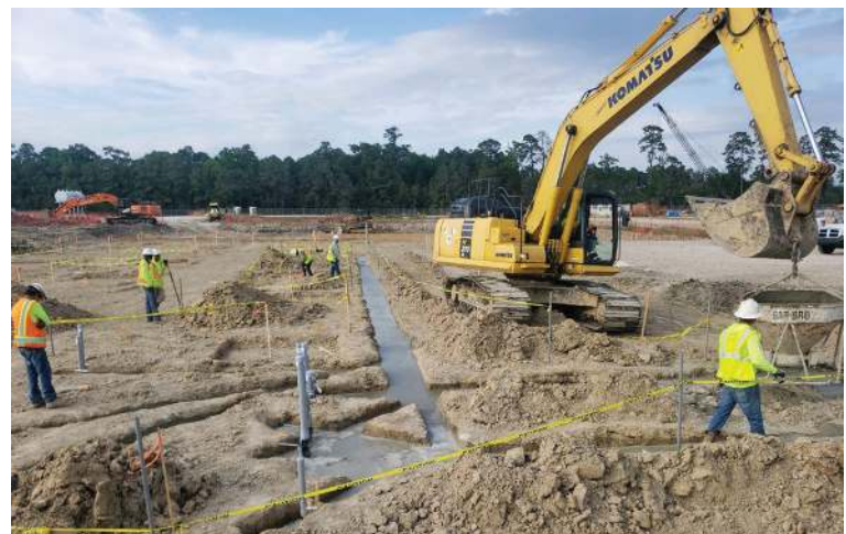
Installed Electrical Conduit in the MB
