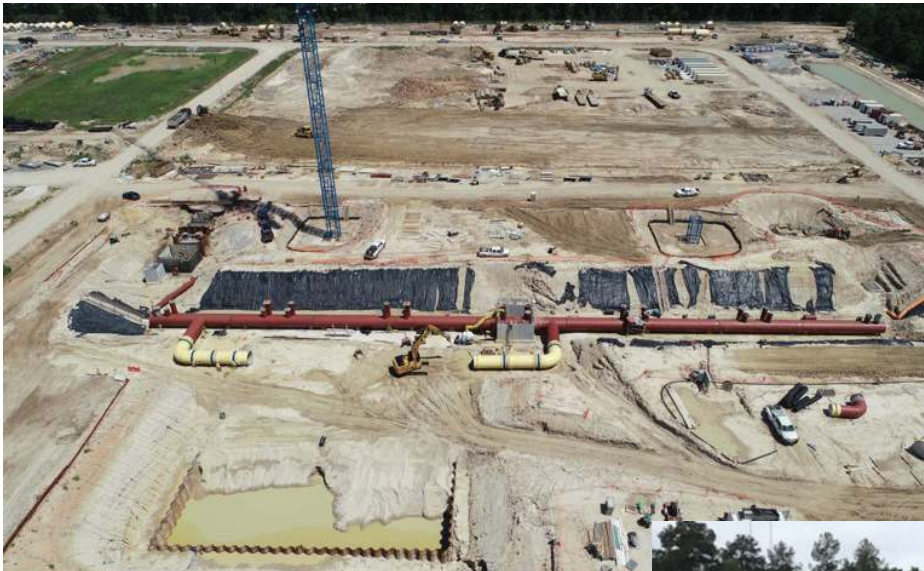
Central Plant – 2nd Phase
