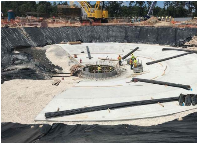
Facility 502 Basin #4 Mud Matt and Rebar Placement
