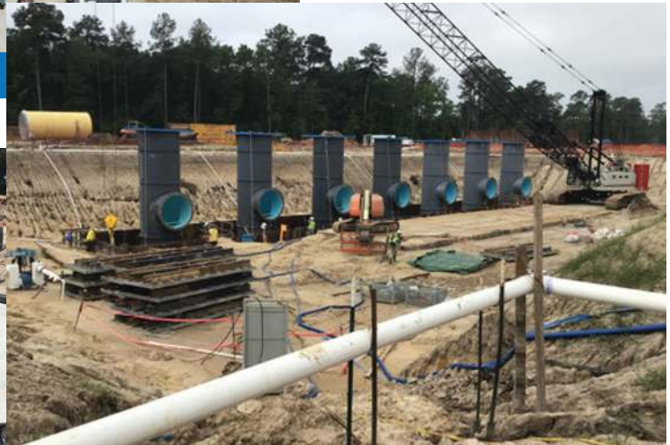
Pump Installation at HSPS 401
