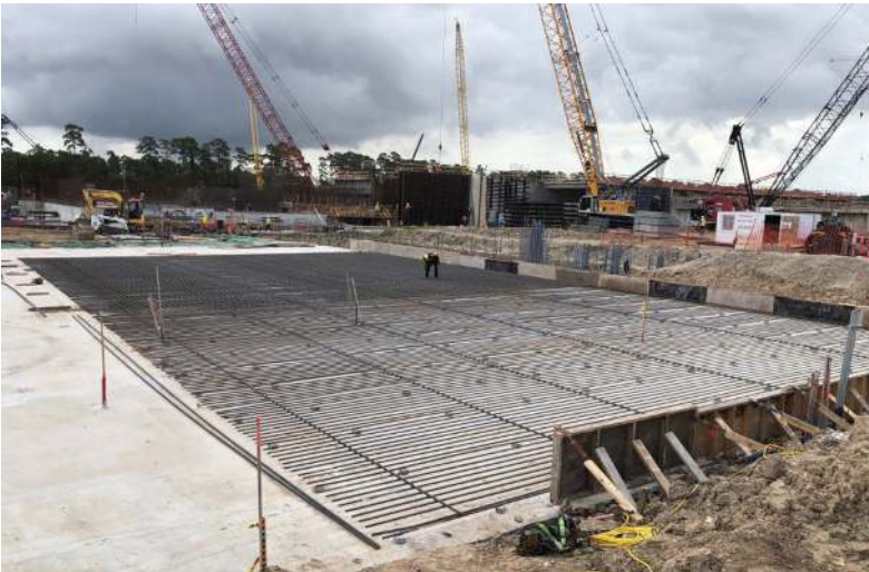
311-Post Chemical Rebar Installation
