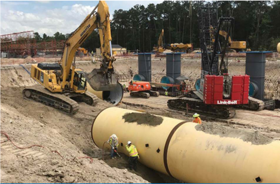
Installing 120" FW HSPS 1
