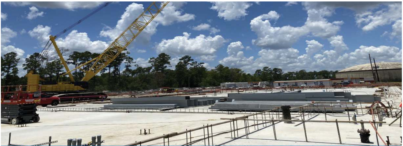
Finished Concrete Slab – Structural Steel Laid Out for Erecting at Facility 520
