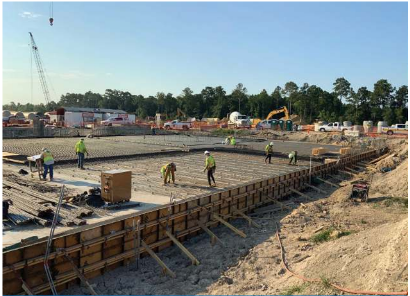
311-PostChemical: Installation of Rebar Slab A3, A4 – Tank Farm
