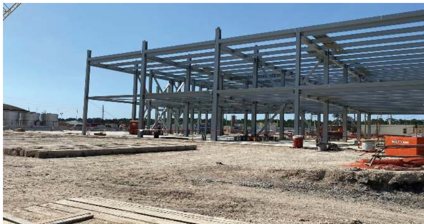
Structural Steel at Dewatering Building
