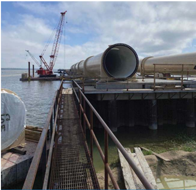
Bridge Piping on Span 6
