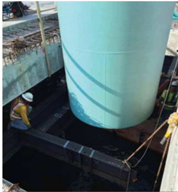
Final Pump Can Placement at IPS
