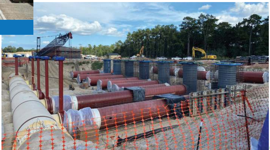
Installation of 78" Pipe HSPS 401
