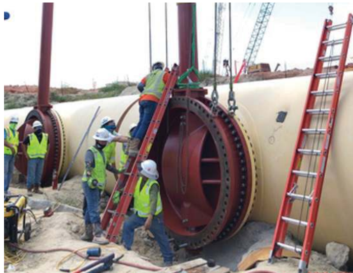
Setting 78" BFVs on 120" FW Corridor 5
