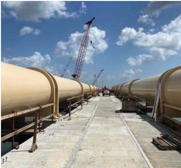
108" Bridge Piping Installation
