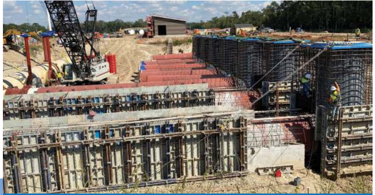
Installation of 78" Inlet Pipes and their Encasement at HSPS 401
