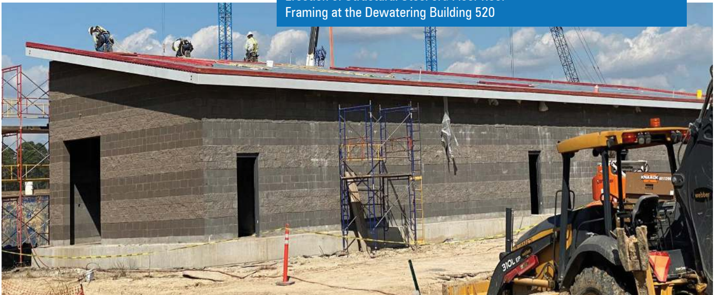
Installation of MSB 111 Roof Blocking Underway
