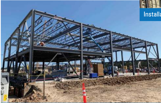
Completed Maintenance Building Steel Structure
