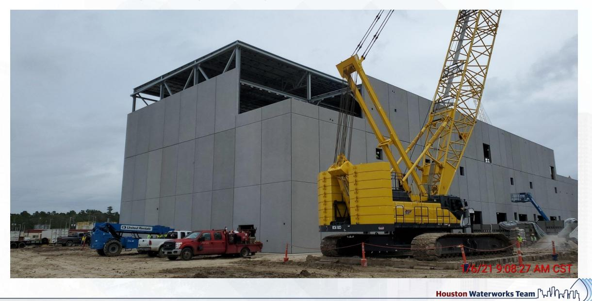
Installation of masonry 1st (Polymer storage), and 2nd (Electrical room/Polymer aging room) and installation of electrical & plumbing rough-in at the 1st floor at Fac 520
