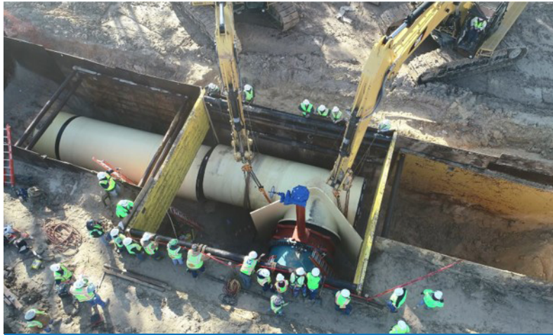
108"x102" Tee Installation Corridor 5
