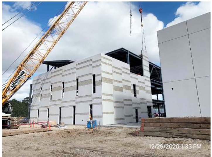
Admin Building Precast Panel Installation
