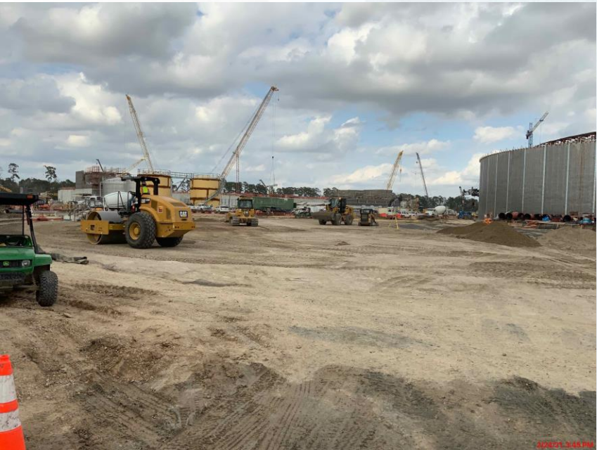
Finalizing soil preparation for floor footing forms and crane mobilization
