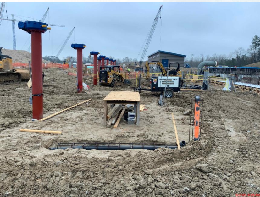
Continued under slab electrical and plumbing
