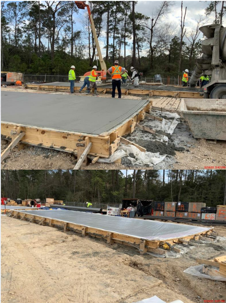
Commenced casting beds & precast wall panel pouring
