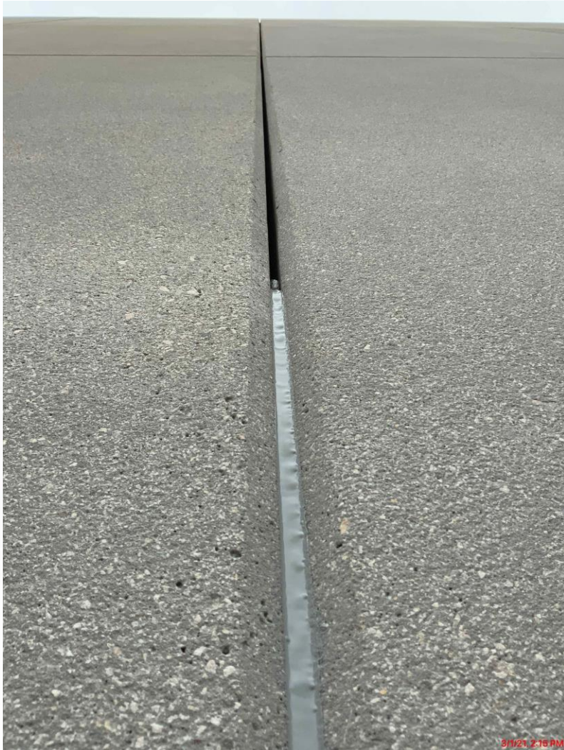
Continued installing caulking in-between precast panels
