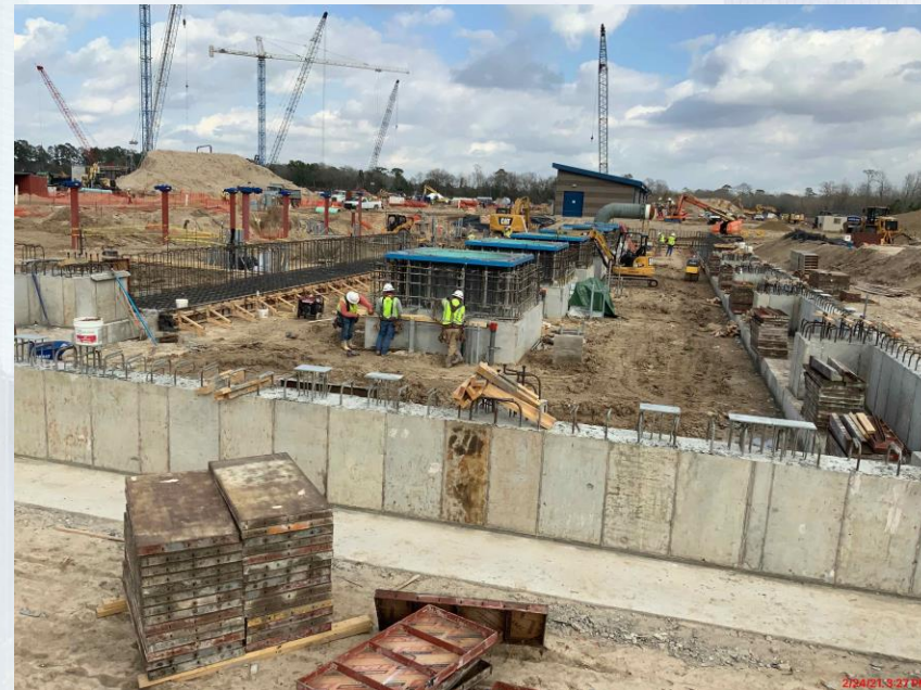
Pouring footers and foundation walls (Pump room)
