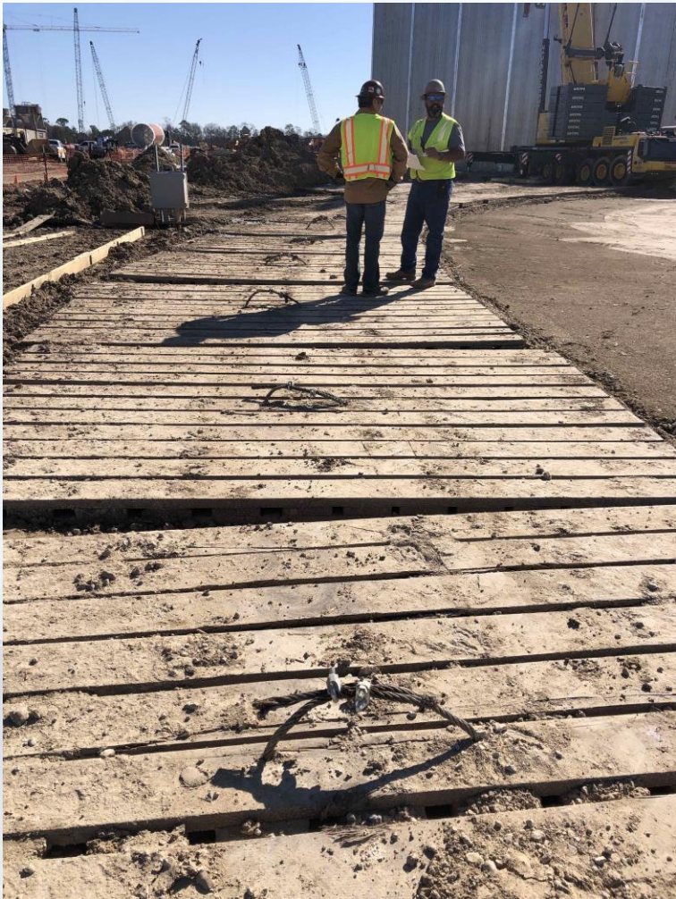
Finalizing soil preparation for floor footing forms and crane mobilization
