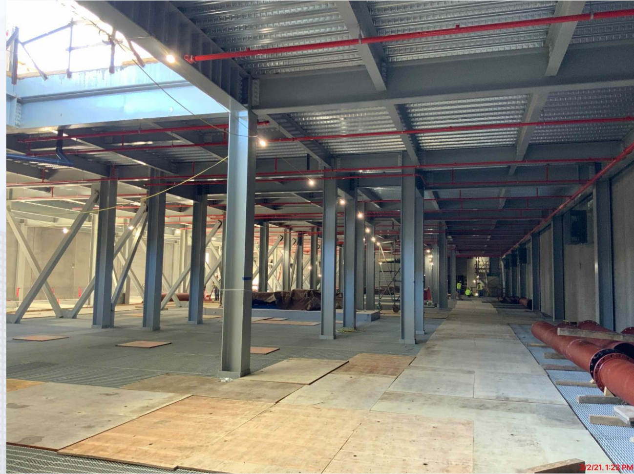
Continued installing fire piping on the 2nd & 3rd floors
