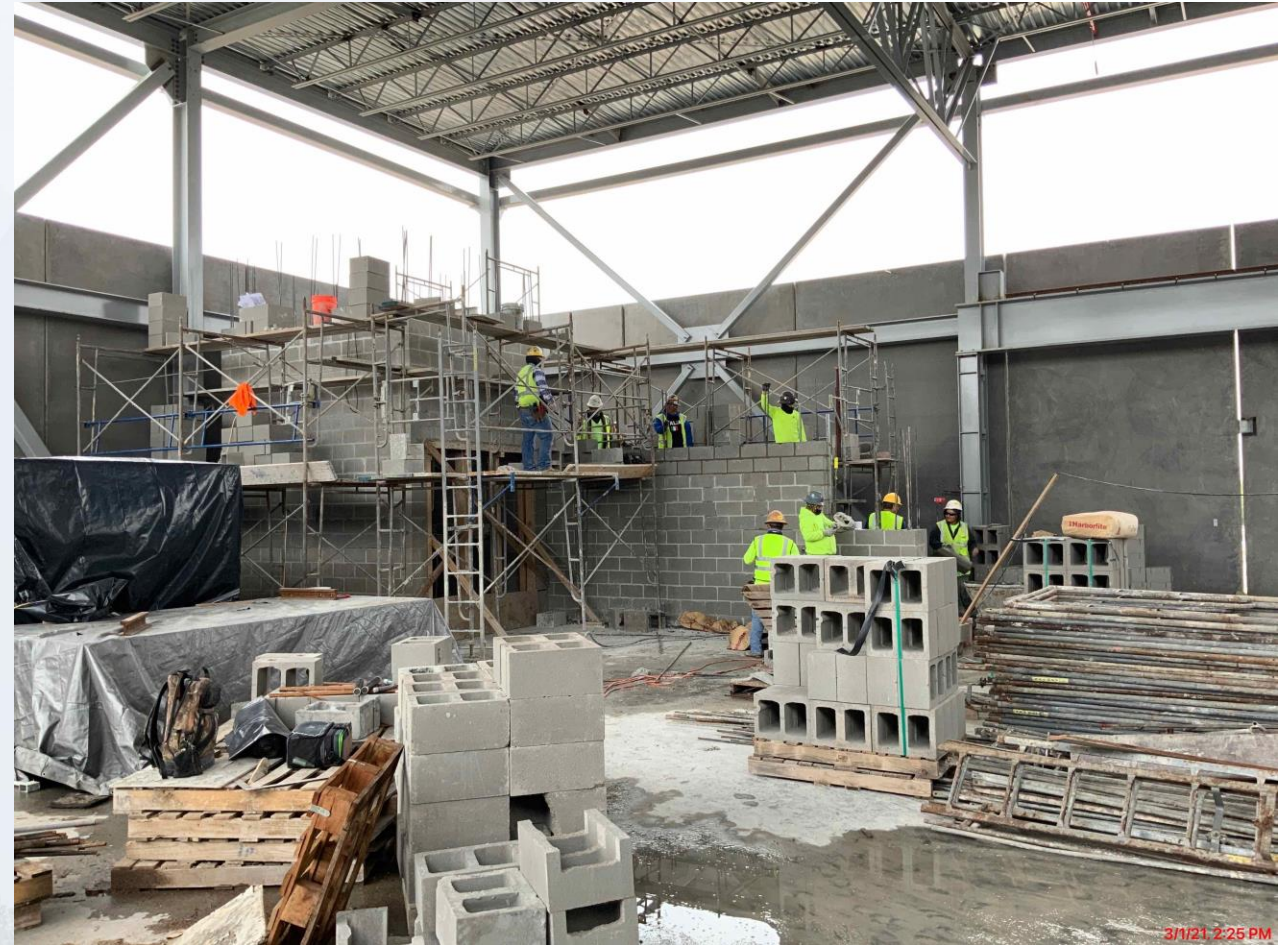
Continued installing CMU at the 3rd floor
