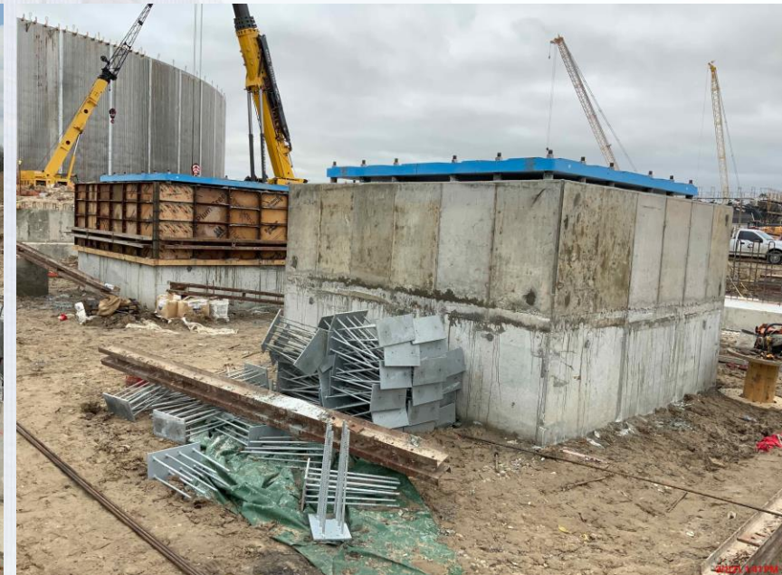
Pump can encasement is near completion
