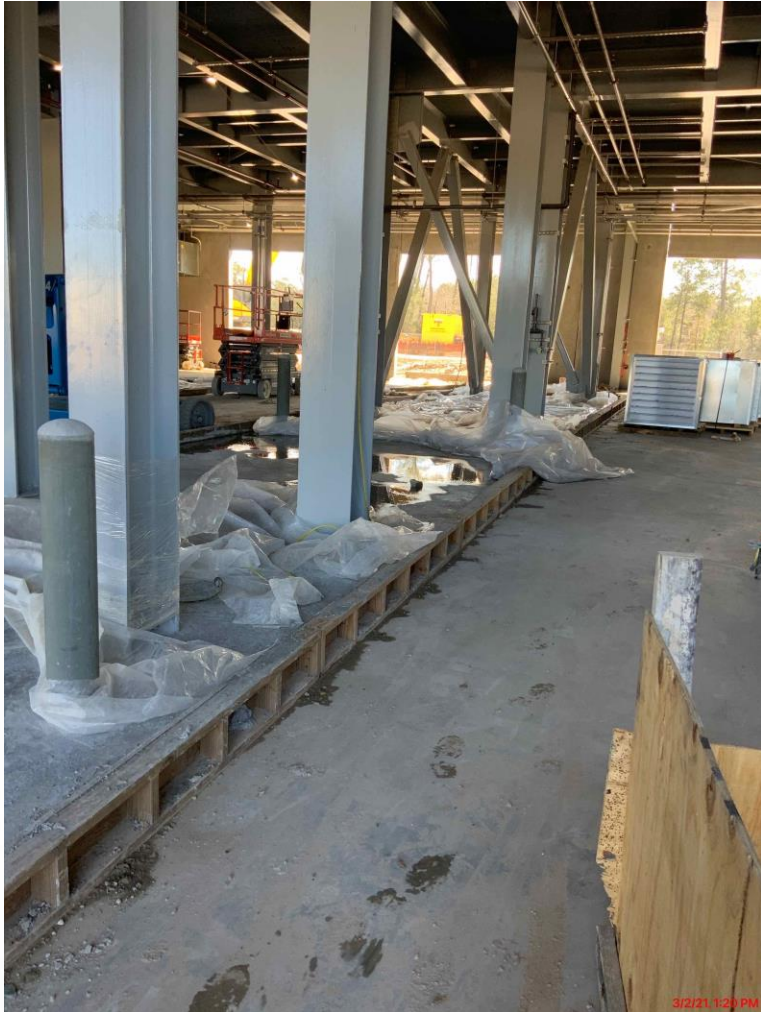
Continued installing equipment pads and walkway curb pads
