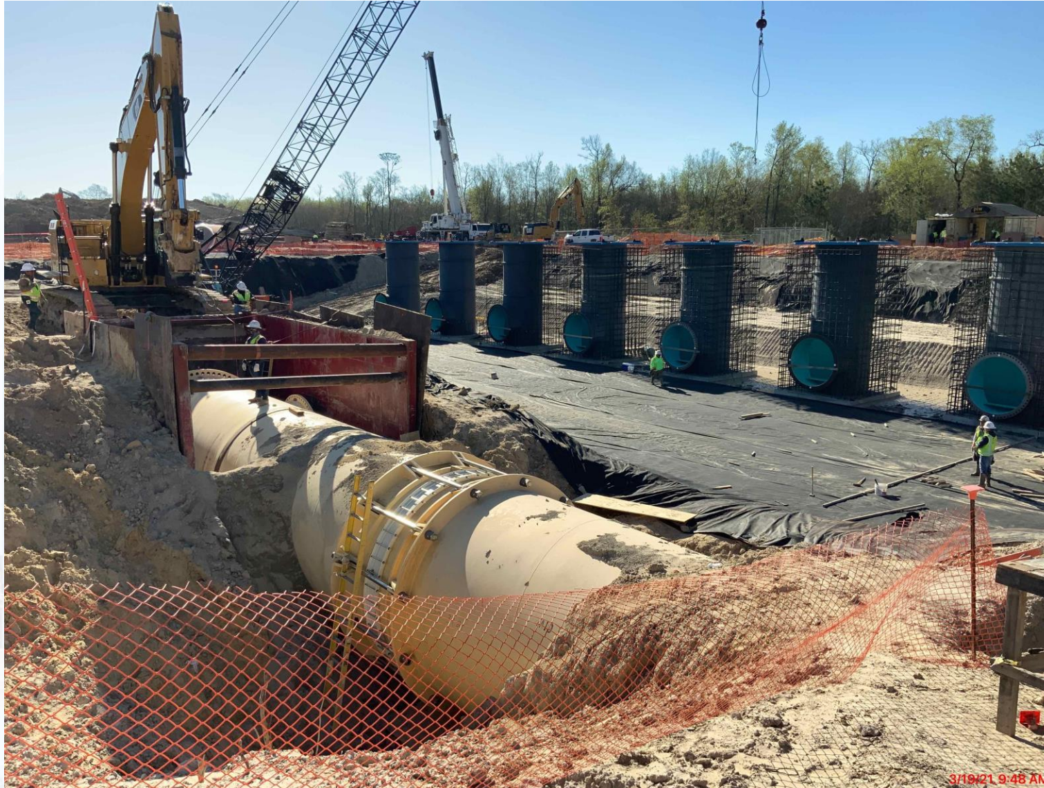
Site work to prepare for supports for 78" at Fac 402
