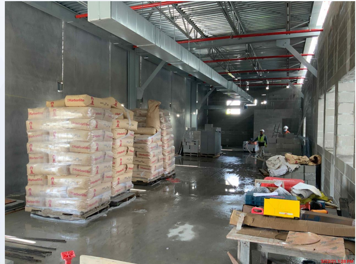
Continued installation of HVAC at the 2nd & 3rd floor at Fac 520
