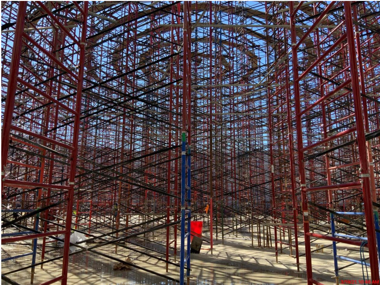
Continued shoring erection at GST 362
