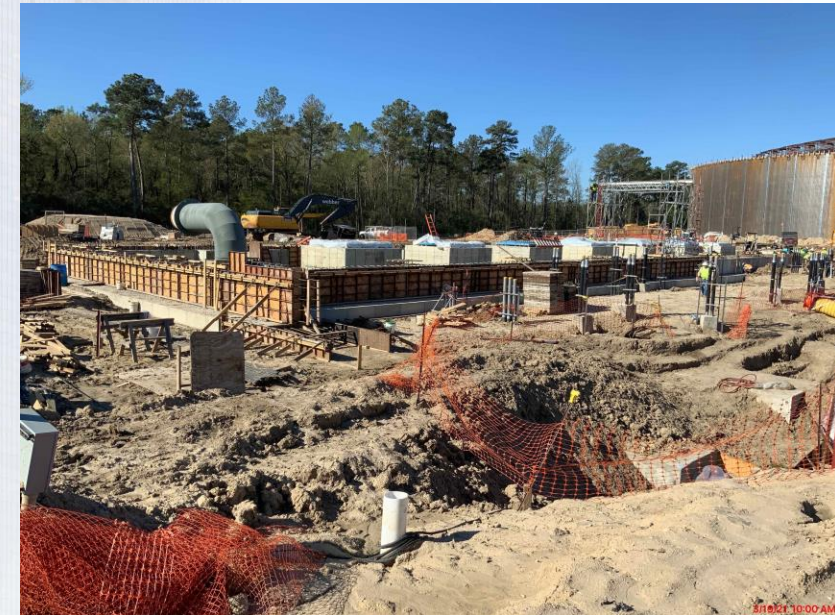
Final backfilling around 48" and 102" header at Fac 401
