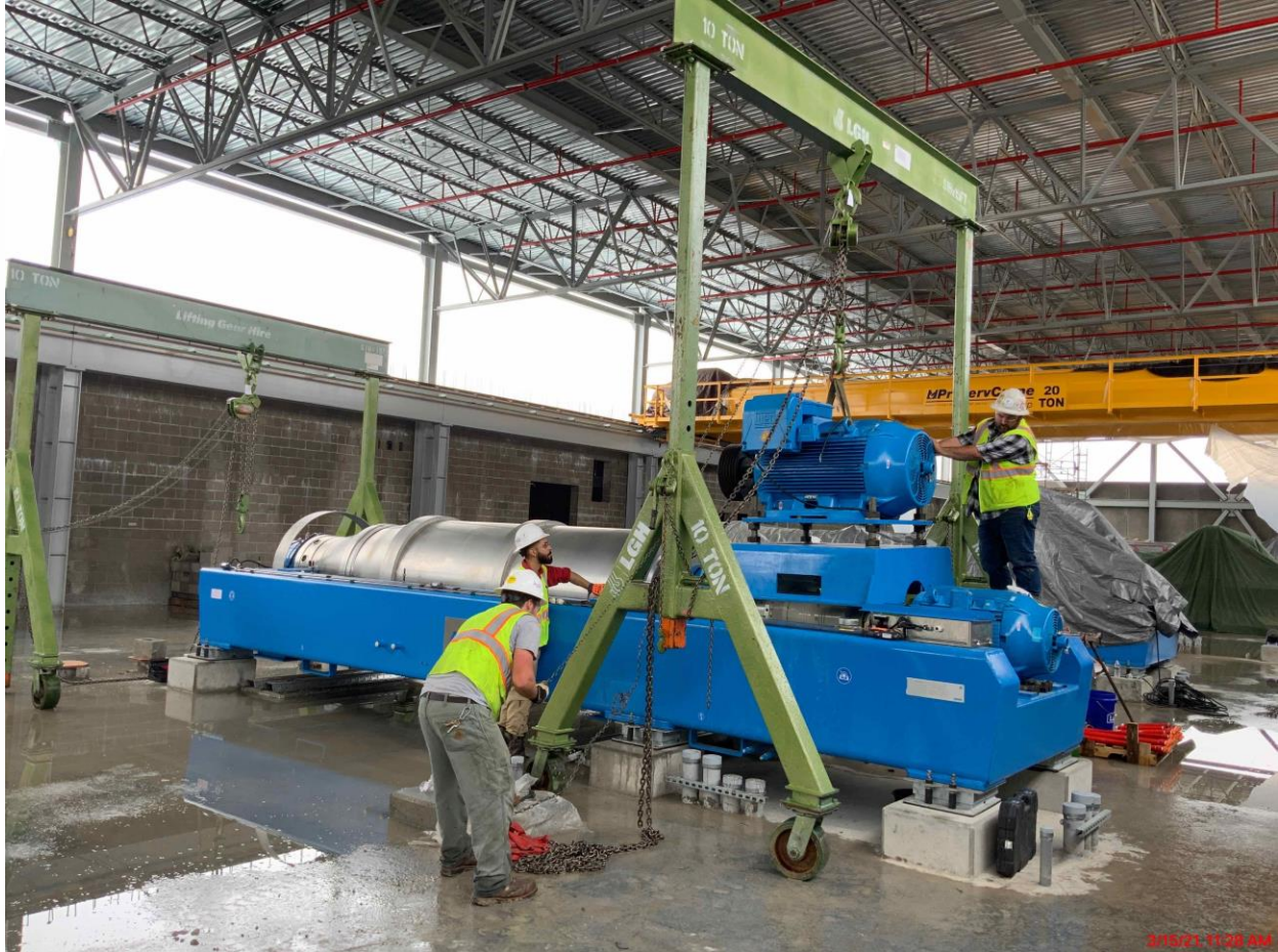
Centrifuges have been put into Maintenance mode and have been rotated per manufacturer recommendations
