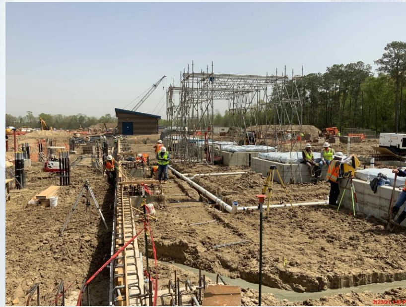
Installing under slab electrical & plumbing utilities at Fac 401
