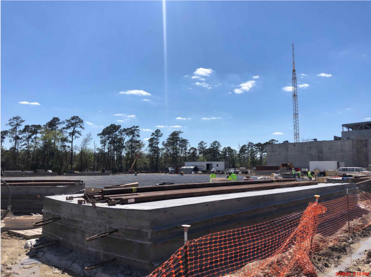
Completed wall panel pouring at GST 361
