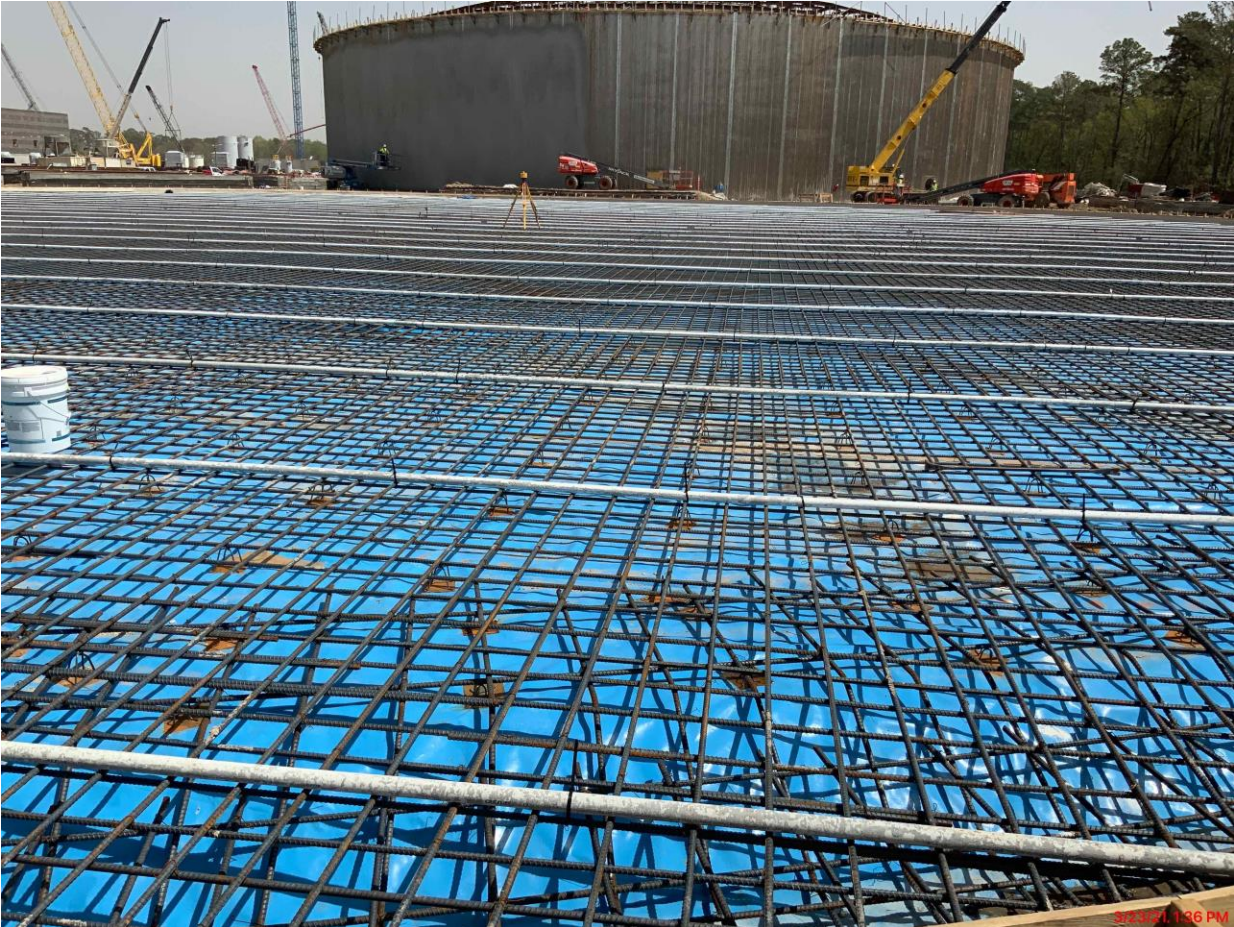
Commenced footing and floor reinforcing at GST 361
