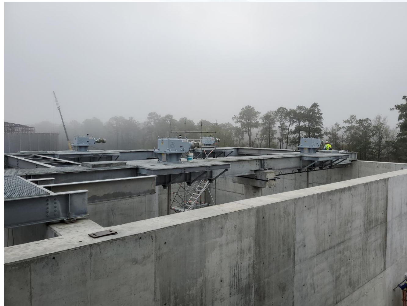
Commenced placement of mixers
