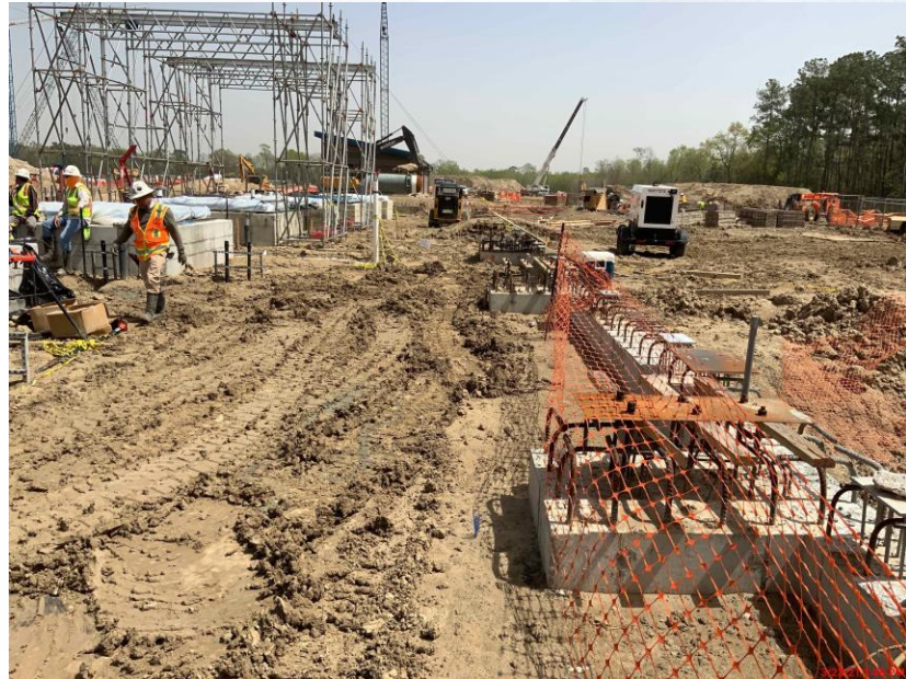
Forming footers for the pump room at Fac 401
