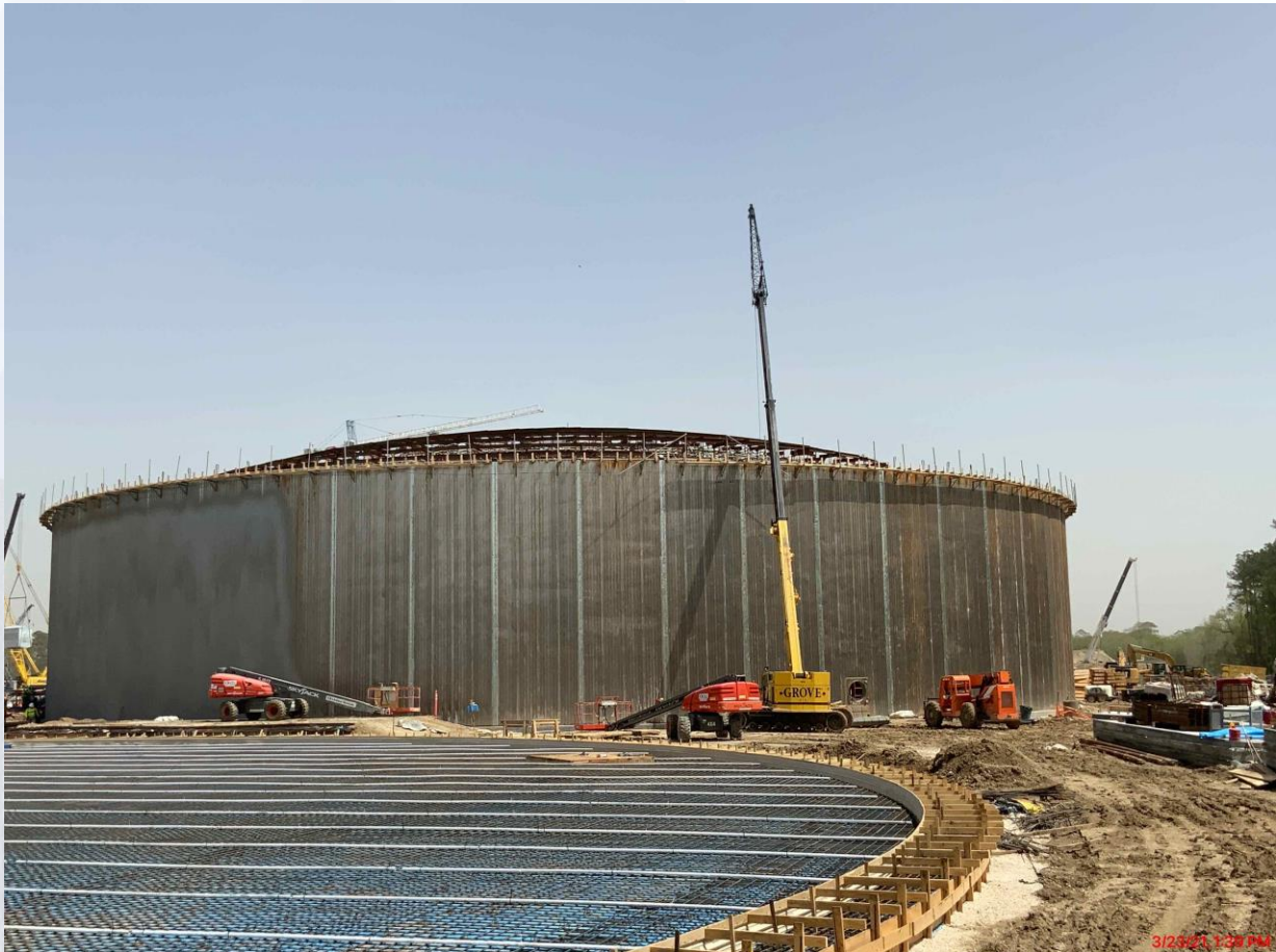
Completed interior shotcrete diaphragm and commenced exterior at GST 362
