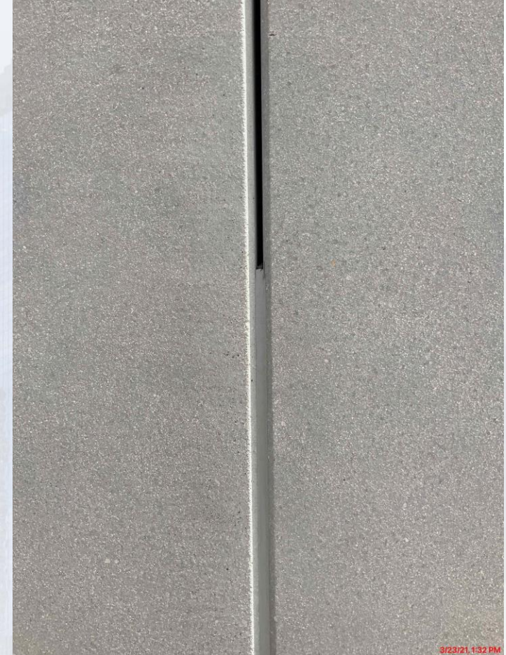
Continued installing caulking in-between precast panels
