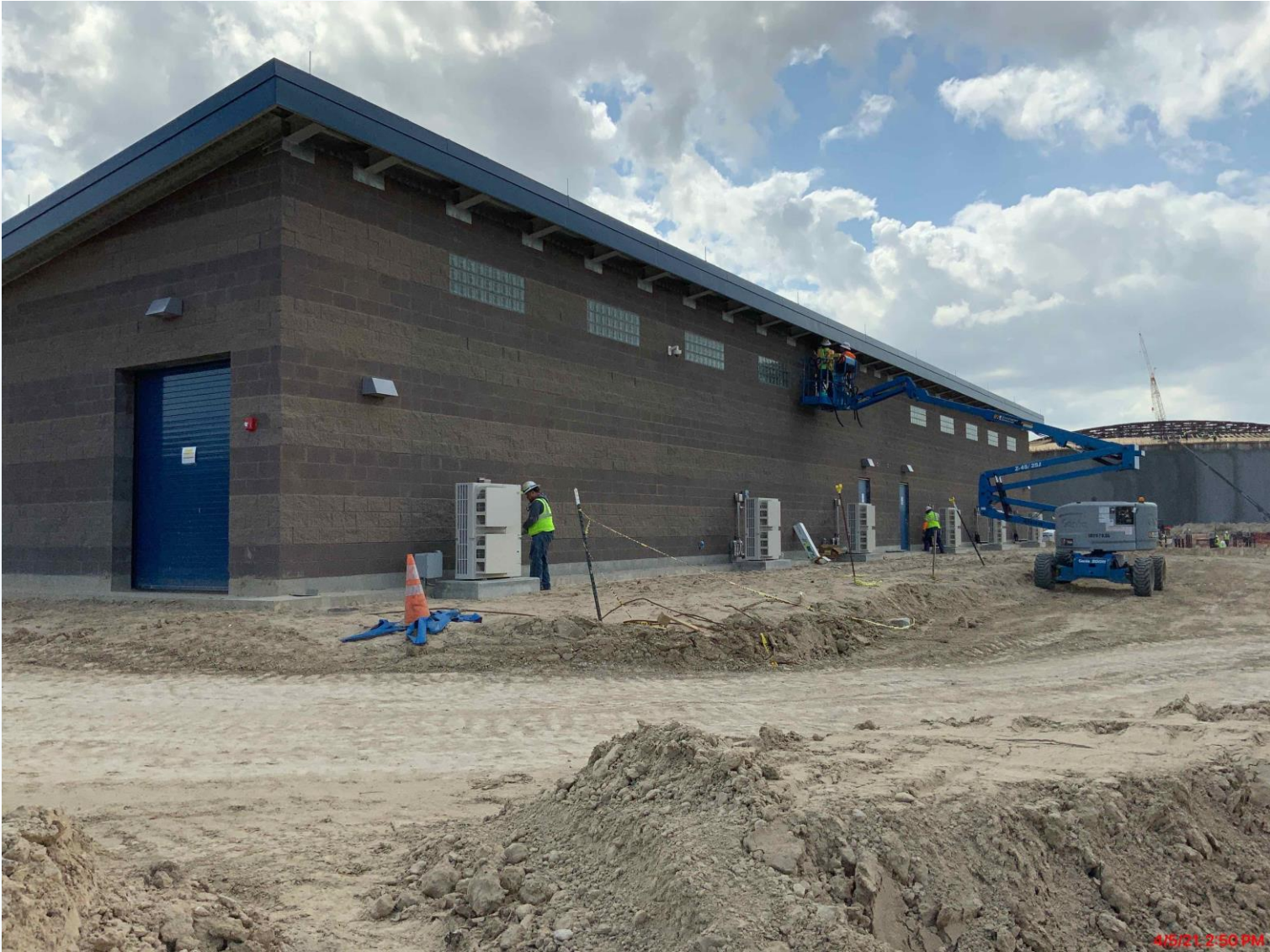
Installation of closure plates
