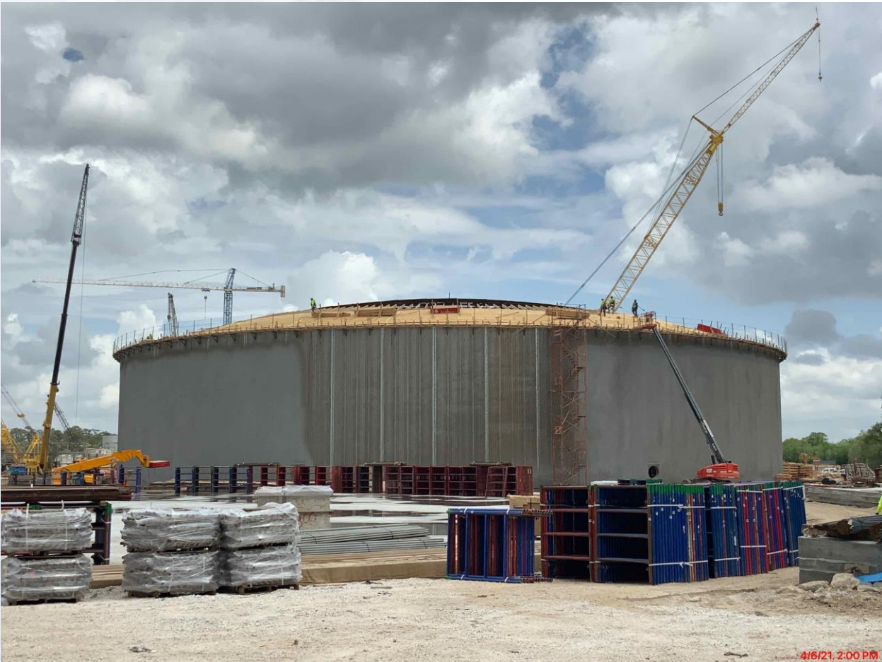
Continued shoring erection at GST 362
