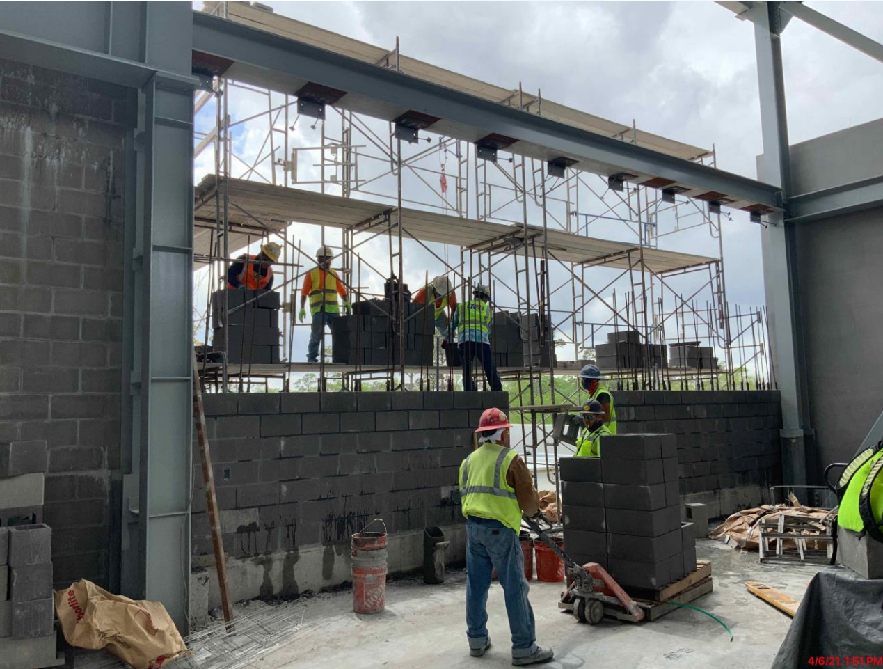
Continued installing CMU at the 3rd floor at Fac 520
