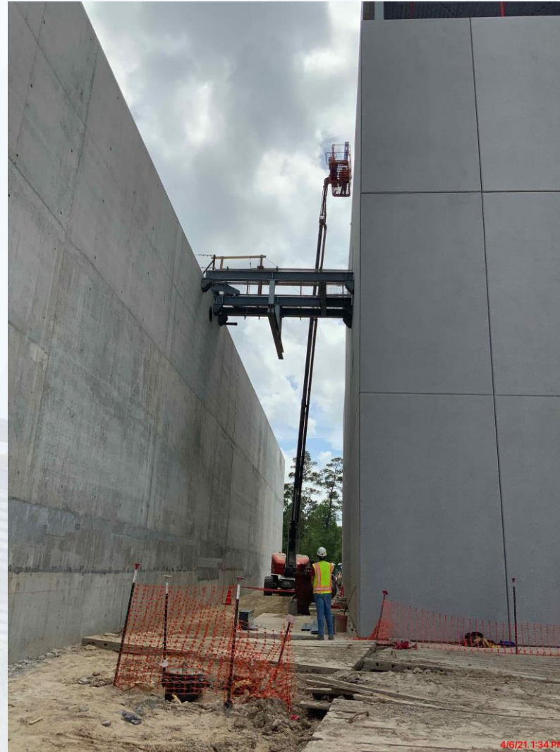
Commenced installation of structural steel stairs and bridge at Fac 510
