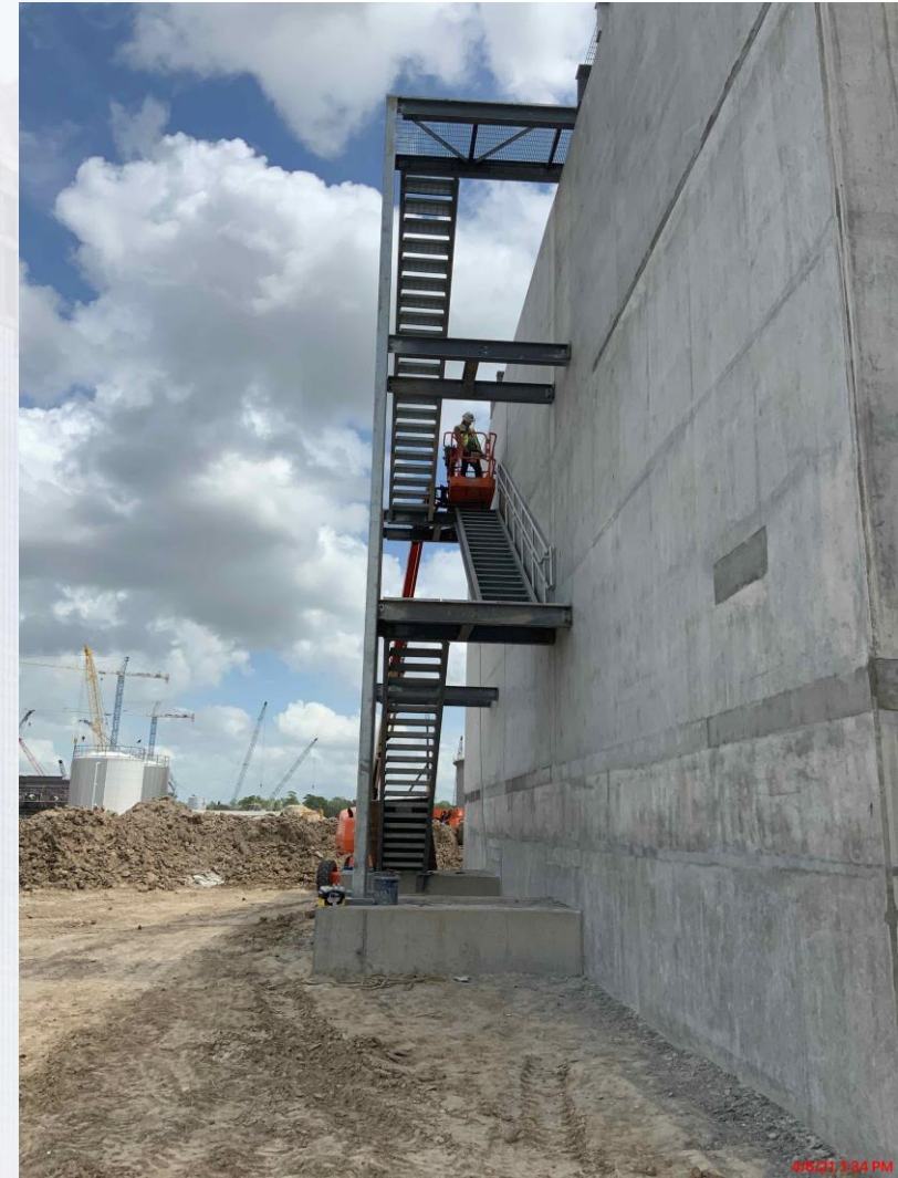
Commenced installation of structural steel stairs and bridge at Fac 510
