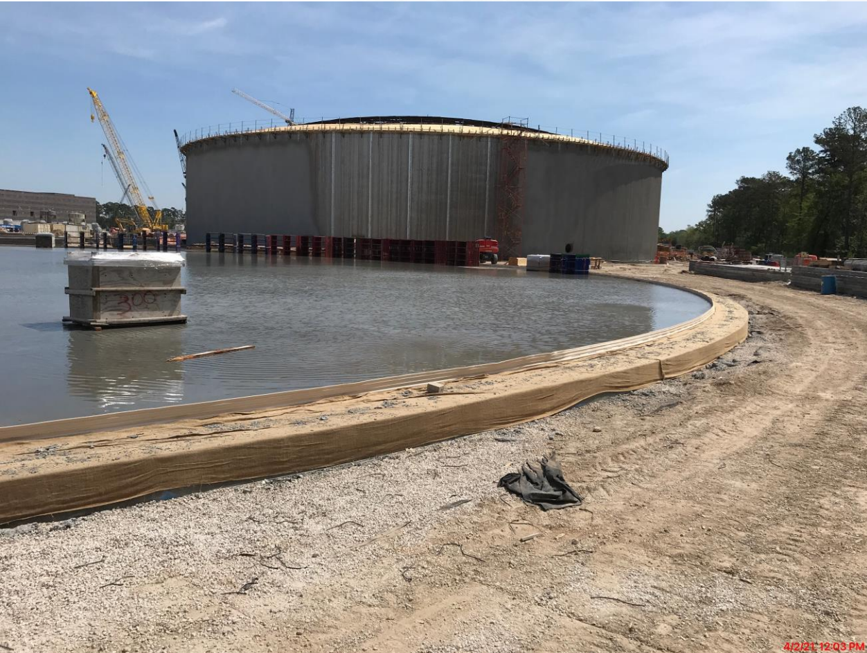
Curing concrete membrane slab & delivery of shoring material
