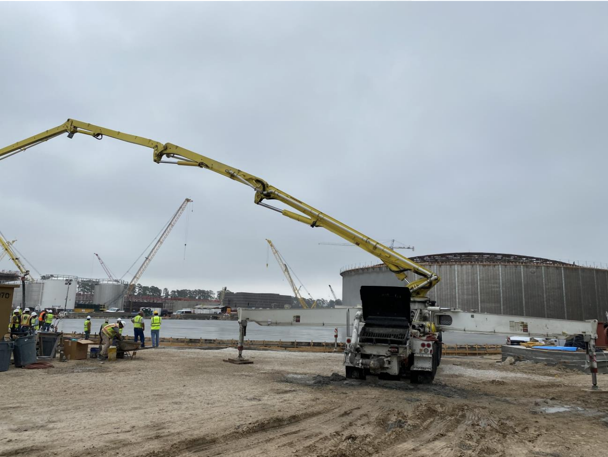
Pouring concrete slab of GST 361
