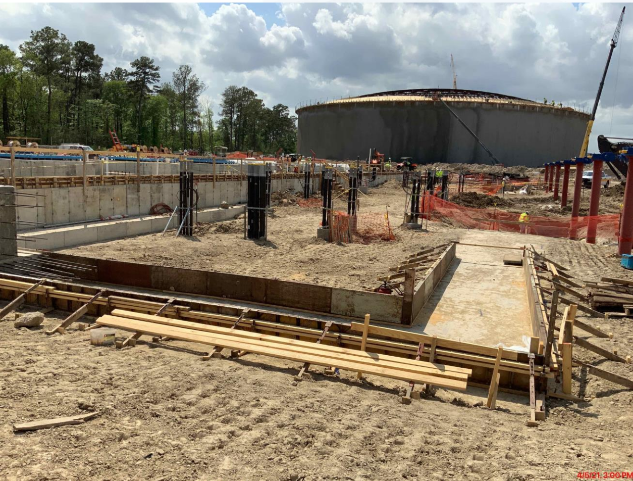
Commenced forming footers for the electrical room at Fac 401
