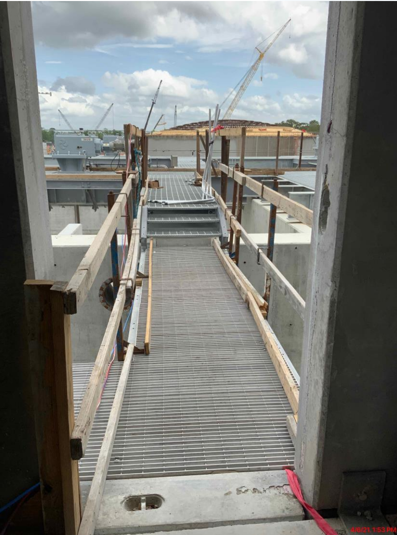
Commenced installation of structural steel stairs and bridge at Fac 510
