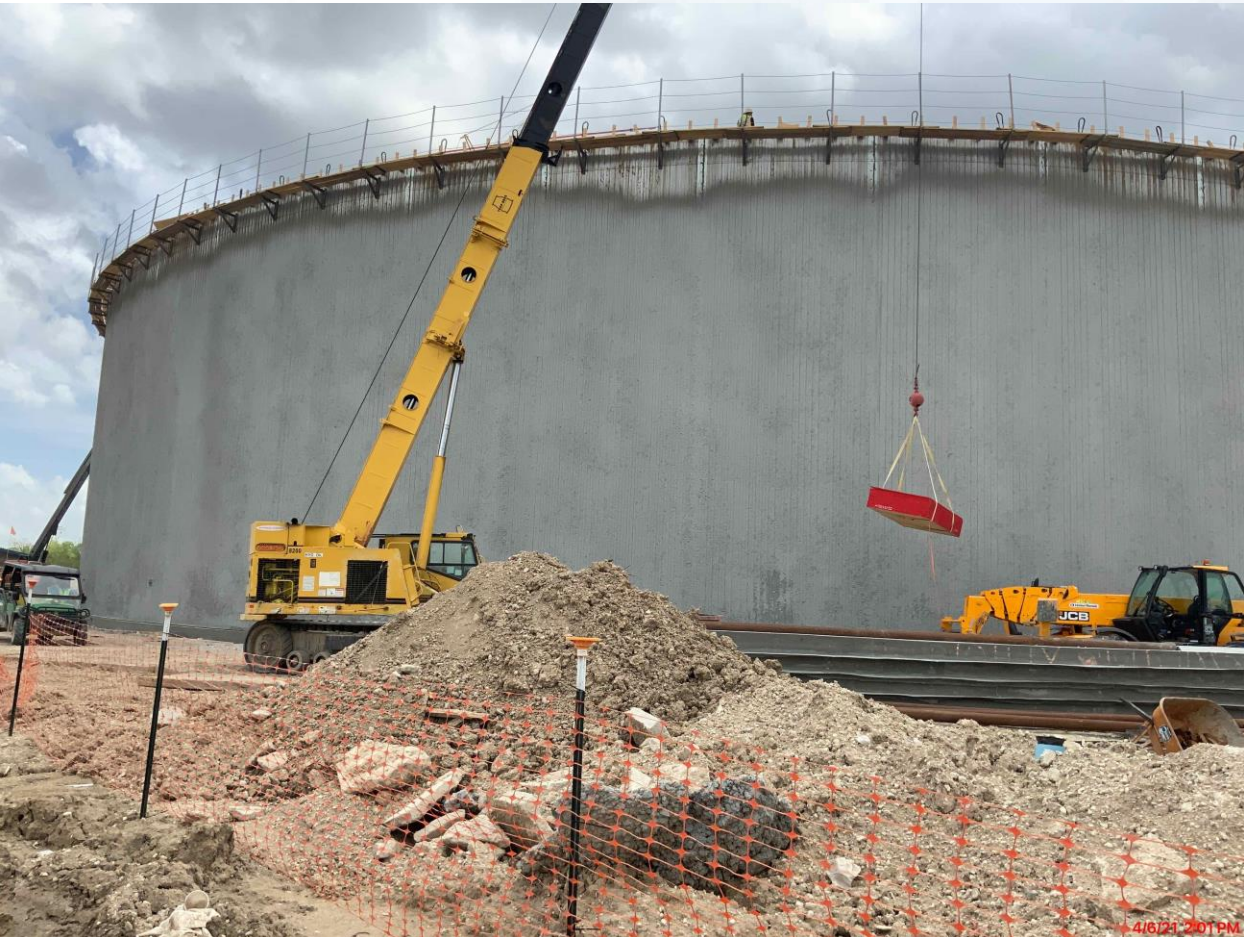
Continued exterior shotcrete at GST 362
