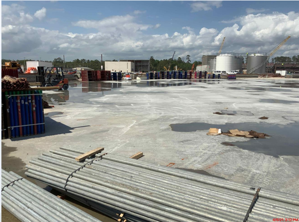
Curing concrete membrane slab & delivery of shoring material
