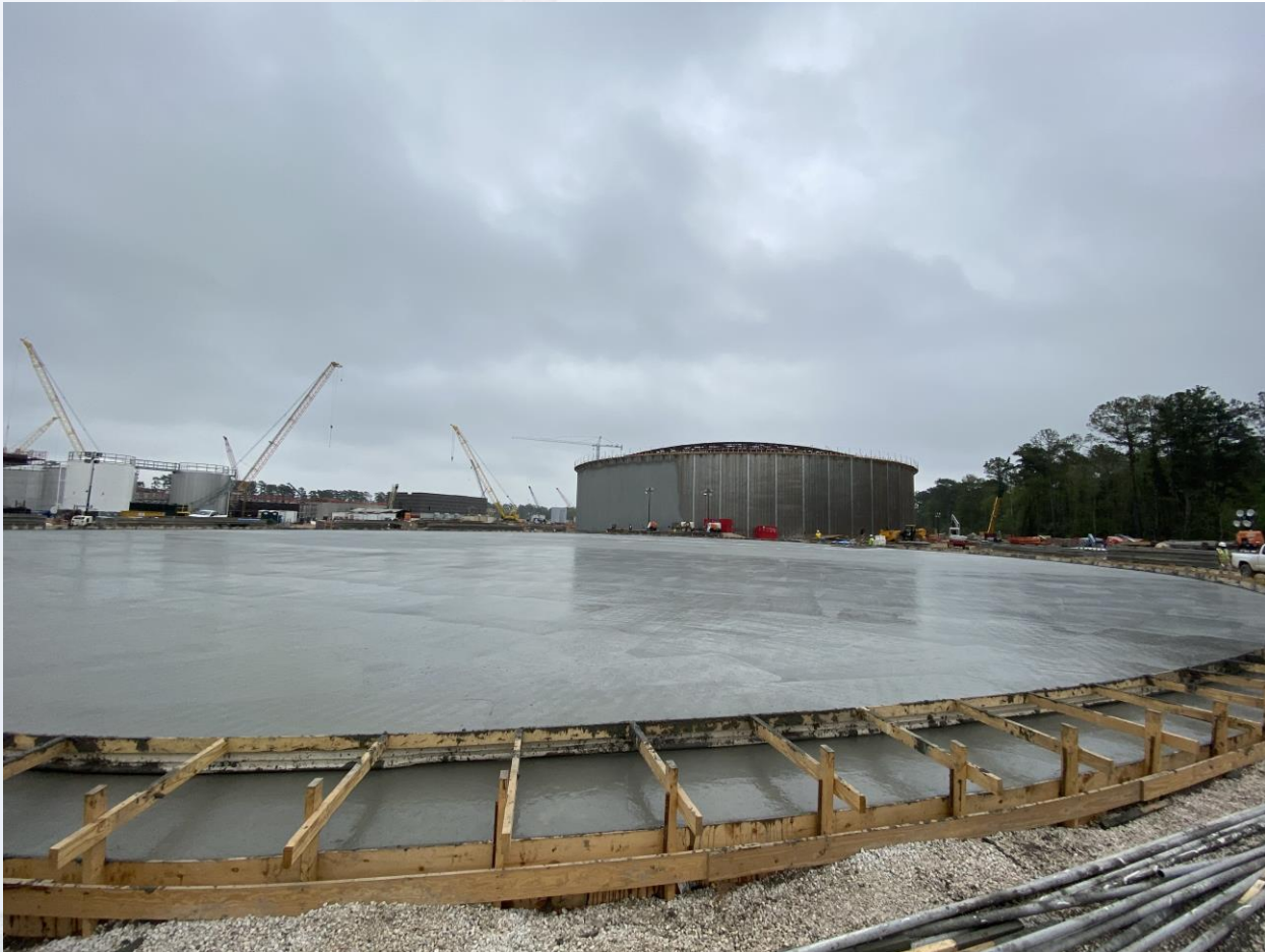
Pouring concrete slab of GST 361
