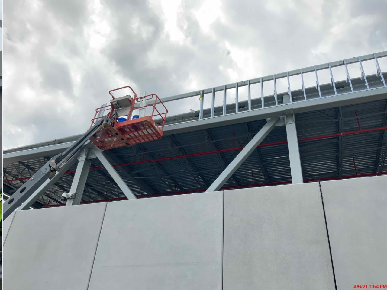
Commenced cold metal framing at Fac 520
