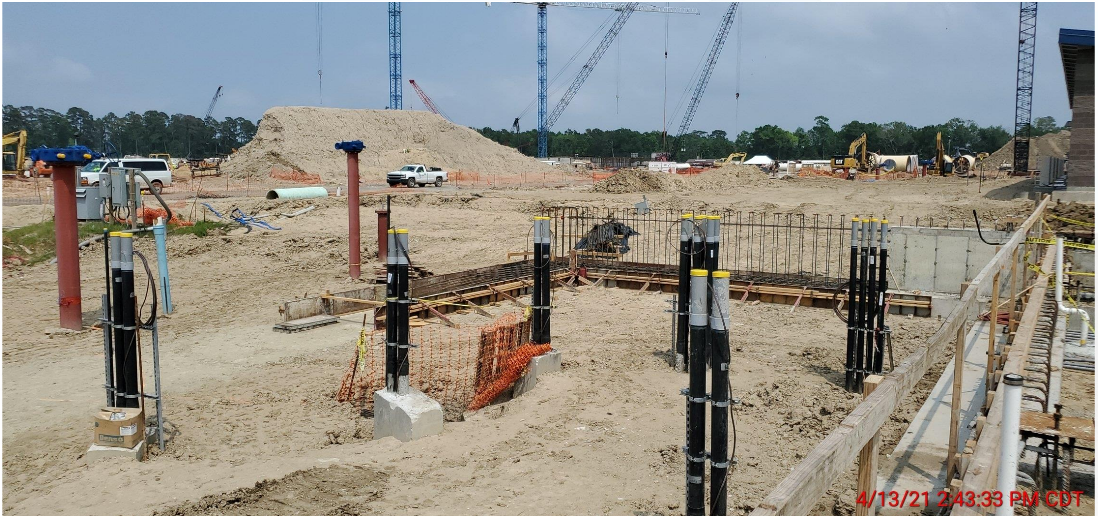
Commenced forming footers for the electrical room at Fac 401
