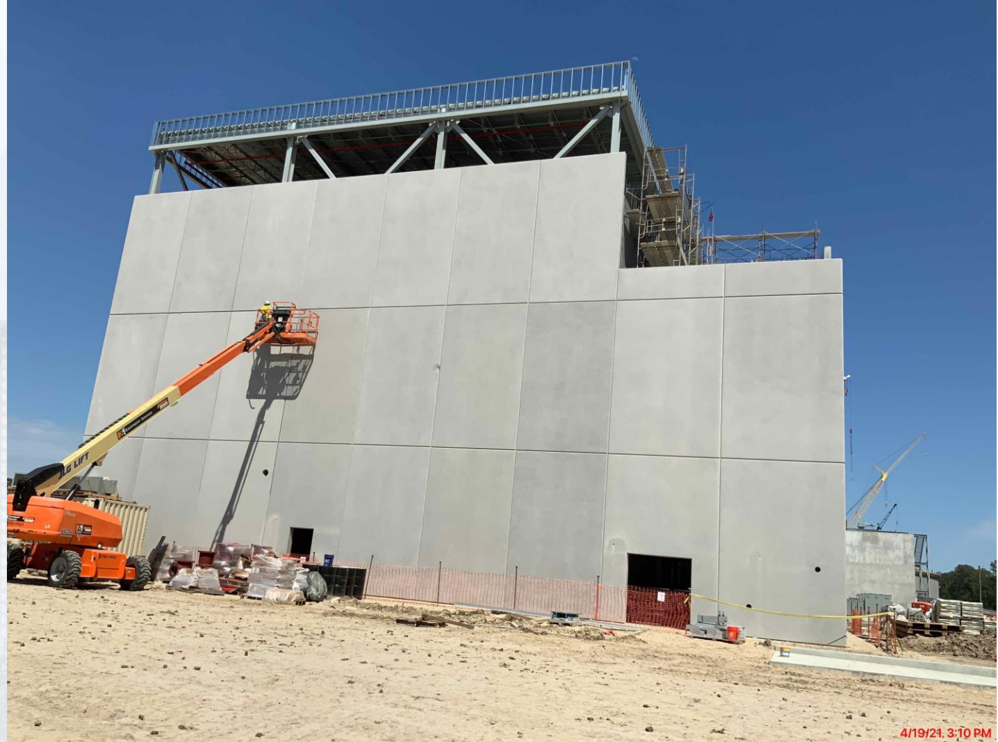
Continued installation of cold metal framing at Fac 520
