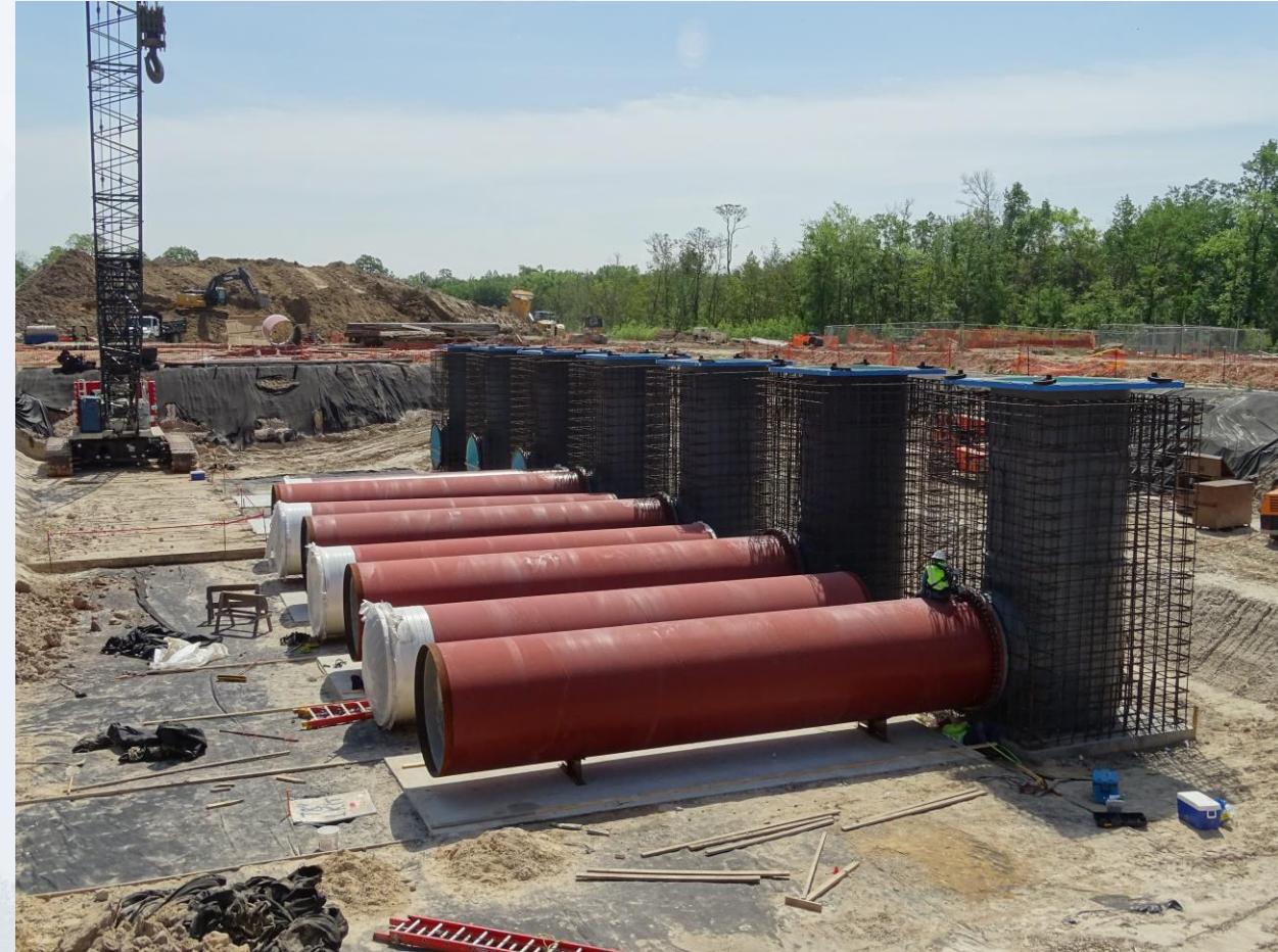
Installation of the 78" pipe at Fac 402
