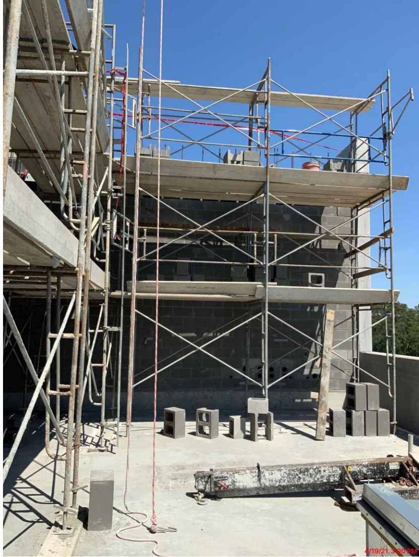
Continued installing CMU at the 3rd floor at Fac 520
