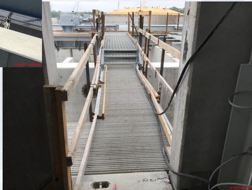
Completed installation of structural steel at Fac 510
