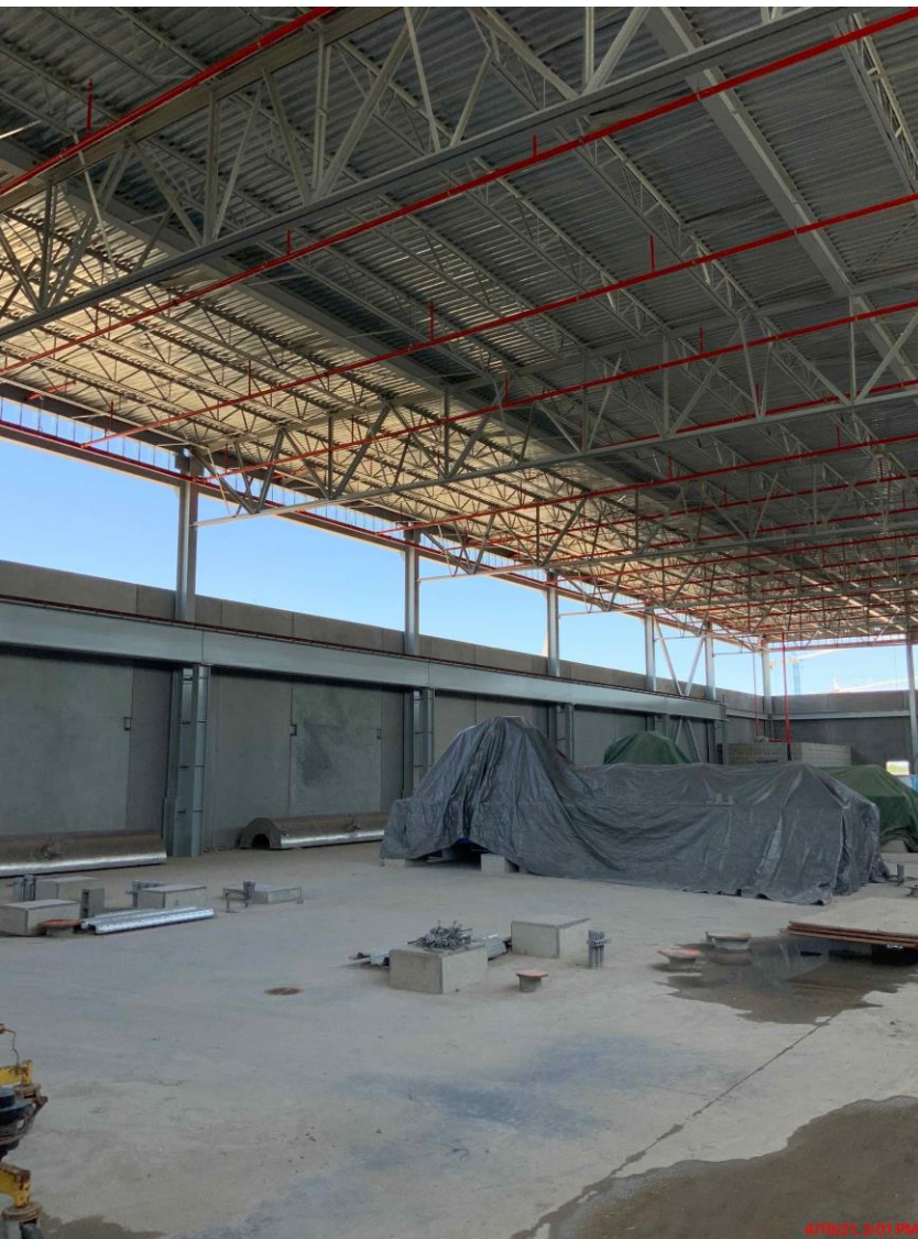
Installation of fire piping on the 3rd floor at Fac 520 is near completion
