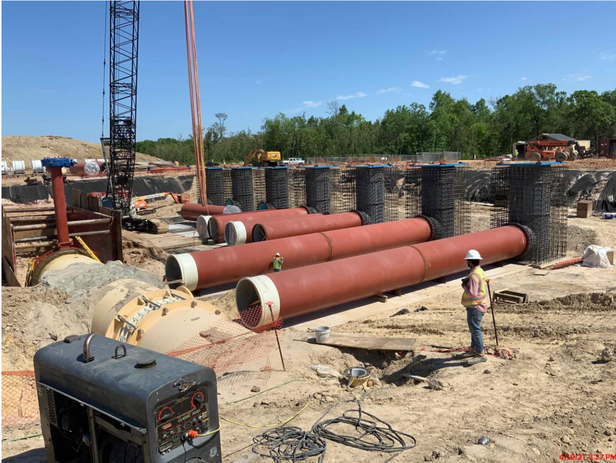
Installation of the 78" pipe at Fac 402
