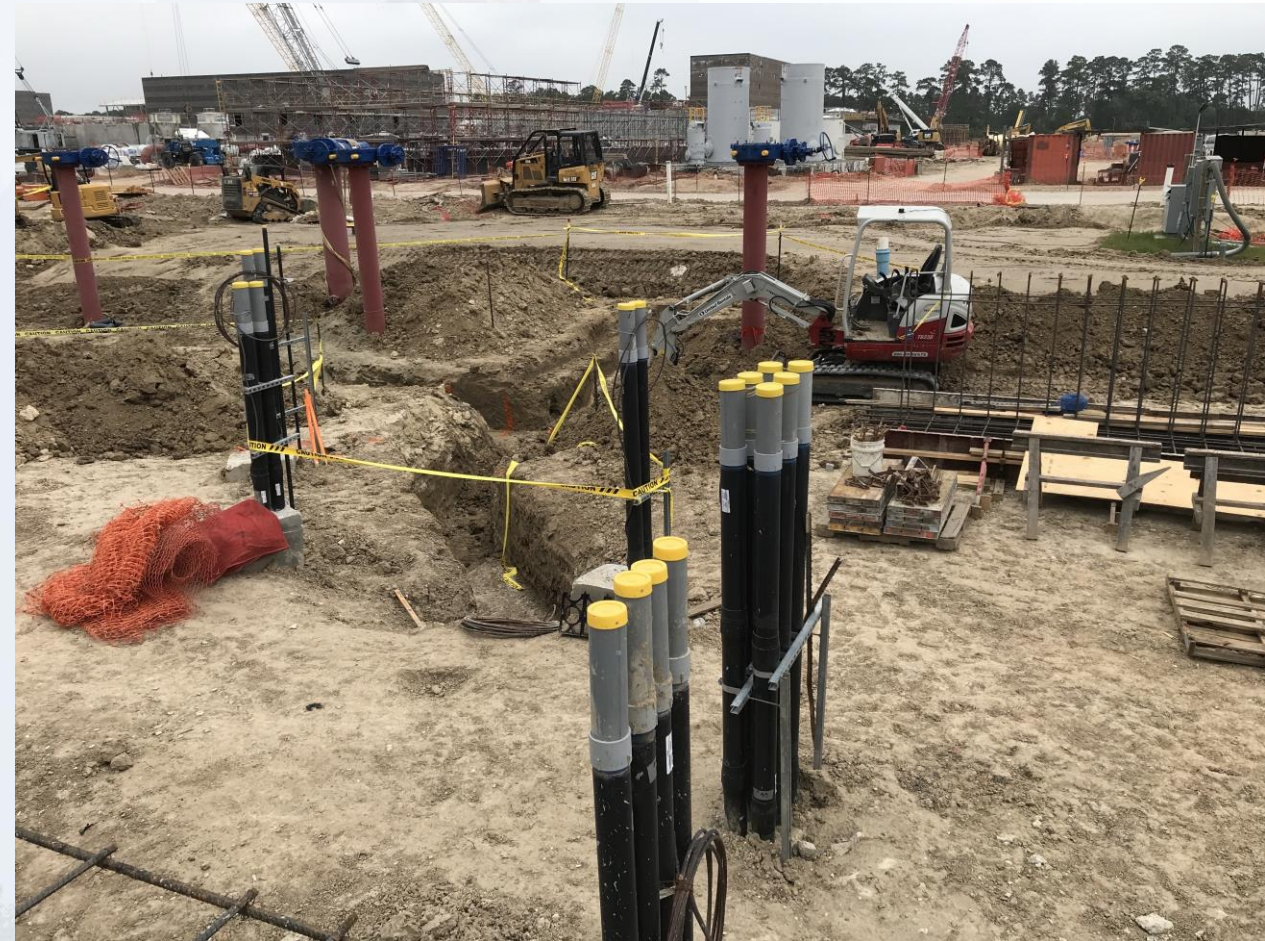
Continued installing under slab electrical & plumbing utilities at Fac 401
