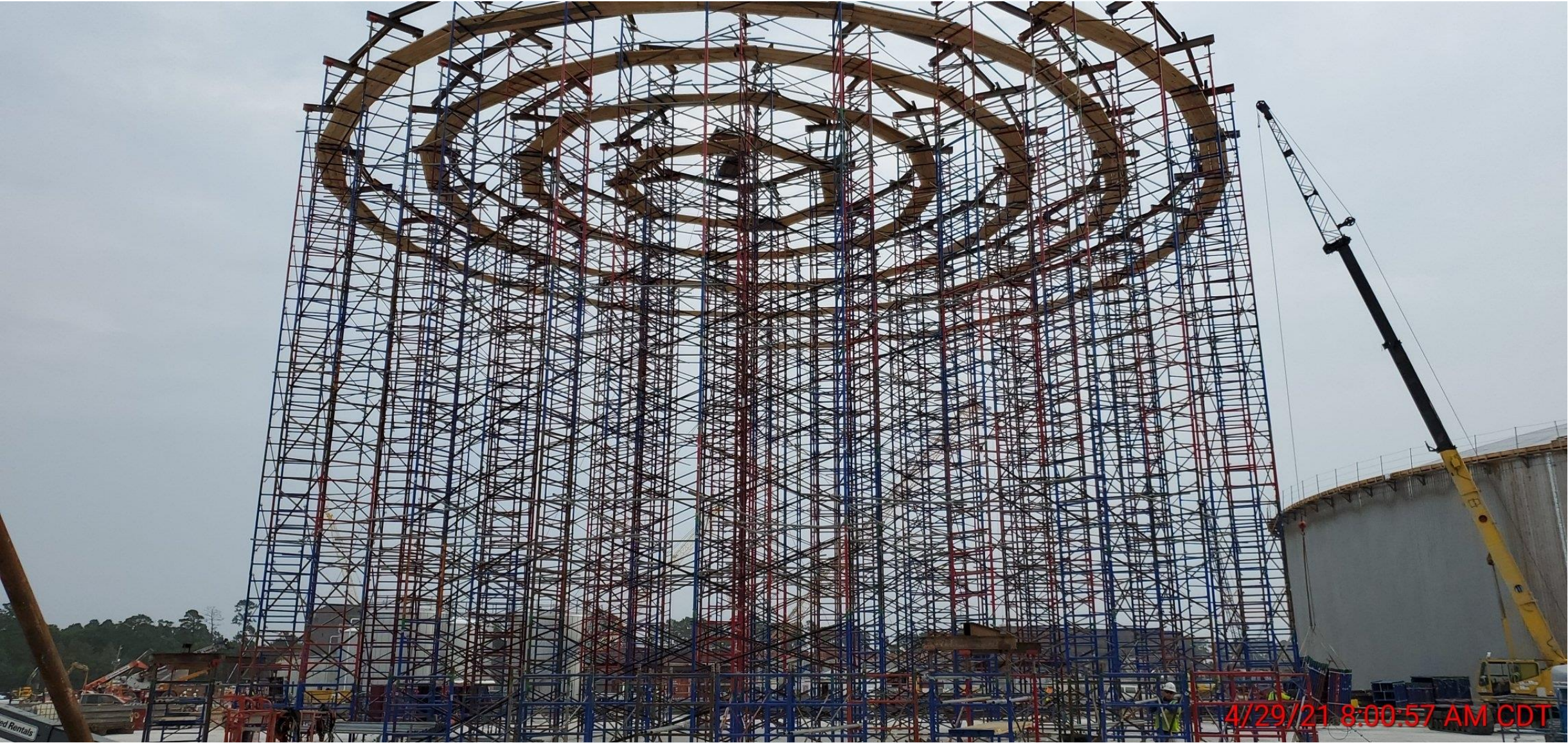
Commenced shoring erection at GST 361
