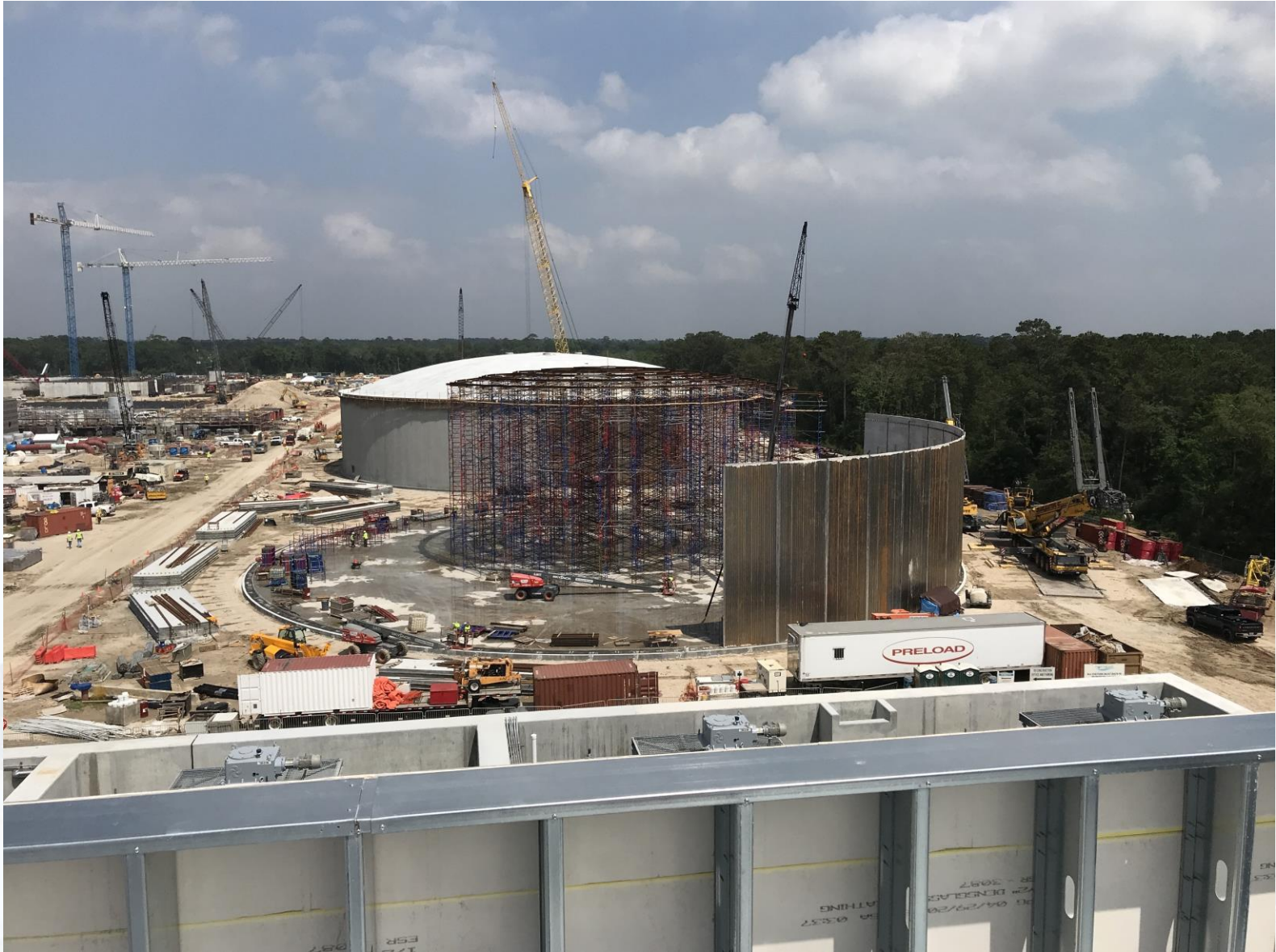
Commenced precast wall panel installation at GST 361
