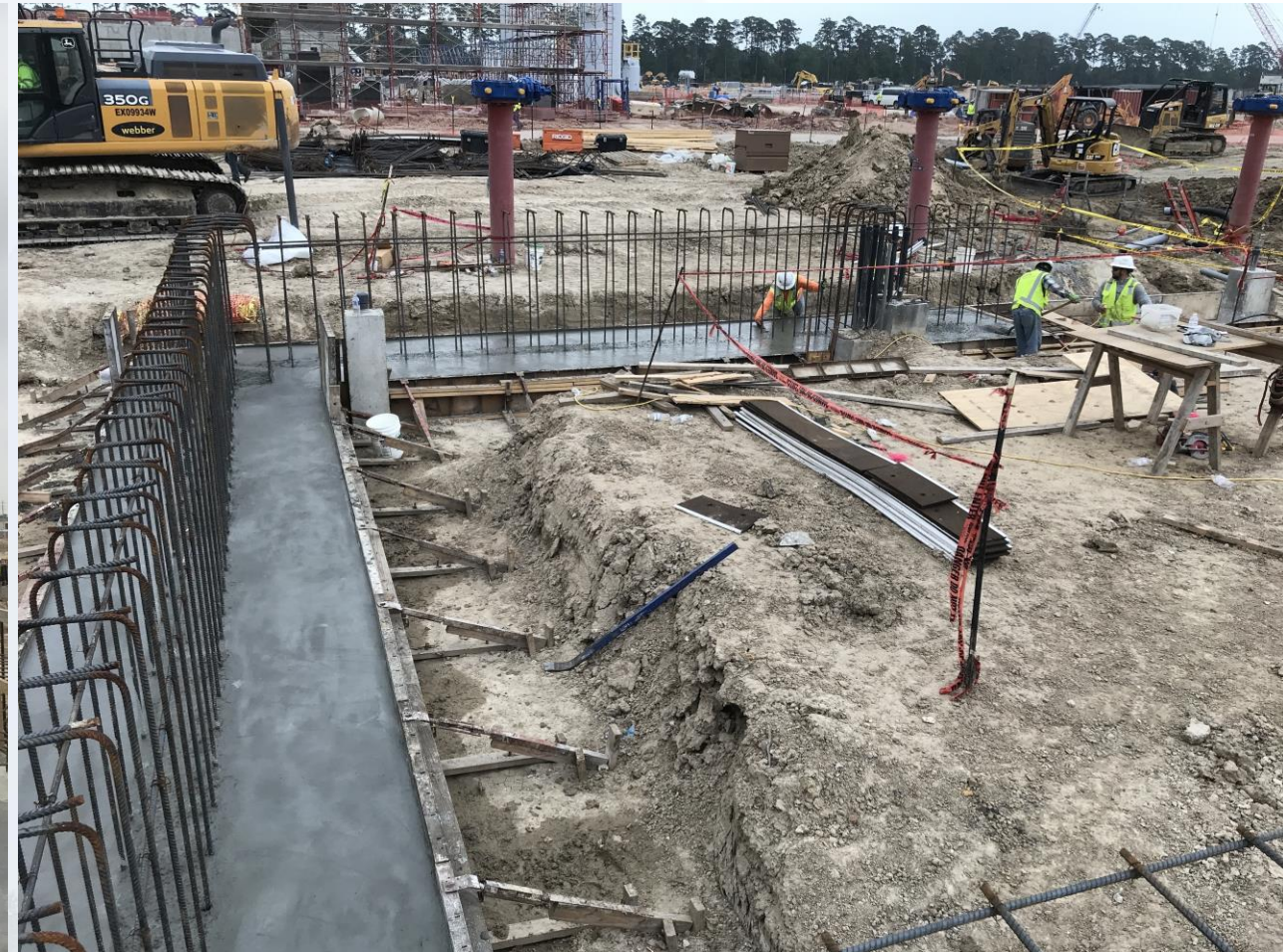
Continued forming footers for the electrical room at Fac 401
