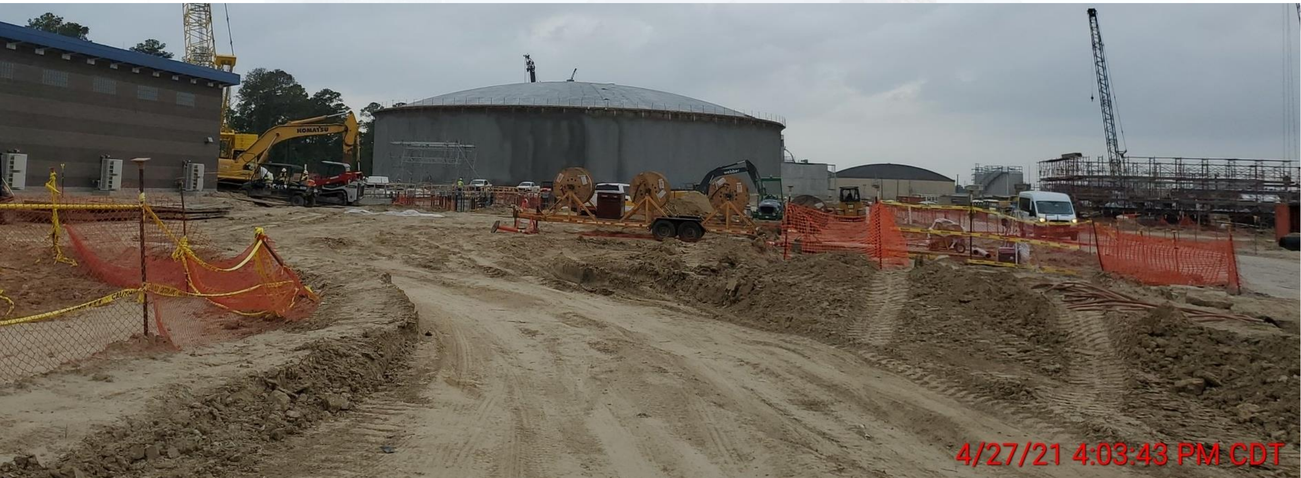
Completed dome Concrete at GST 362
