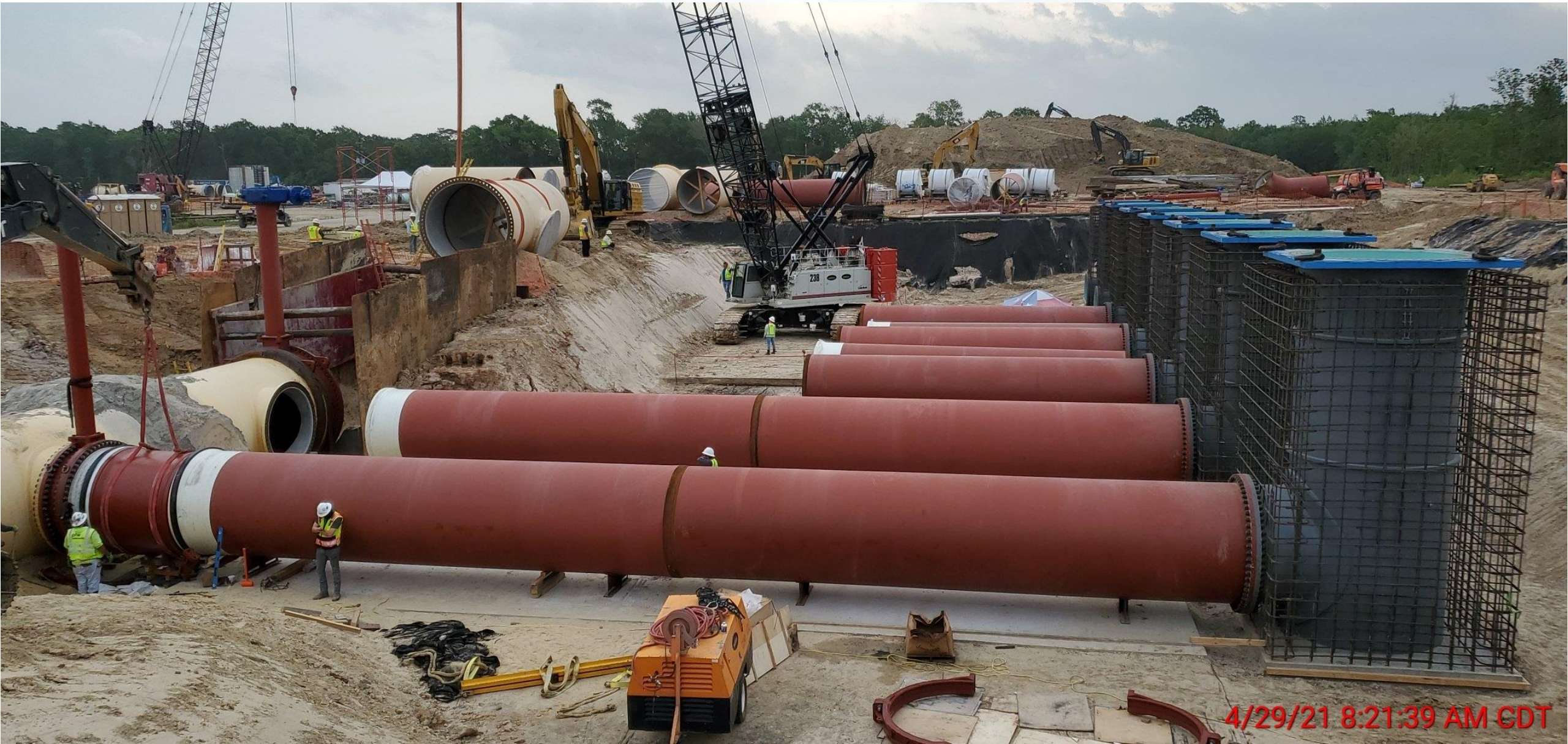
Installation of the 78" pipe at Fac 402
