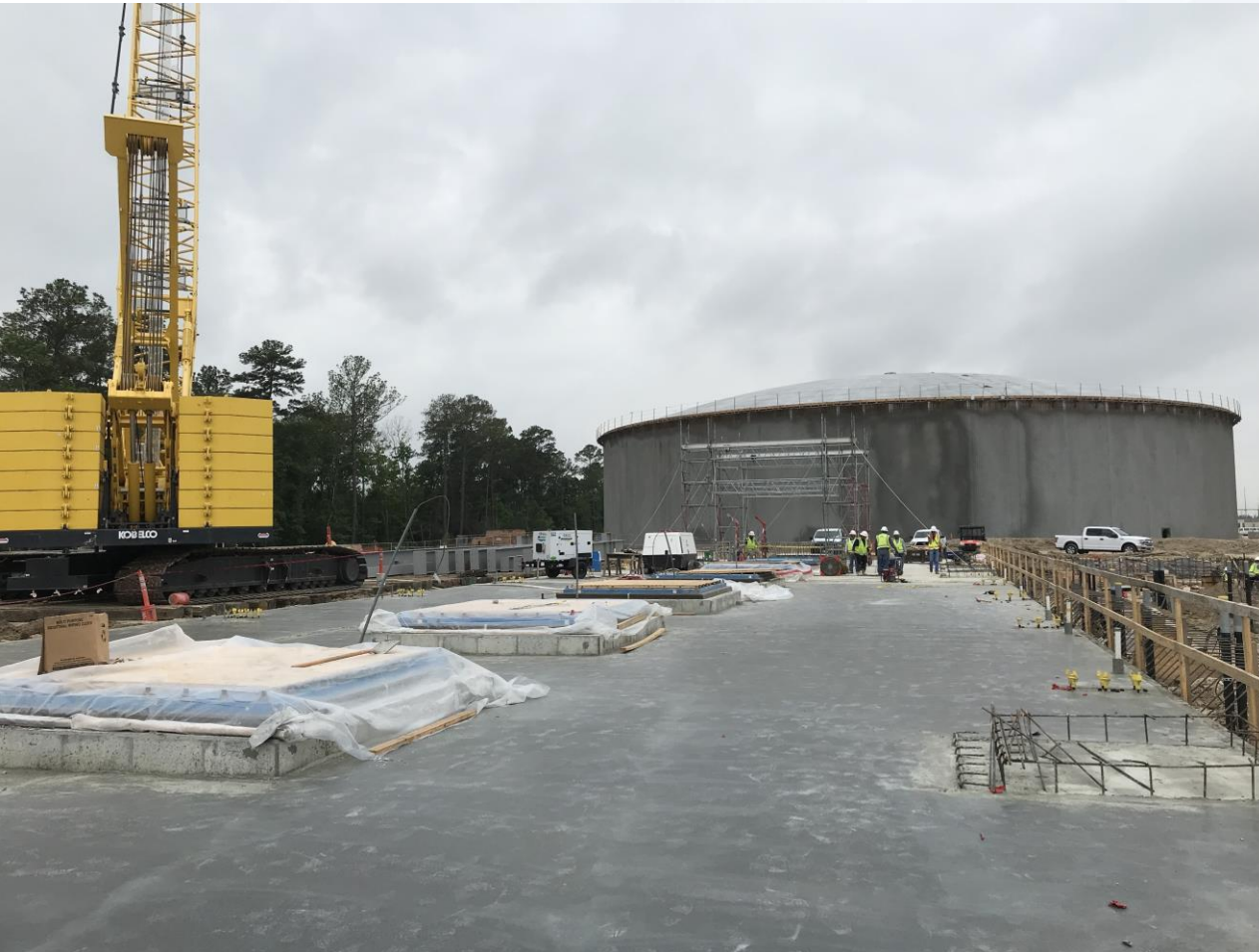
Completed concrete slab pour at the pump room at Fac 401
