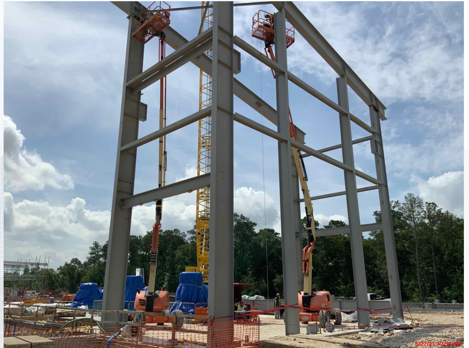
401 – Commenced steel erection
