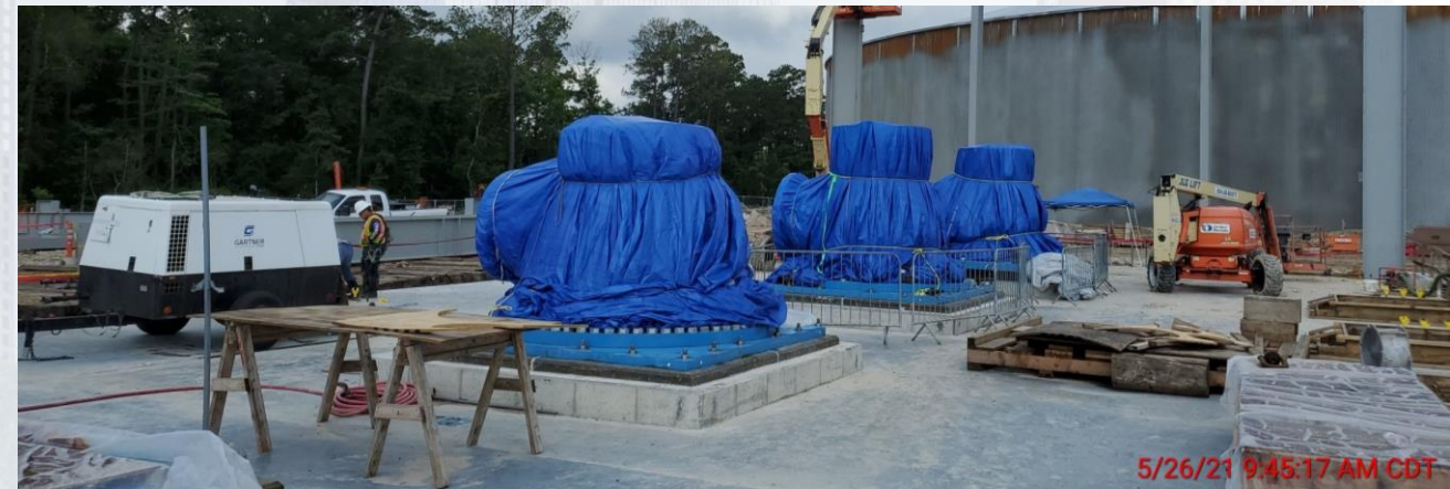
401 – Delivery and installation of 3 of the 6 vertical turbine pumps
