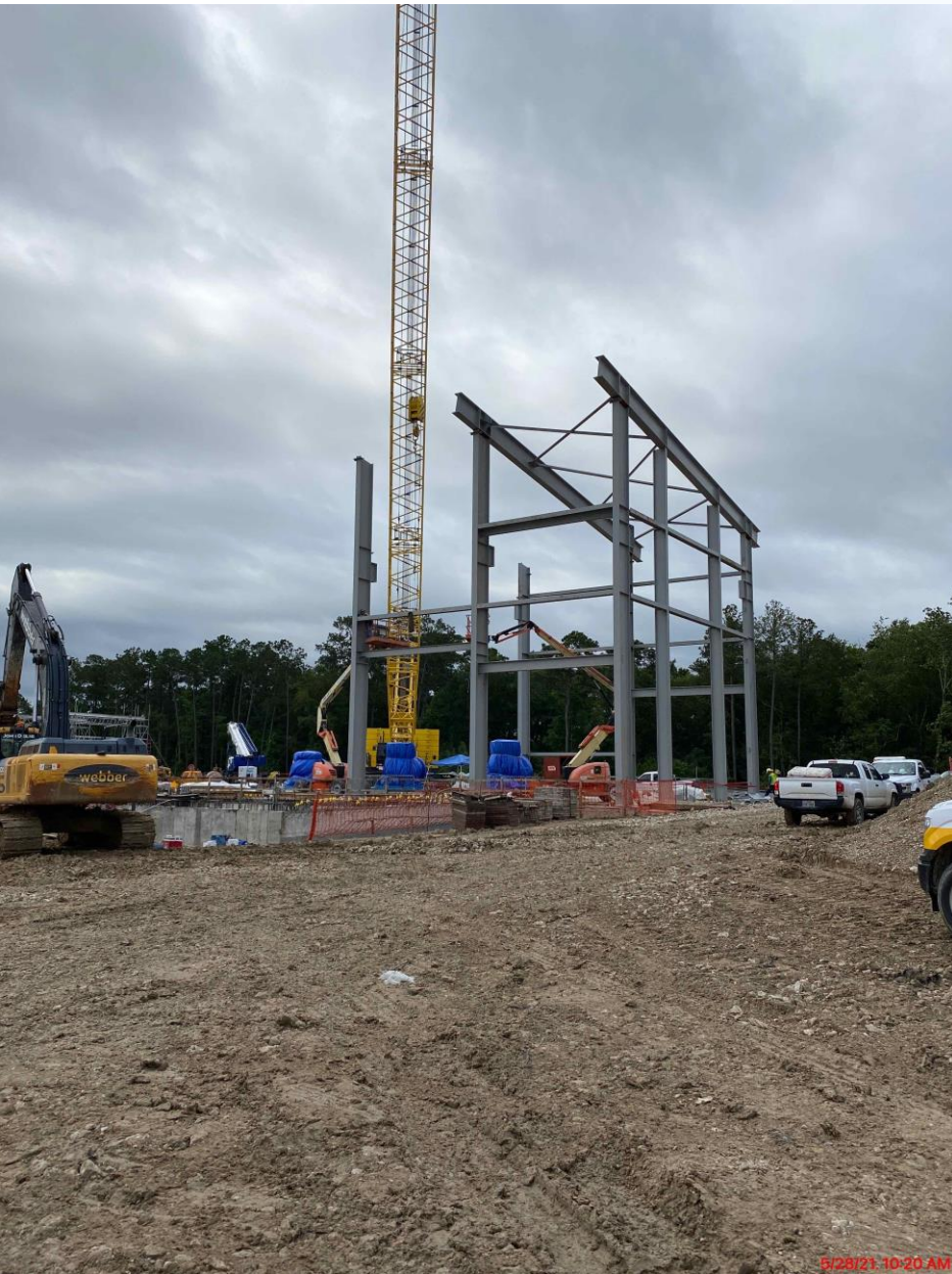
401 – Commenced steel erection
