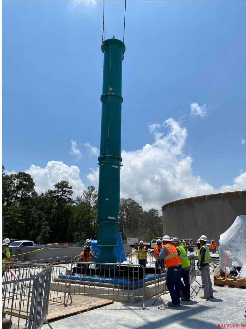
401 – Delivery and installation of 3 of the 6 vertical turbine pumps
