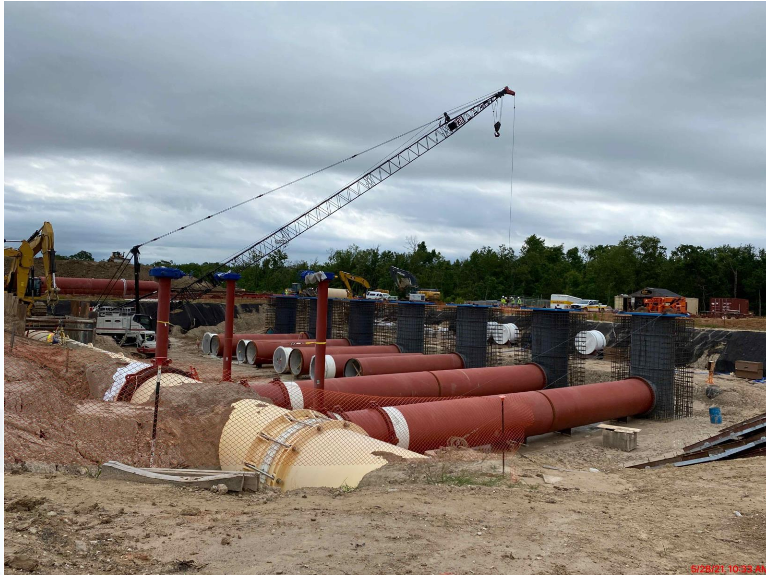
402 – Continued installation of 78" buried pipe
