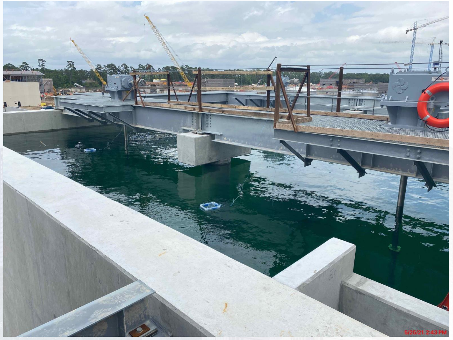
510 – Commenced water tightness testing of basins & slide gates
