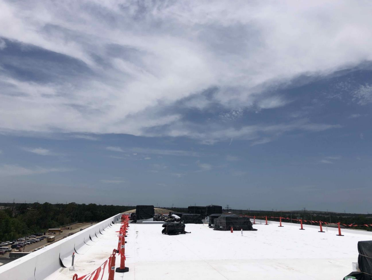
520 - Commenced TPO roofing upper level
