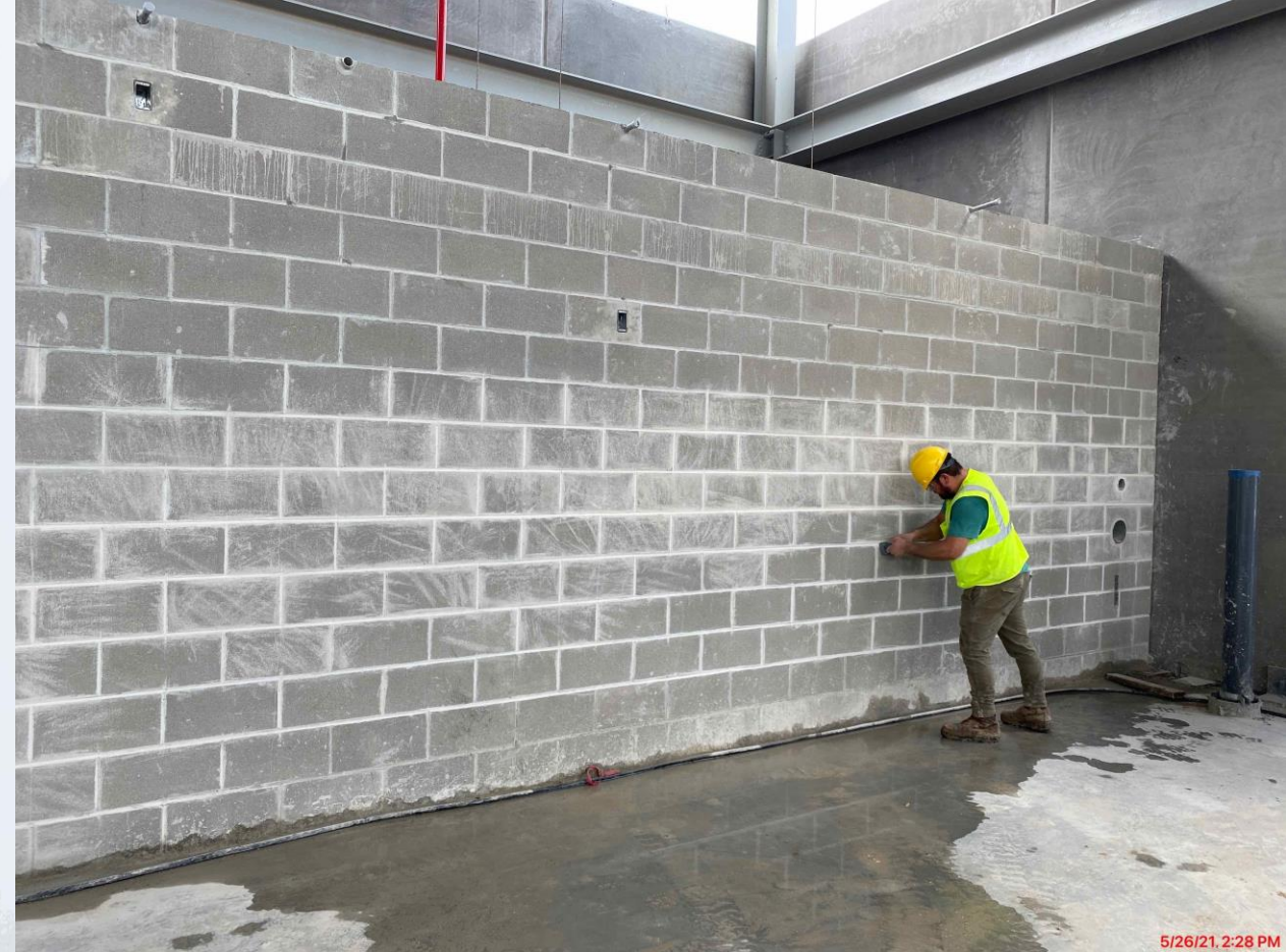
520 - Cleaning CMU at the electrical, mechanical, and other rooms
