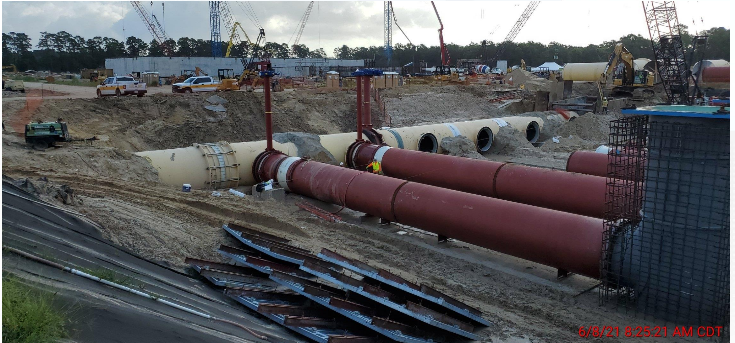
402 – Continued installation of 78" buried pipe
