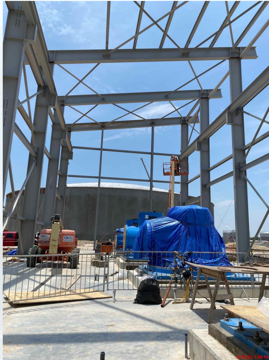
401 – Continued steel erection
