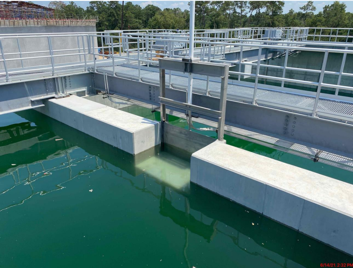
510 – Continued water tightness testing of basins & slide gates
