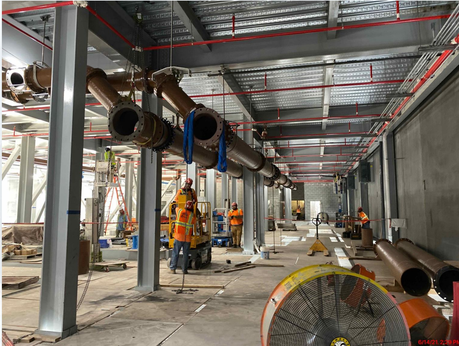
520 – Continued process pipe installation
