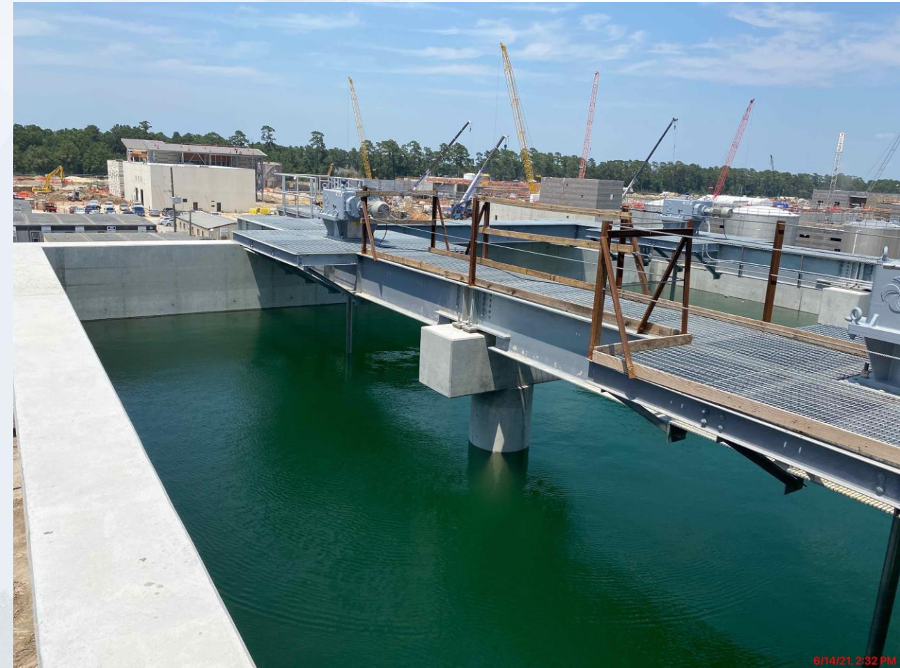
510 – Continued water tightness testing of basins & slide gates
