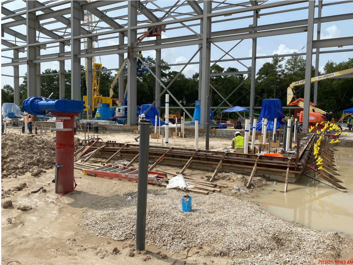
401 – Below slab plumbing and backfilling (electrical room).
