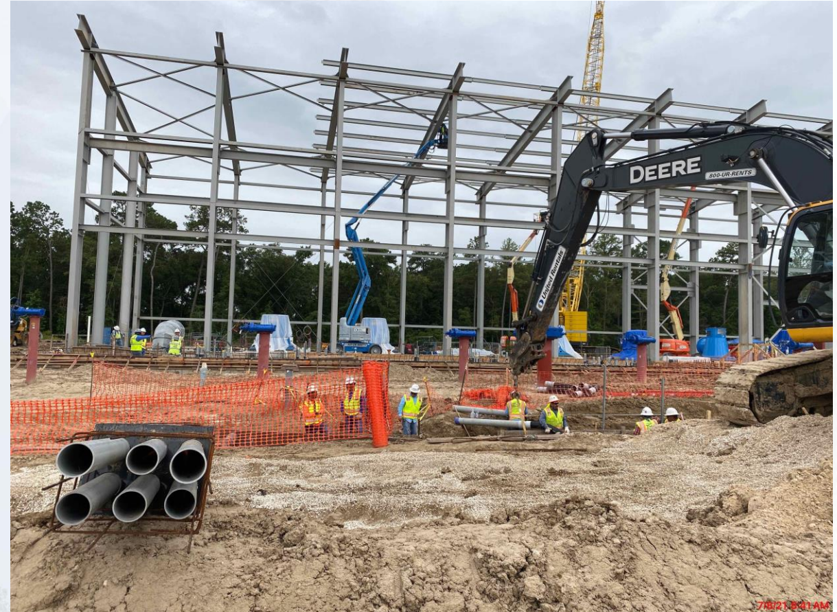
401 – Below slab plumbing and backfilling (electrical room).
