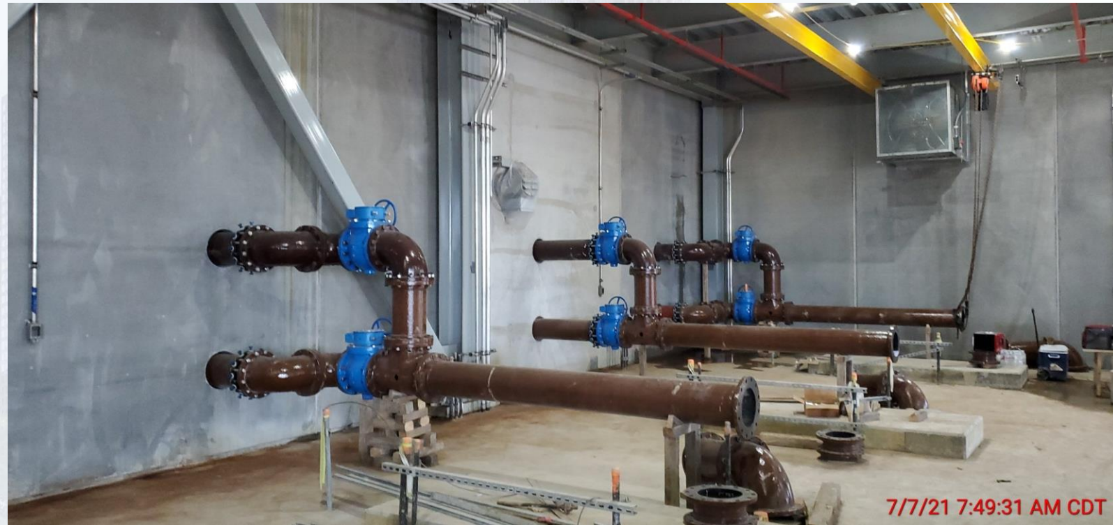
520 – Continued process pipe installation
