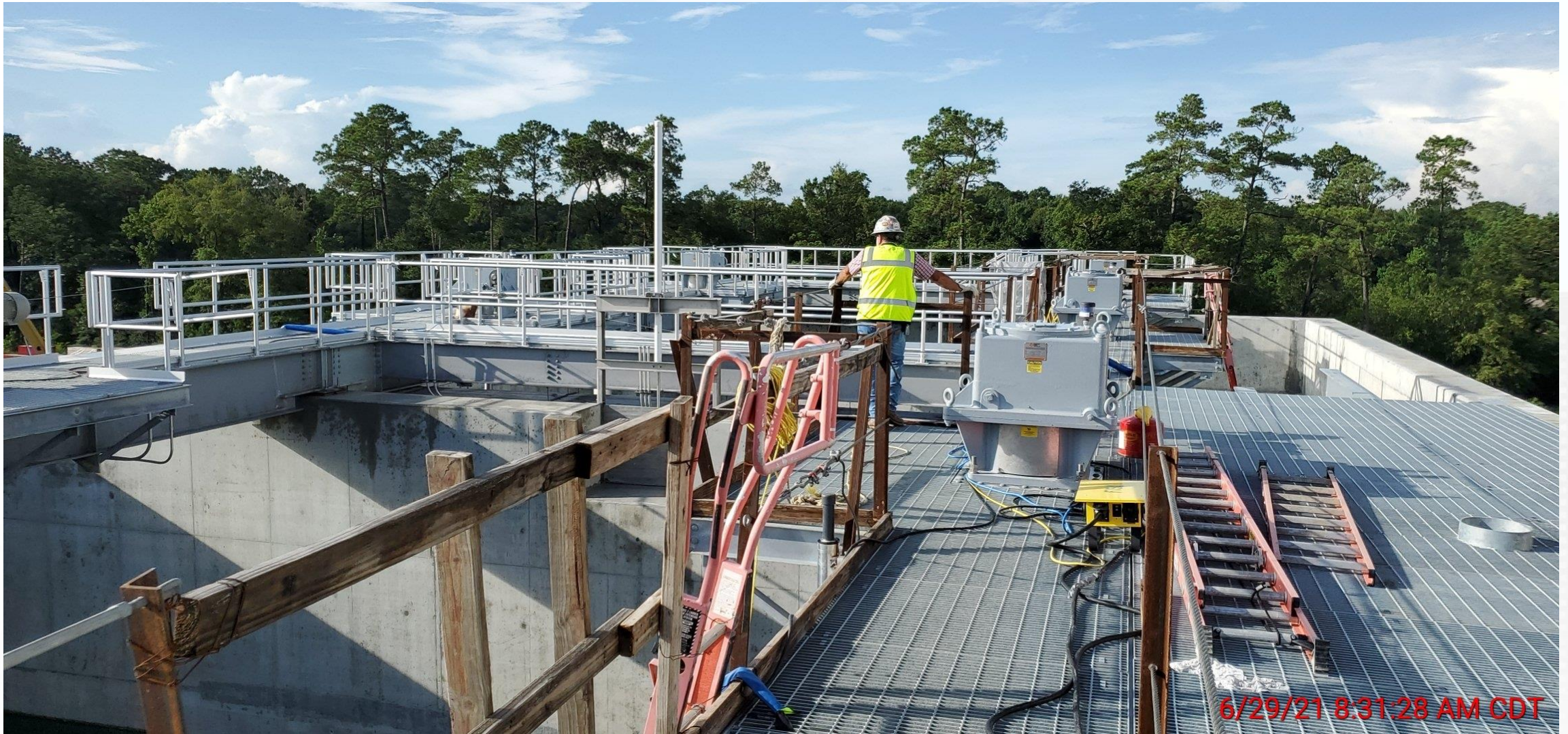
510 – Continued handrail installation.
