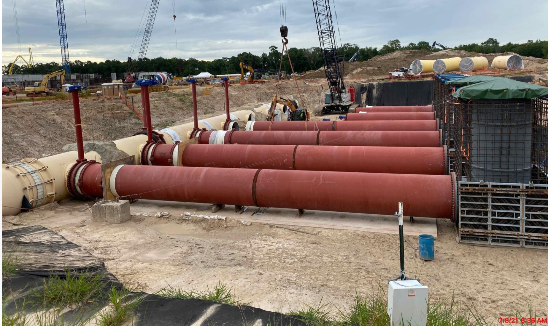
402 – Continued installation of 78" buried pipe
