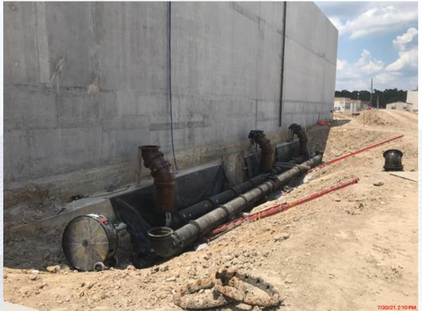
510 – Continued process pipe installation
