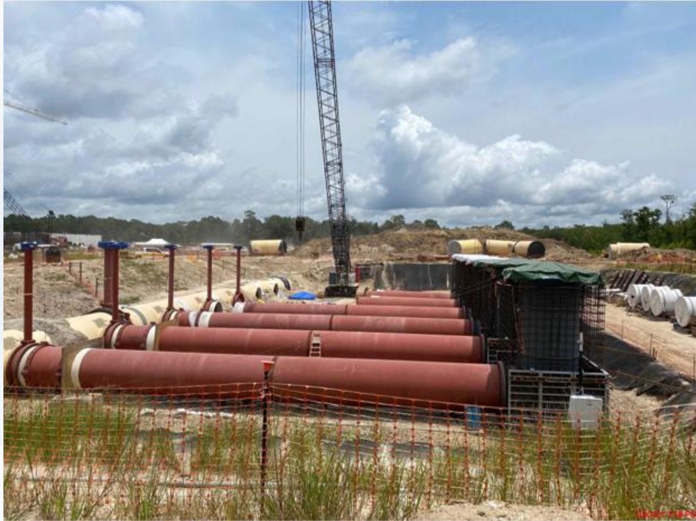
402 – Continued installation of 78" buried pipe
