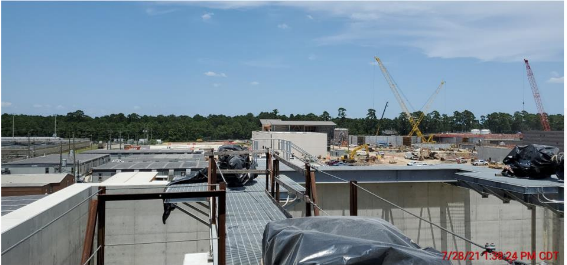
510 – Continued handrail installation.
