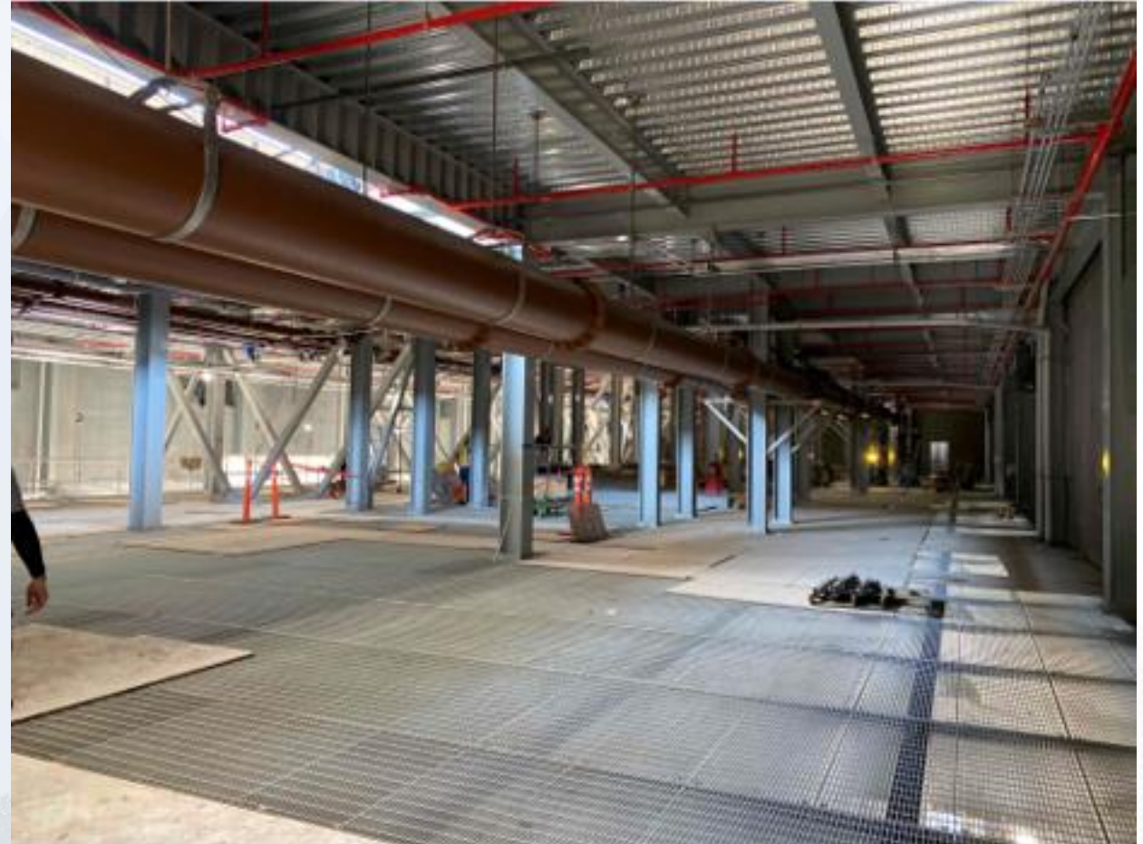
520 – Continued process pipe installation
