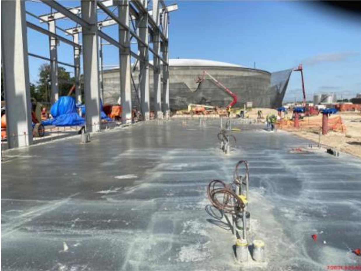
401 – Poured concrete slab at the electrical room and transformer pad
