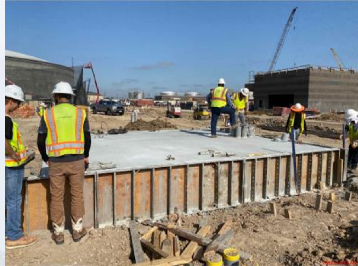
401 – Poured concrete slab at the electrical room and transformer pad
