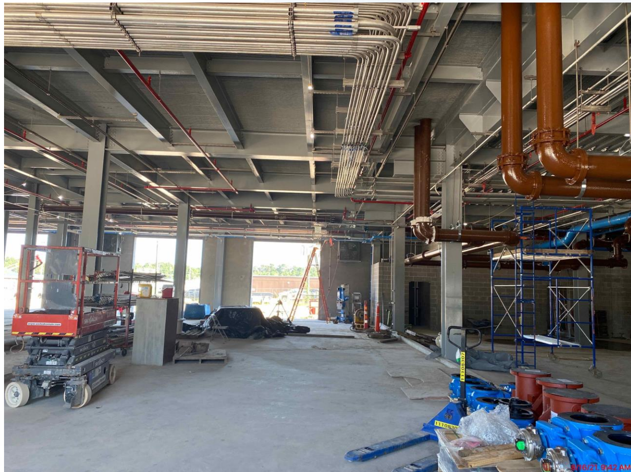
520 - Continued electrical support & conduit installation at the 1st & 2nd floor
