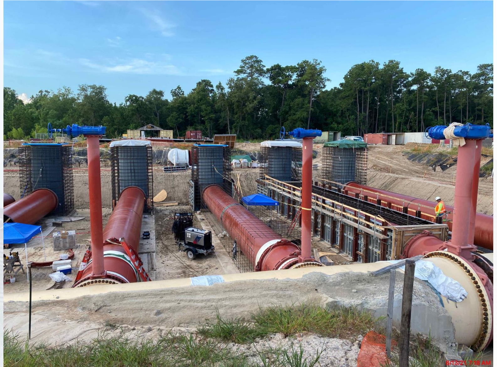
402 – Continued installation of 78” buried pipe laterals to cans & commenced pipe encasement
