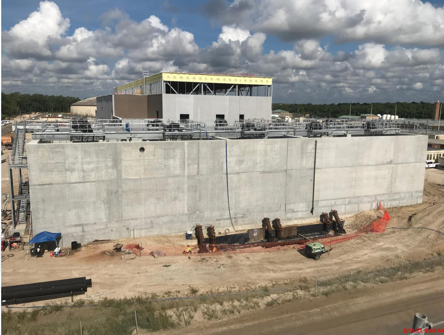
510 – Continued process pipe installation
