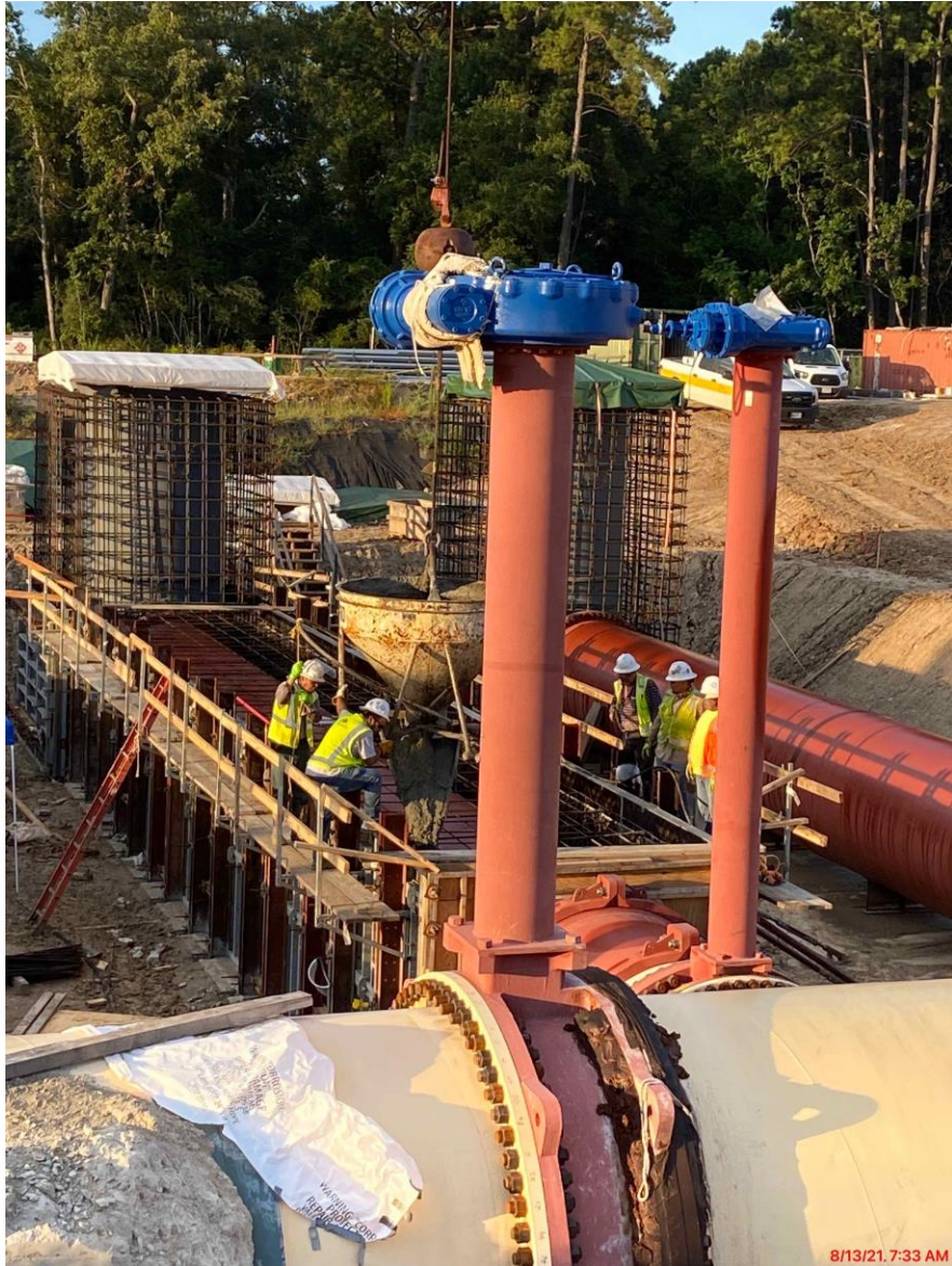
402 – Continued installation of 78” buried pipe laterals to cans & commenced pipe encasement
