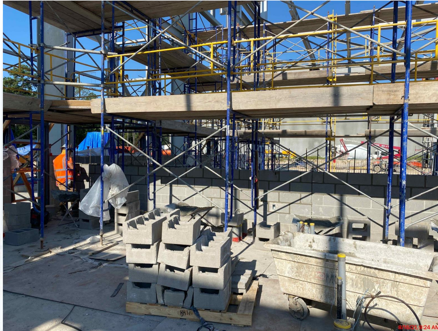
401 – Continued installation of CMU
