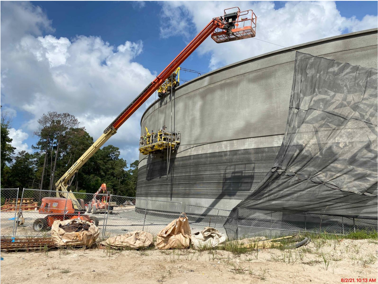
361 - Continued prestress and shotcrete
