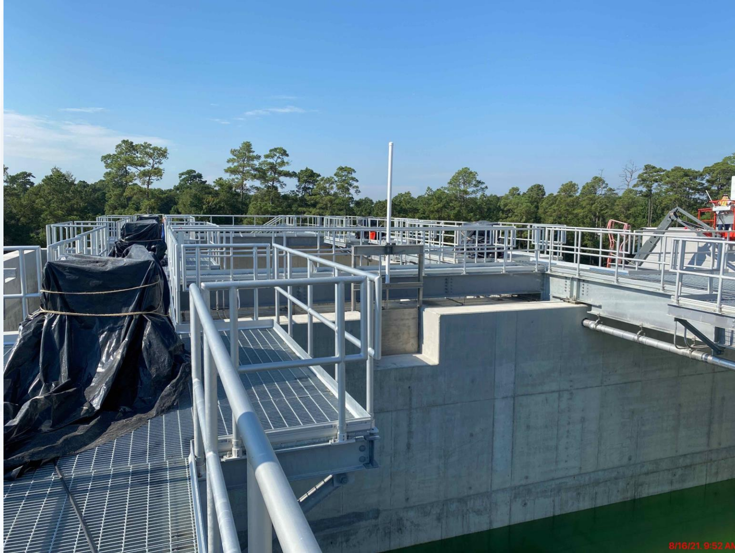
510 – Completed handrail installation
