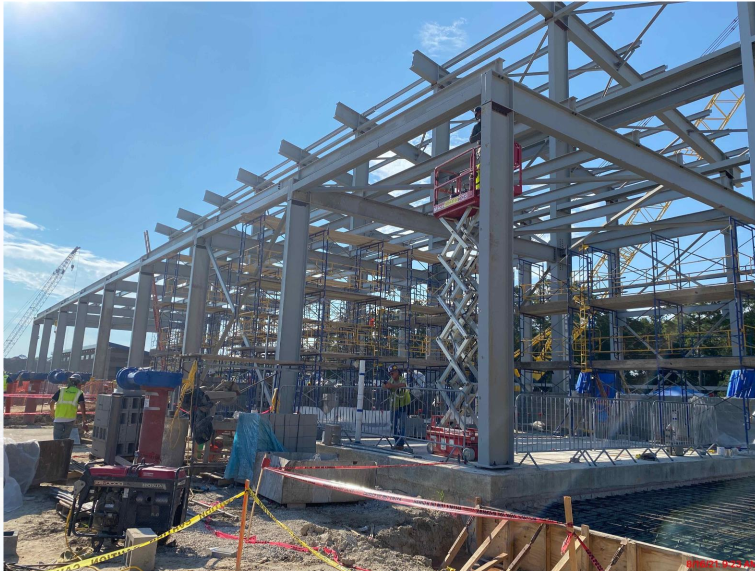
401 – Bolts & detailing of structural steel
