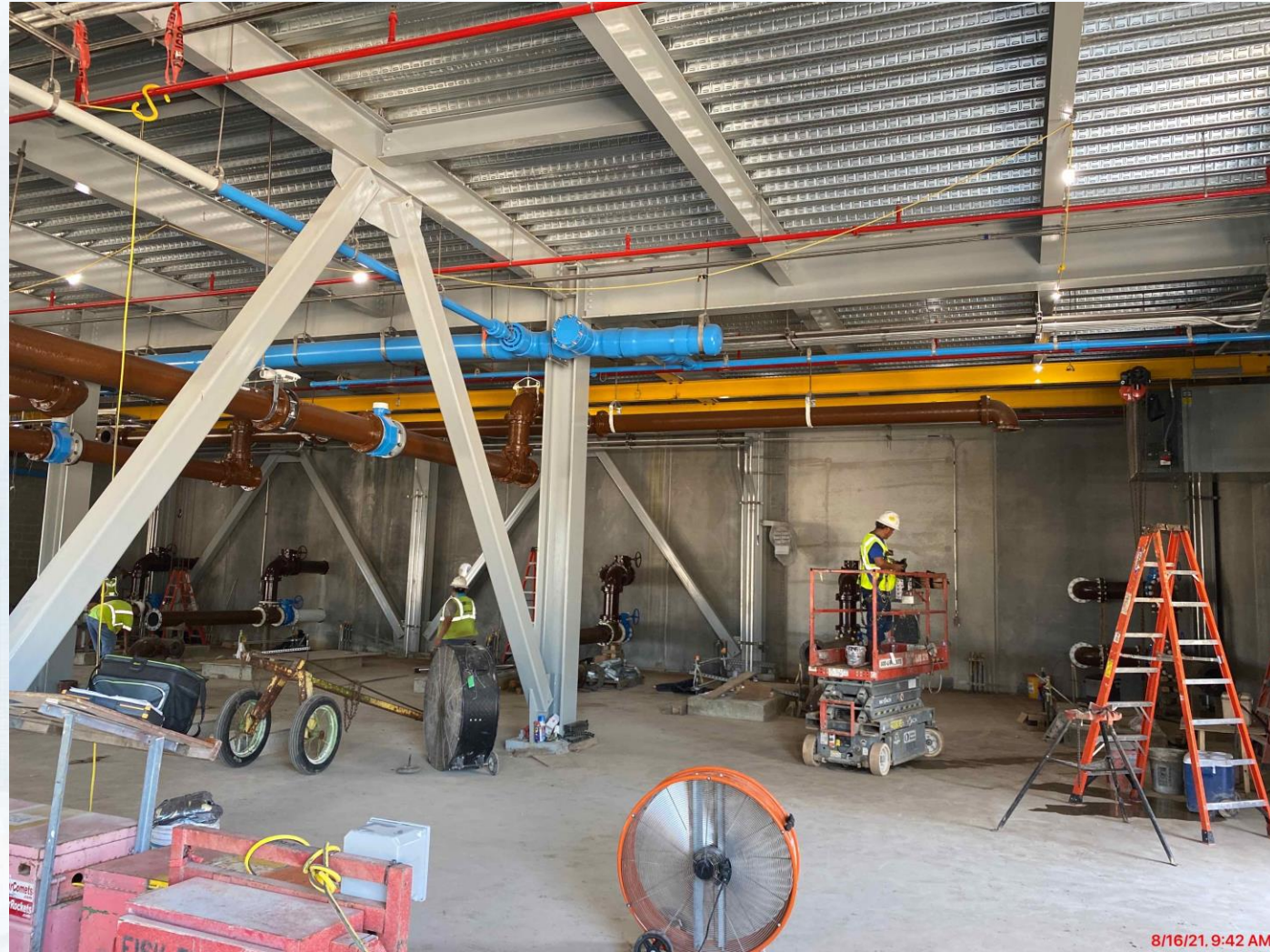
520 – Continued process pipe installation
