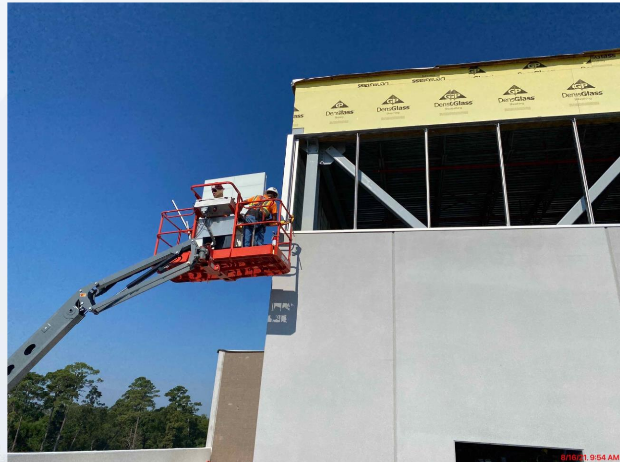
520 – Continued installation of translucent wall panels
