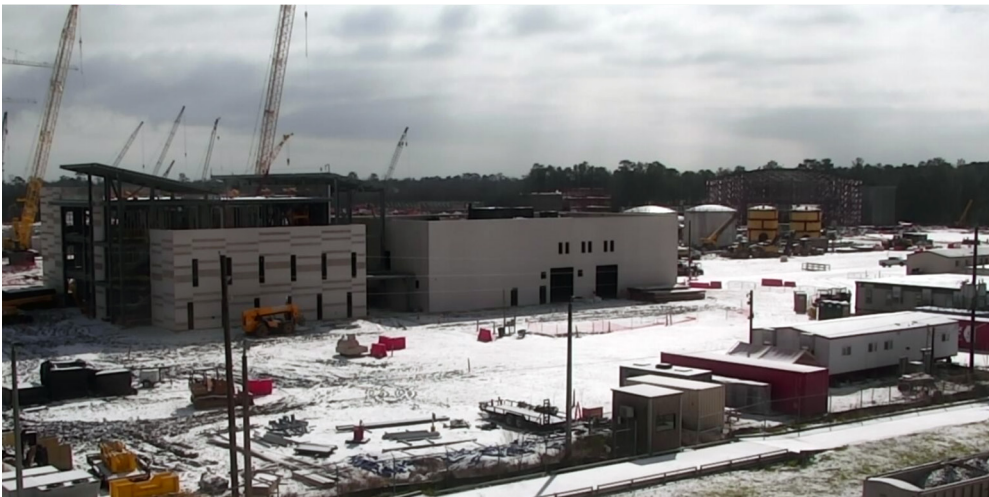
Administration and Maintenance Buildings
