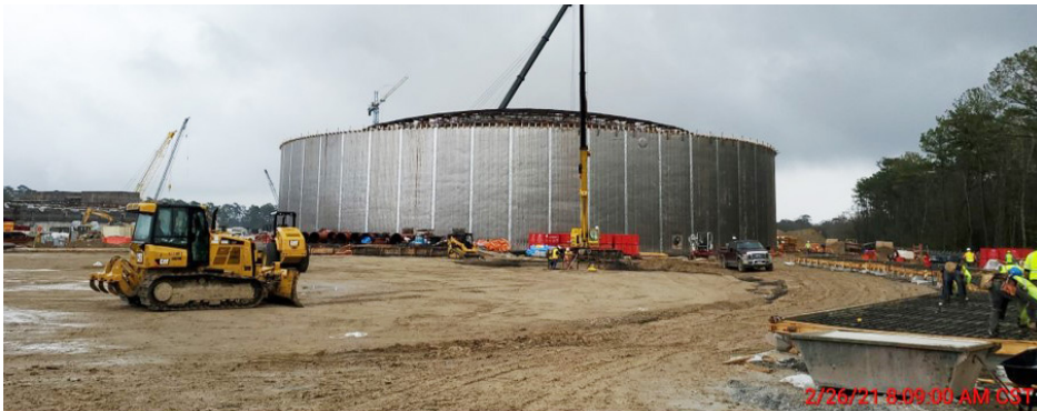
Completed Wall Panel Install - GST 362
