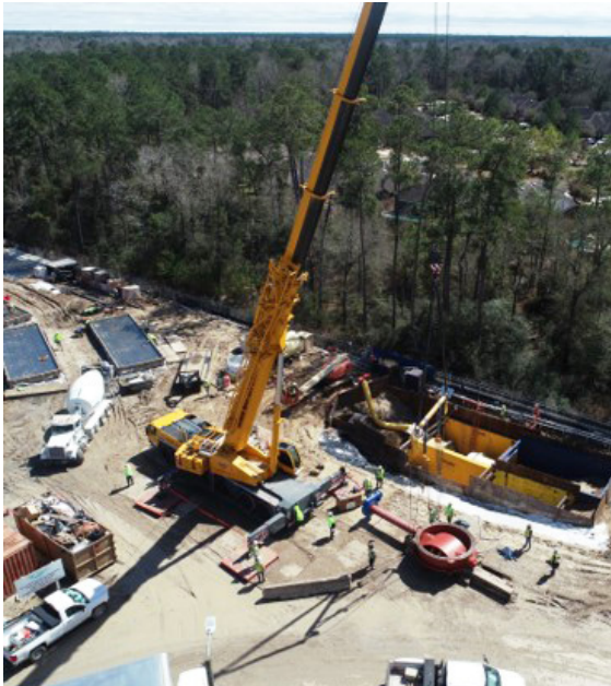
120-inch FW BFV Installation Corridor 5
