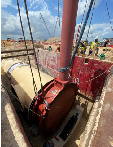
Setting the 120" BFV on FW piping Corridor 5
