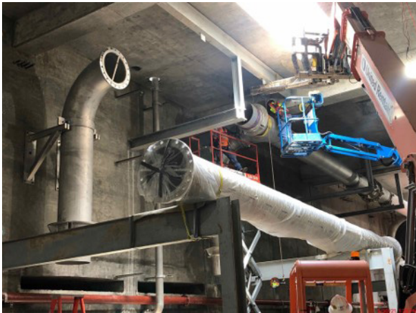
Installing Gallery Piping Facility 281
