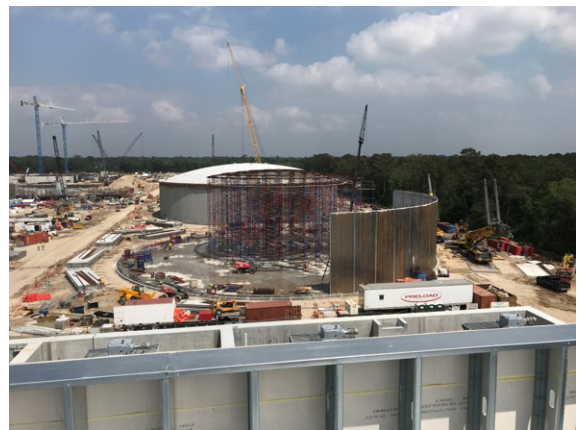
Completed Concrete Dome GST 362
