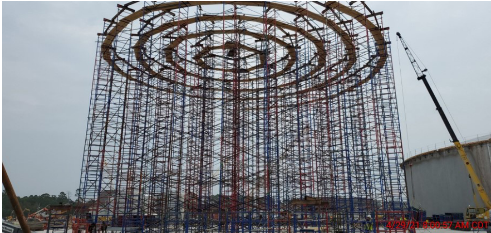
Shoring Install GST 361
