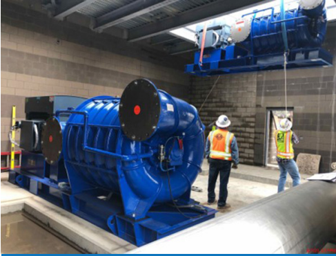
Setting the Air Scour Blowers Facility 281-Filter Module
