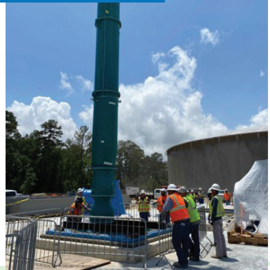
Install VT Pump Facility 401 HSPS
