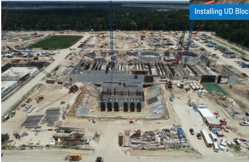
Central Plant - 2nd Phase Overall
