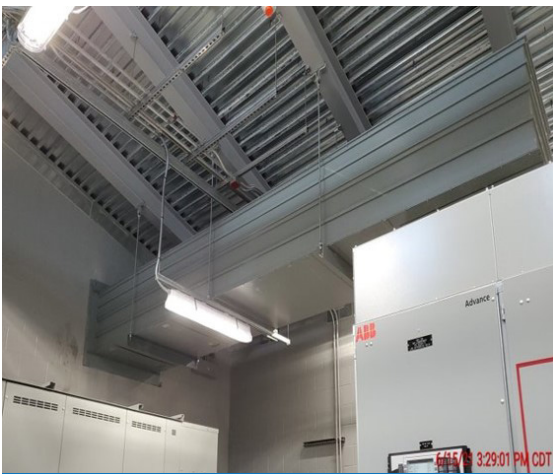
Completed Bus Duct Installation Facility 111
