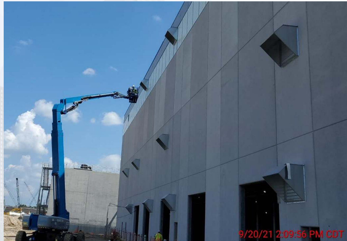
520 – Completed installation of translucent wall panels & completed installation of metal wall panels
