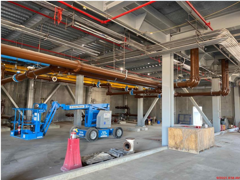
520 – Continued process pipe installation & continued electrical support & conduit installation at 1st, 2nd and 3rd floor
