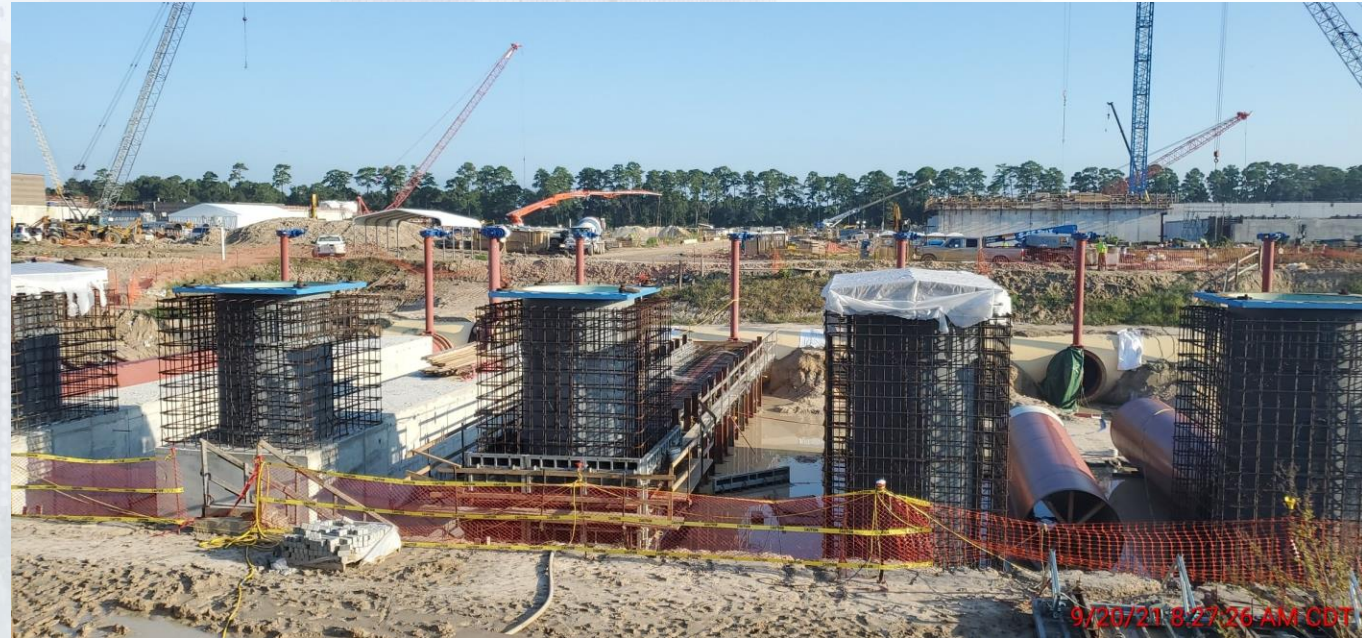
402 – Continued installation of 78” buried pipe laterals to pump cans & continued pipe encasement of 78” buried pipe laterals to pump cans
