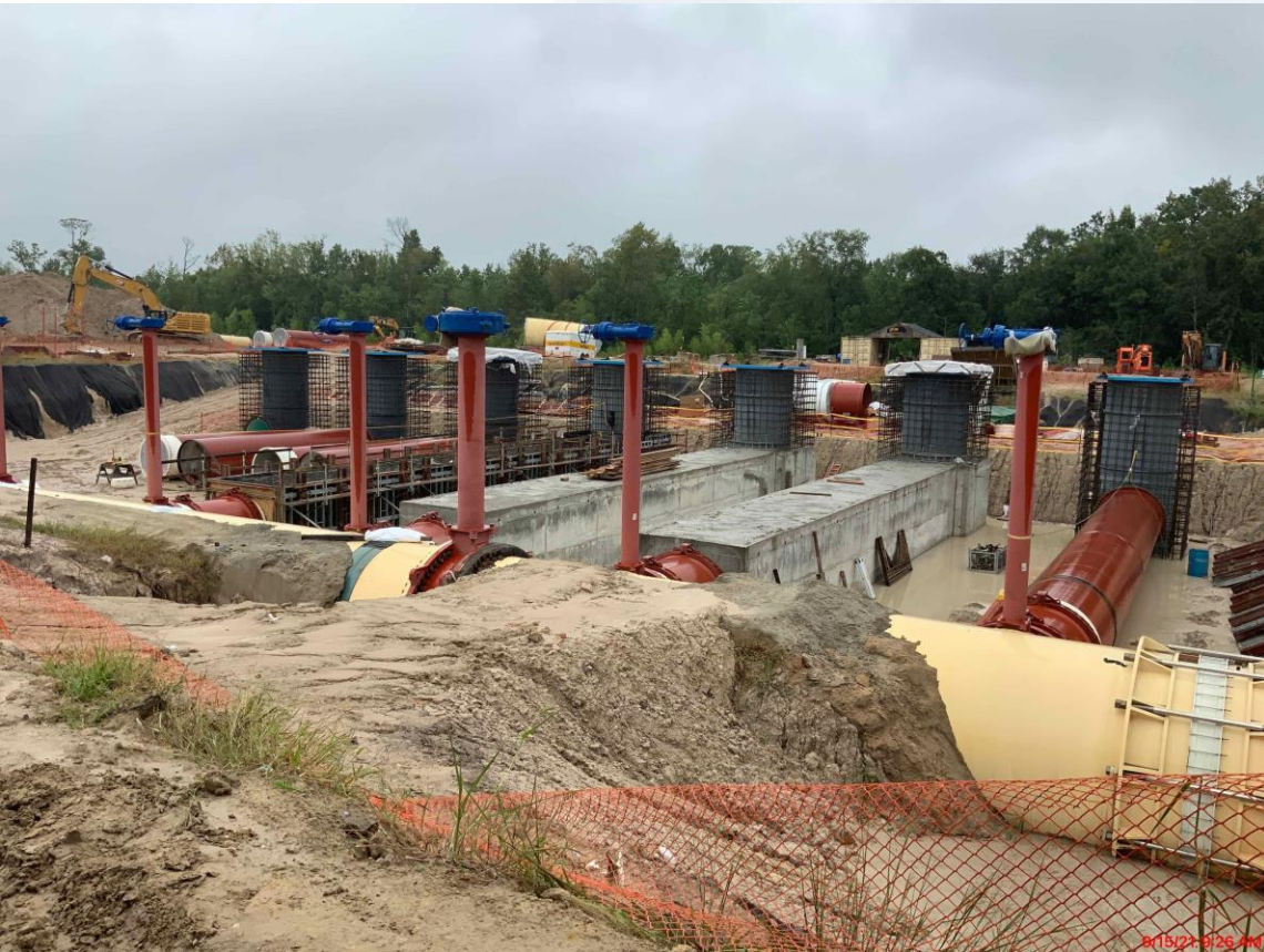
402 – Continued installation of 78” buried pipe laterals to pump cans & continued pipe encasement of 78” buried pipe laterals to pump cans
