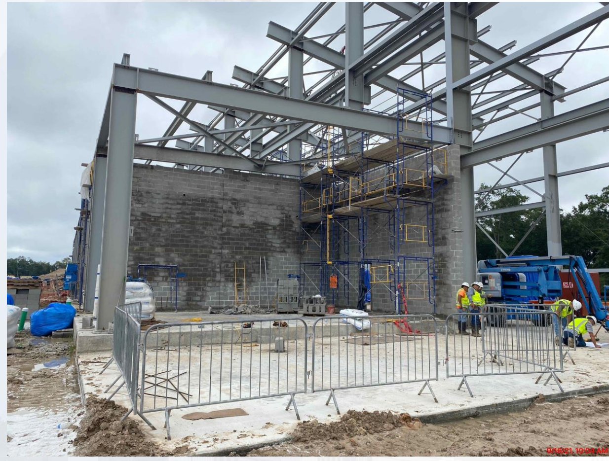
401 – Installation of CMU and detailing of structural steel
