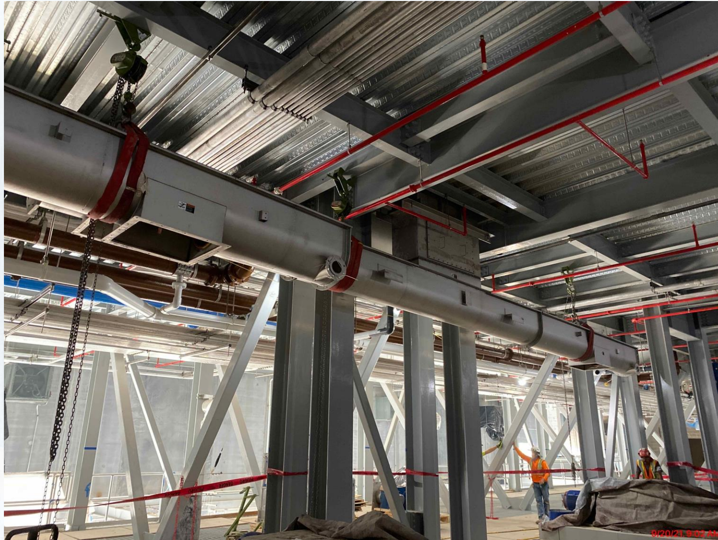
520 – Commenced conveyor installation at the 2nd floor
