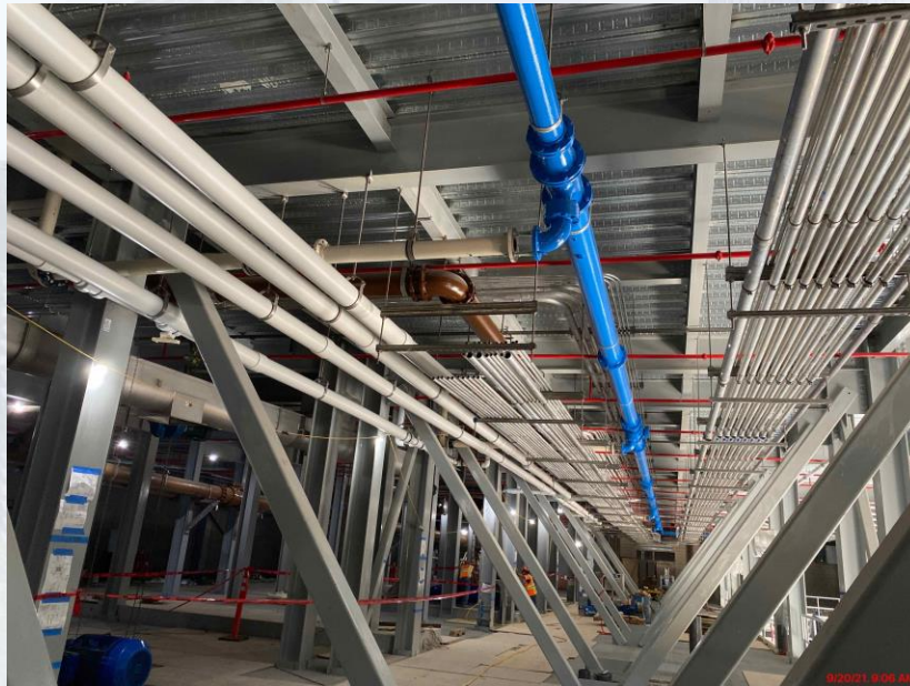
520 – Continued process pipe installation & continued electrical support & conduit installation at 1st, 2nd and 3rd floor
