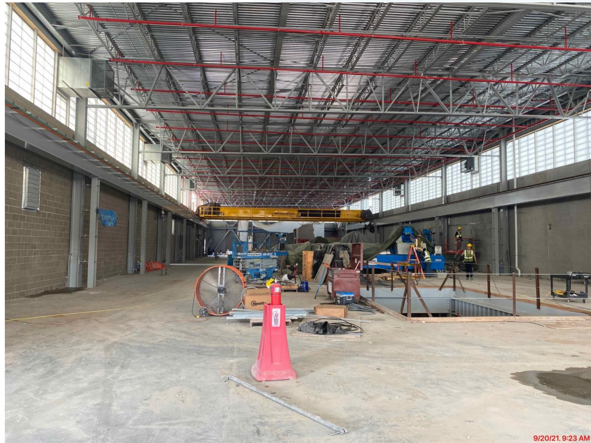
520 – Completed installation of translucent wall panels & completed installation of metal wall panels
