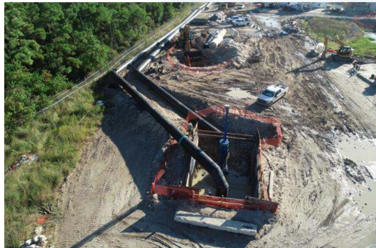
Existing 66-inch Raw Water West by-pass location
