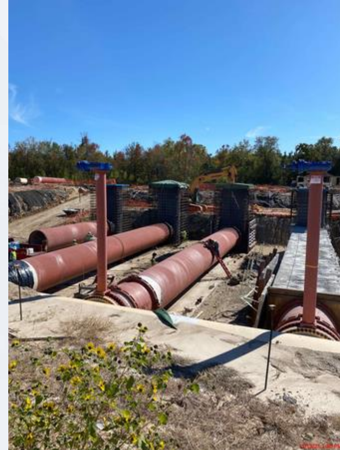
402 – Continued pipe encasement of 78” buried pipe laterals to pump cans.
