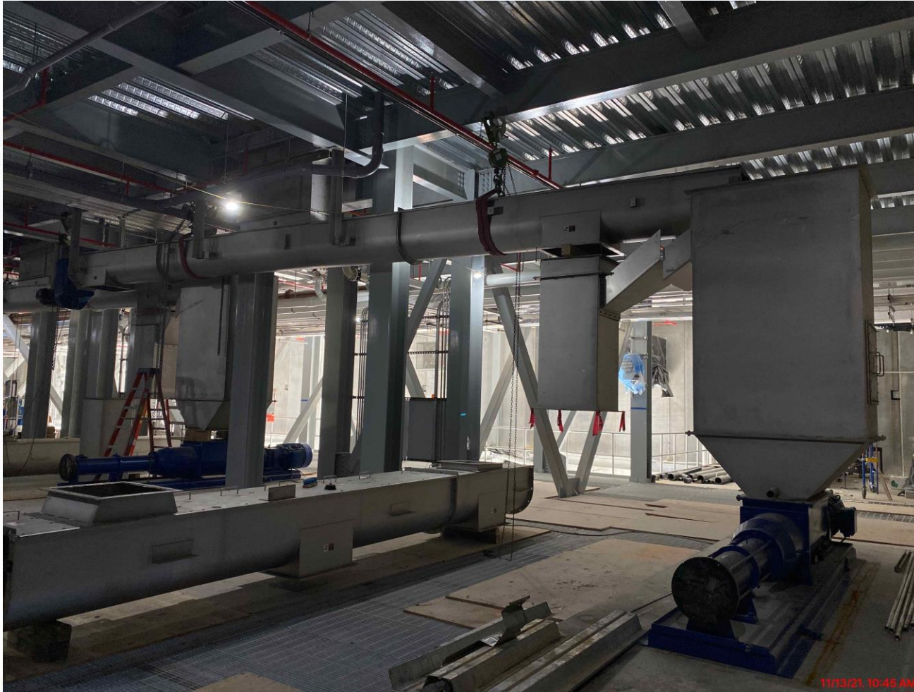
520 – Commenced conveyor installation at the 2nd floor
