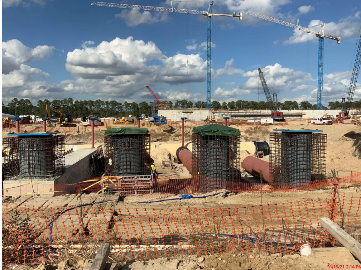
402 – Continued pipe encasement of 78” buried pipe laterals to pump cans.
