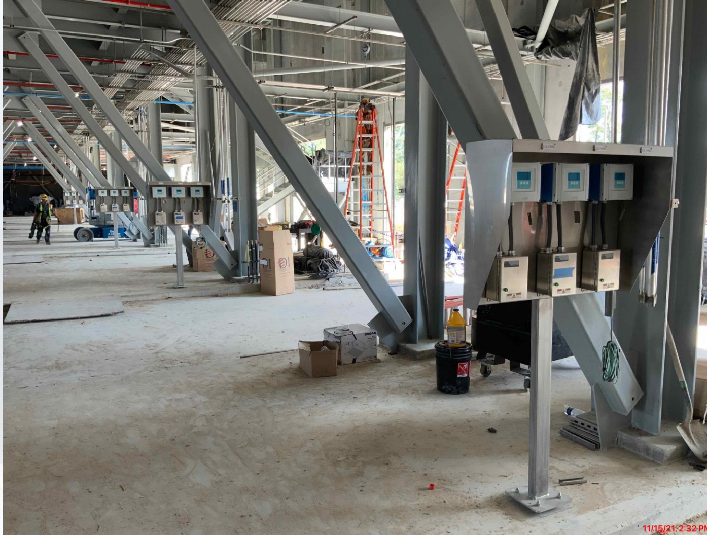
520 – Continued installation of LIT's, and other instruments.
