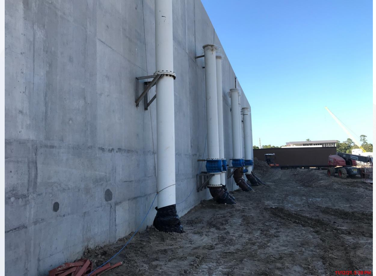
510 – Installation of LIT's and continued process pipe installation
