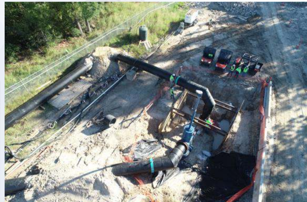
Existing 66-inch Raw Water East by-pass location
