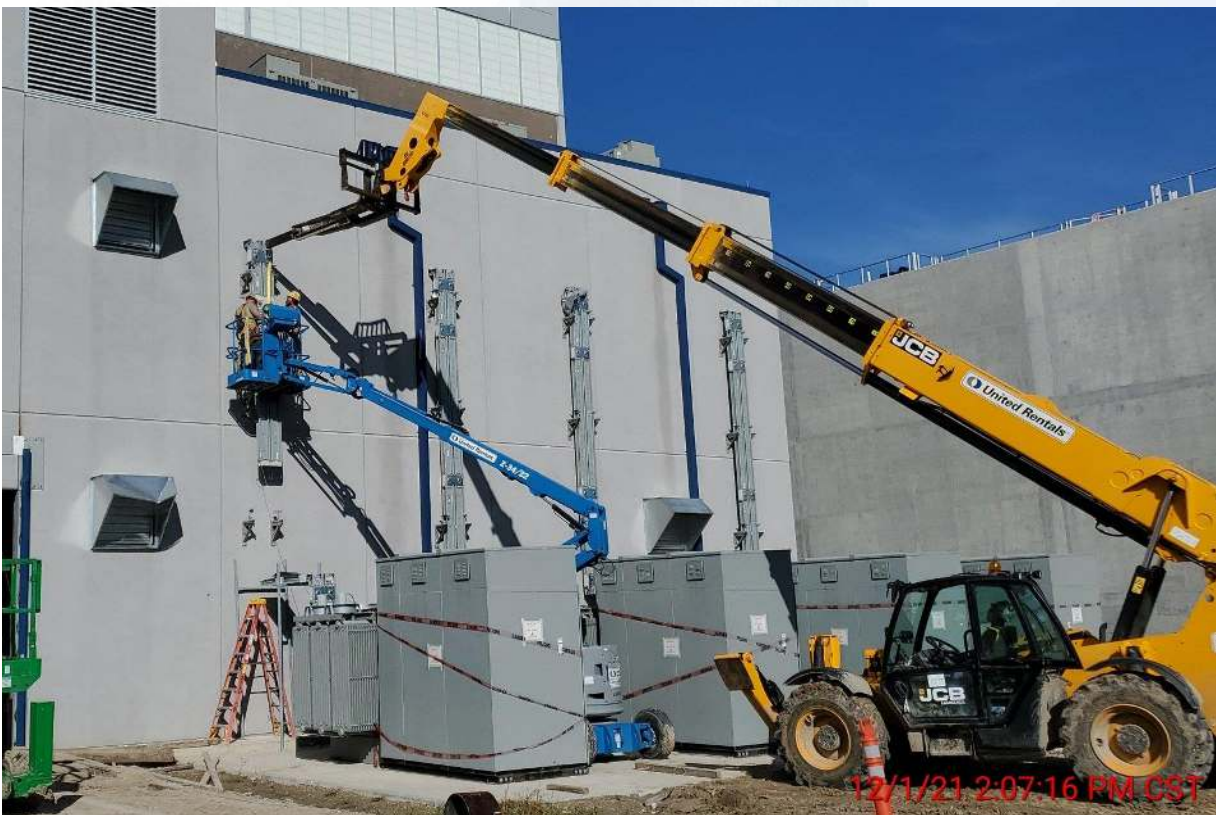
520 – Continued installation of bus duct and overhead doors
