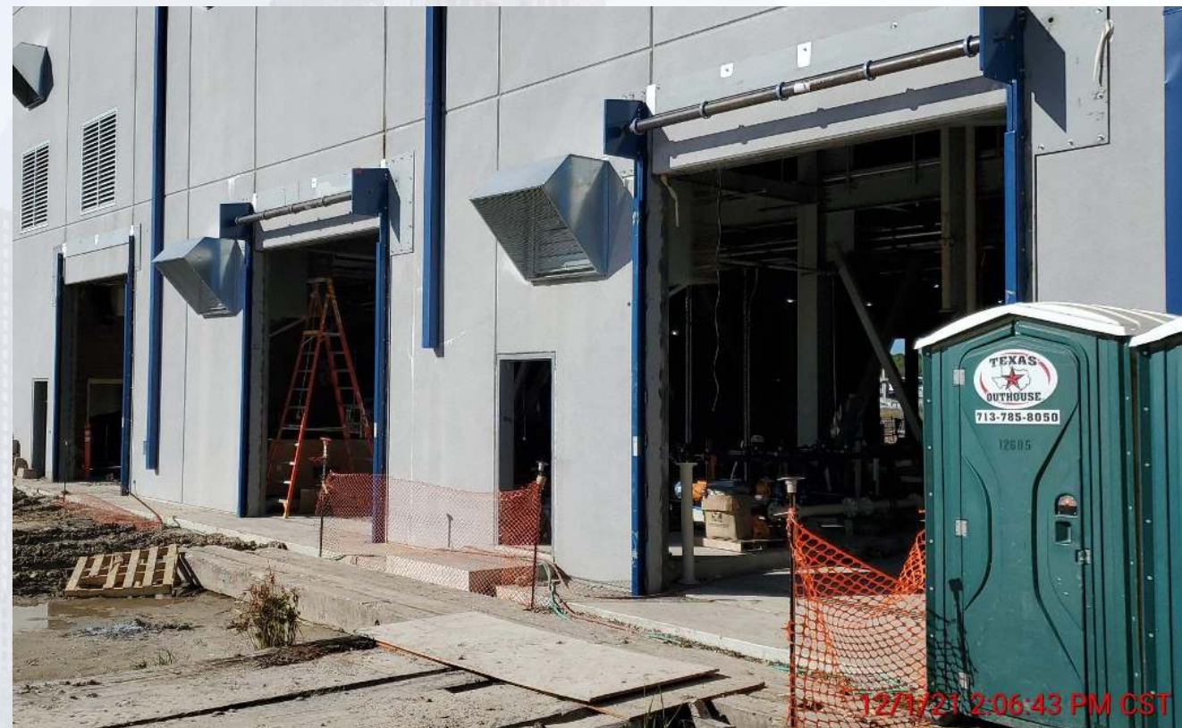
520 – Continued installation of bus duct and overhead doors
