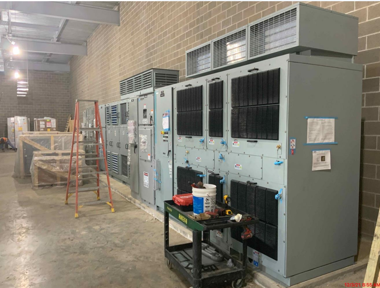
401 - Delivery of ASD's and switchgear
