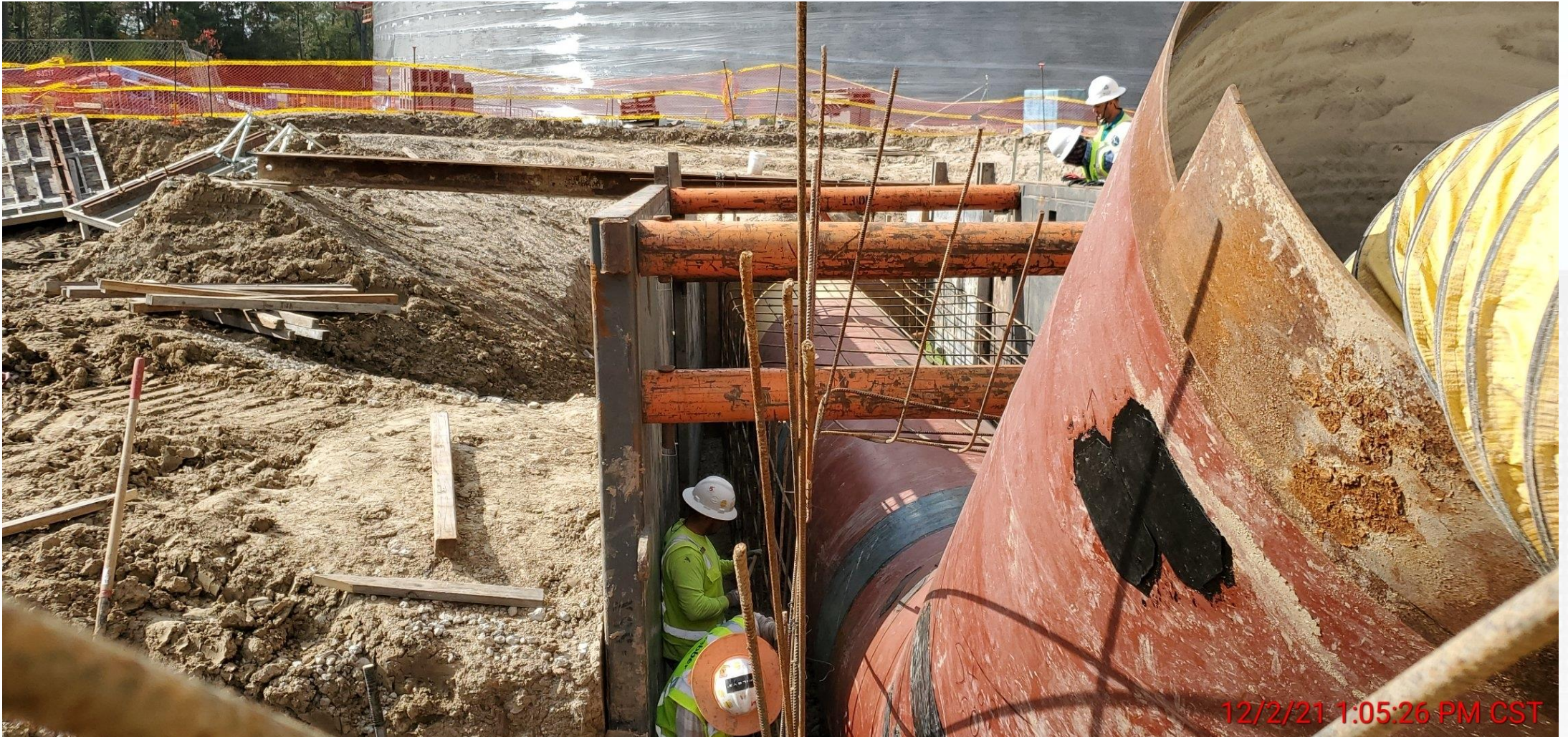
401 – Continued 60-inch BWS installation
