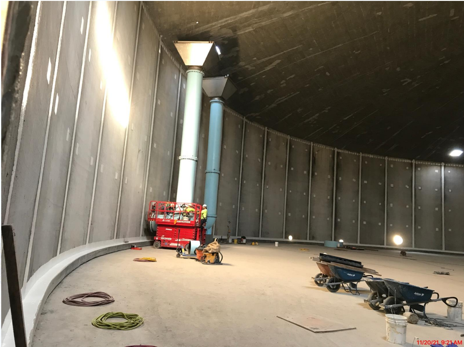
362 – Continued interior tank work
