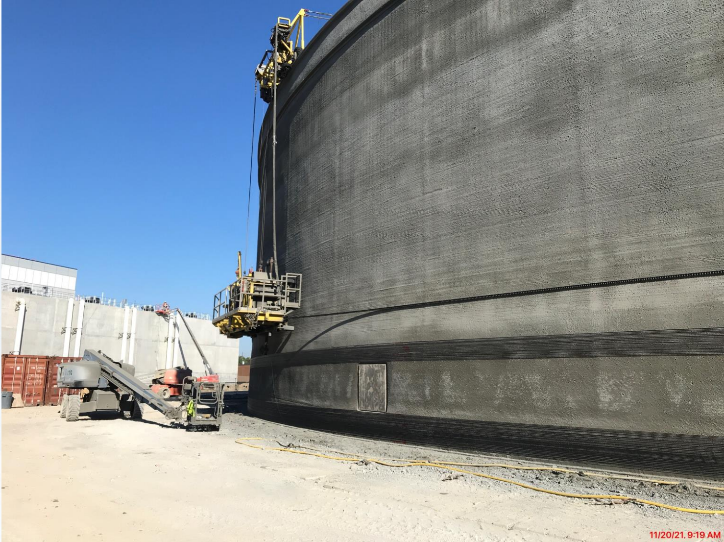
361 – Completed prestress and continued shotcrete
