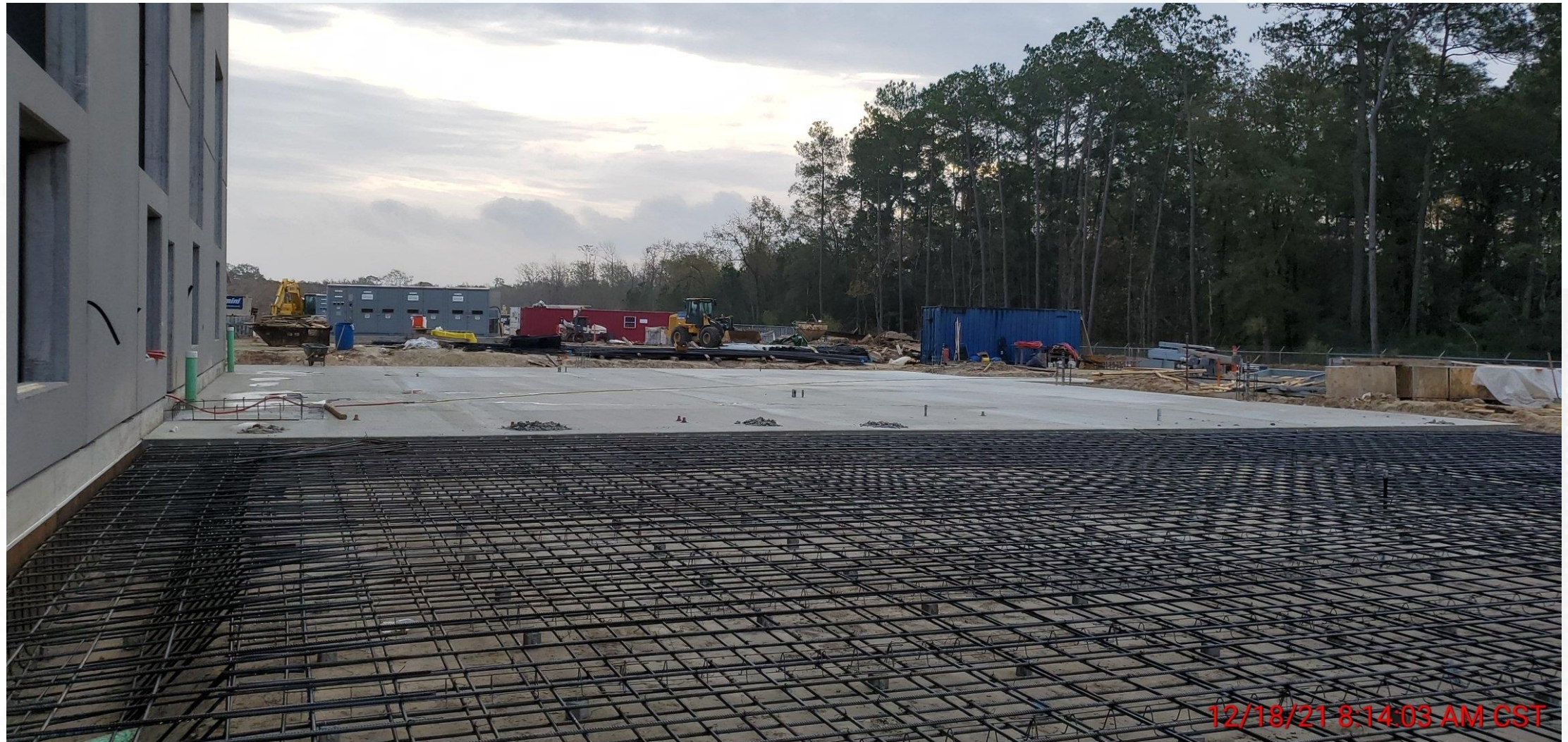
401 – Poured concrete slab
