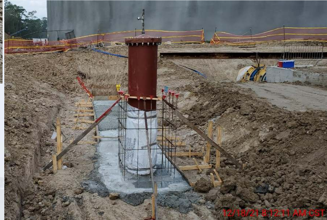
401 – Continued 60-inch BWS installation
