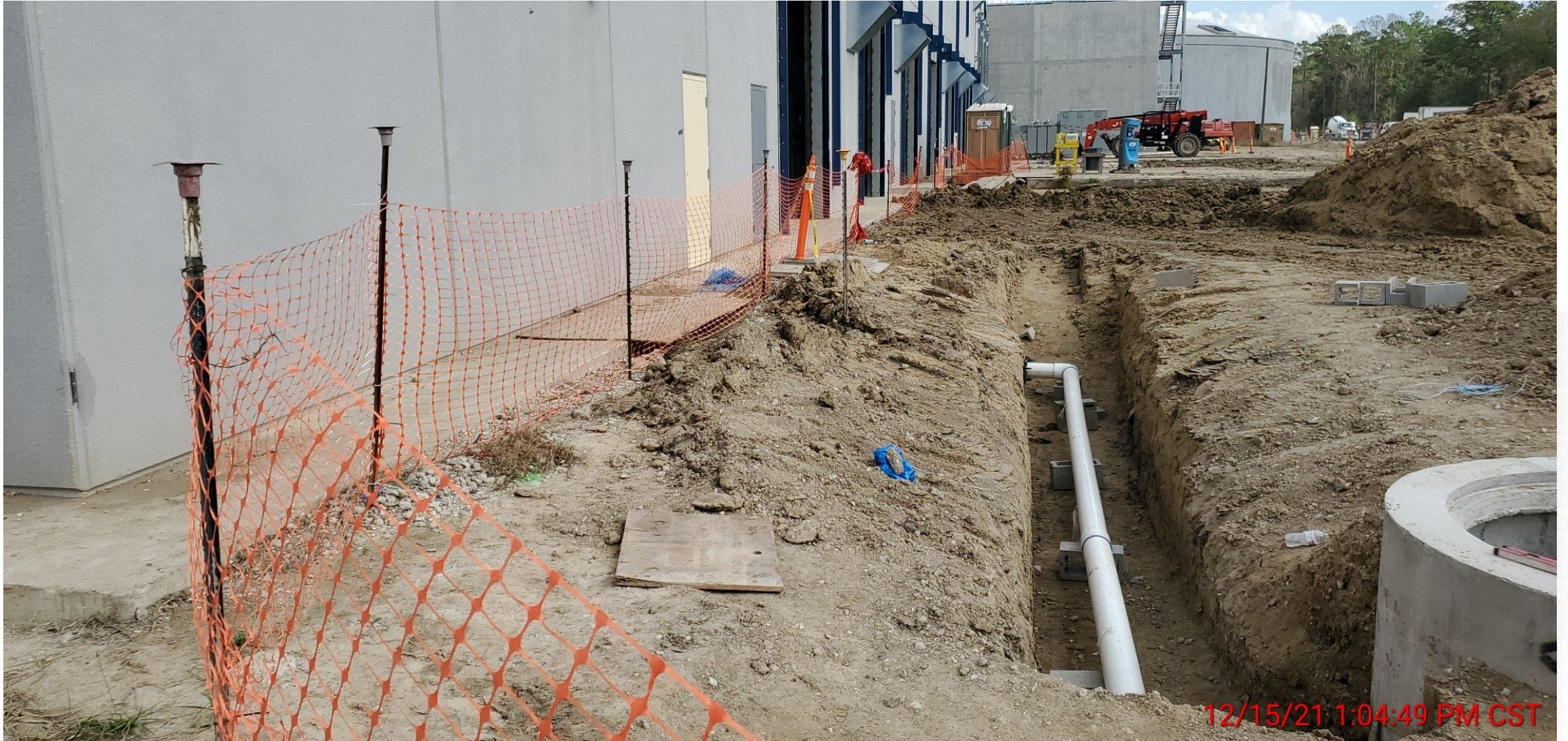
520 – Commenced installation of underground PVC
