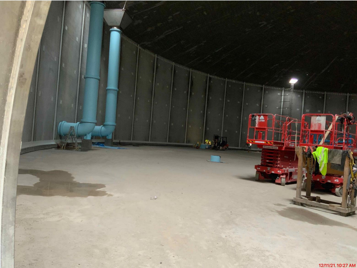
362 – Continued interior tank work
