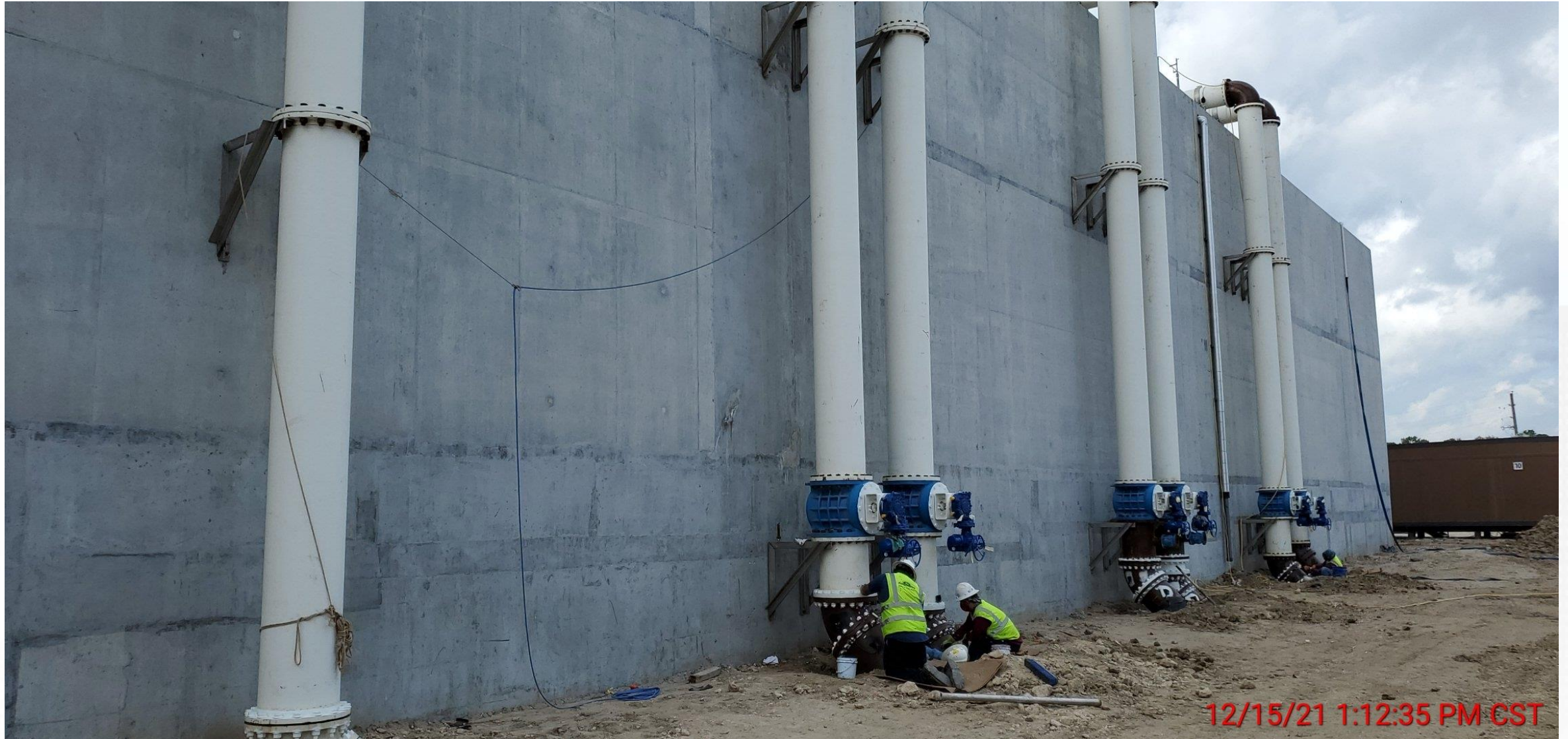
510 – Continued process pipe installation
