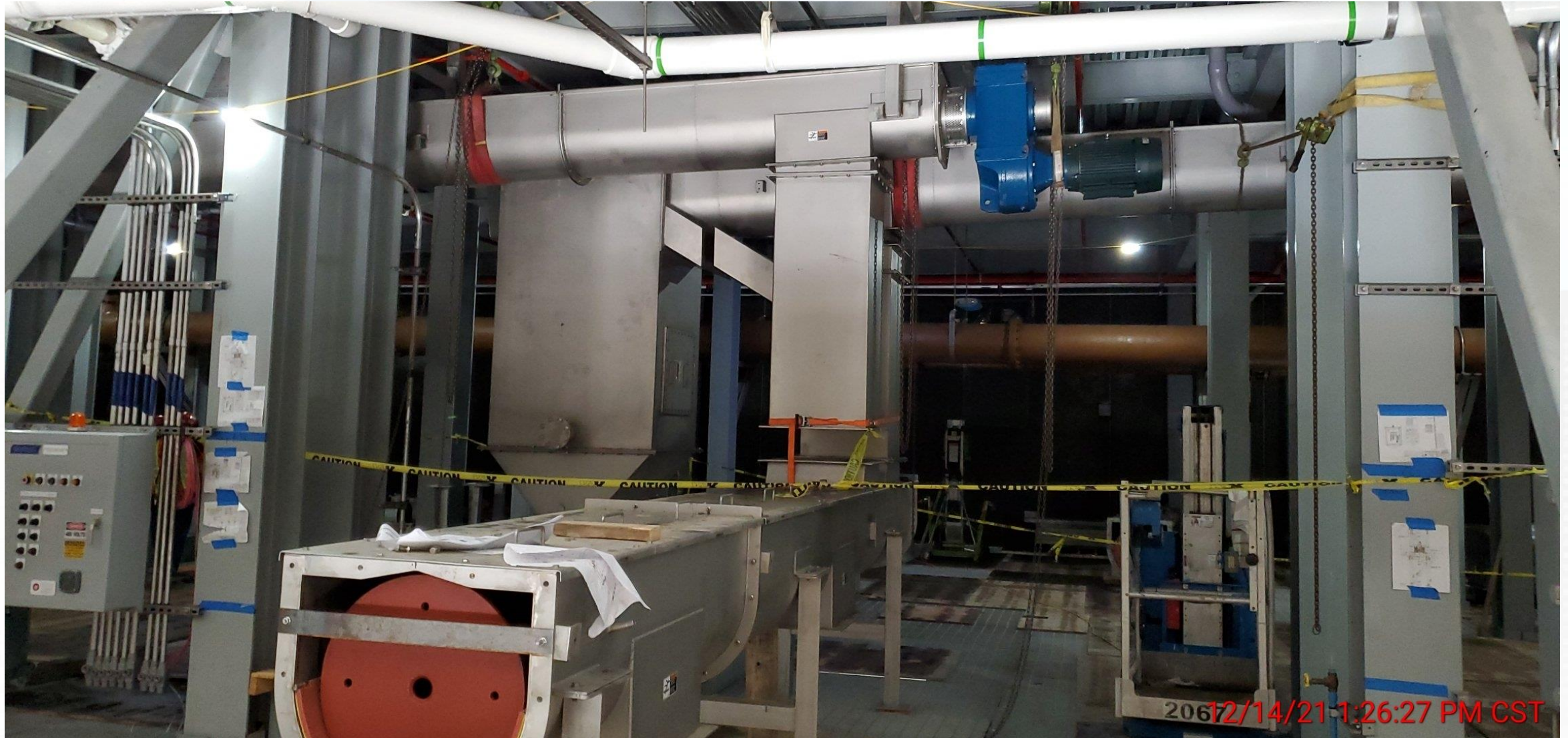
520 – Continued upper and lower conveyor installation at the 2nd floor
